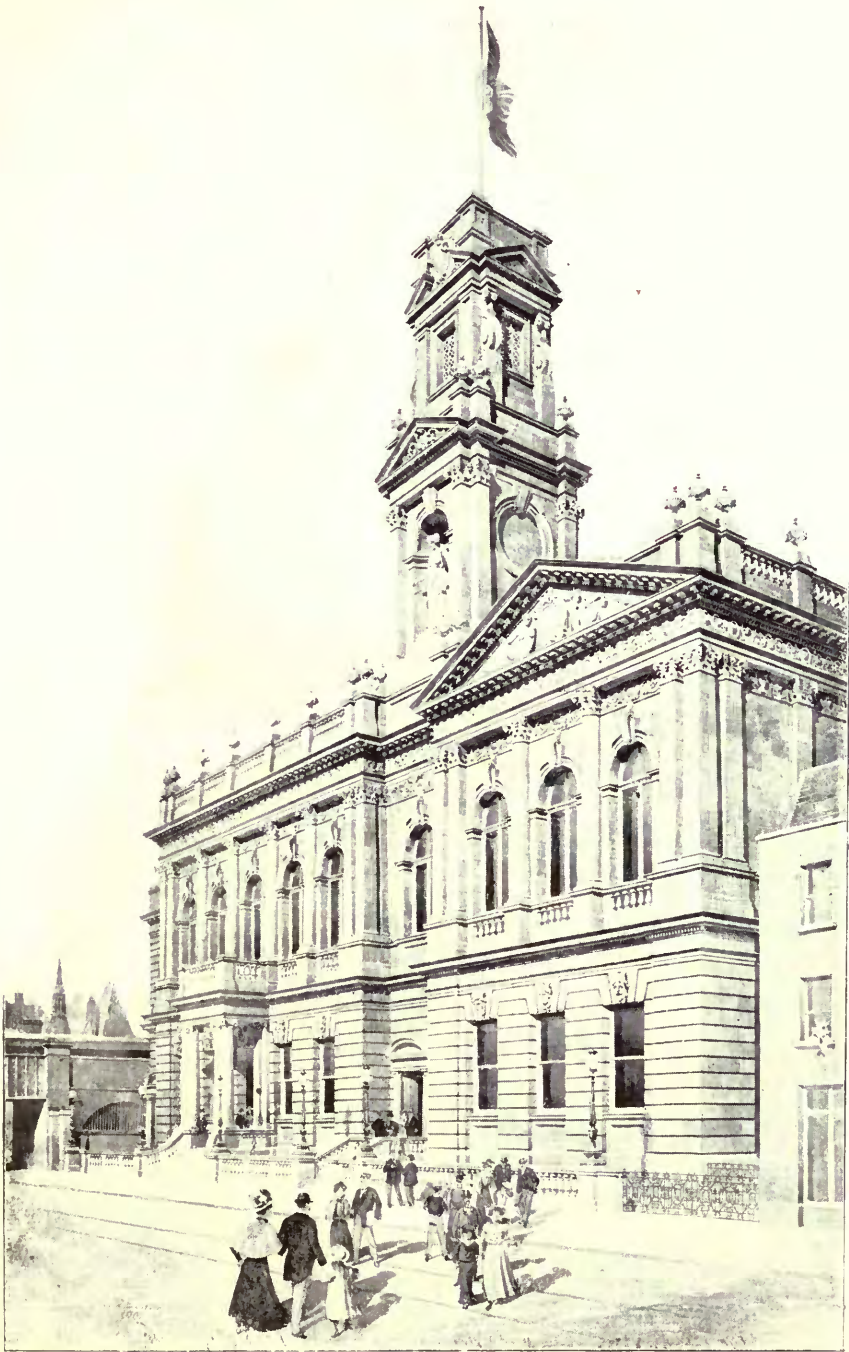
1365. Shoreditch Town Hall, Old Street, WILLIAM G. HUNT, Architect. (For Plans, see p. 11.)
