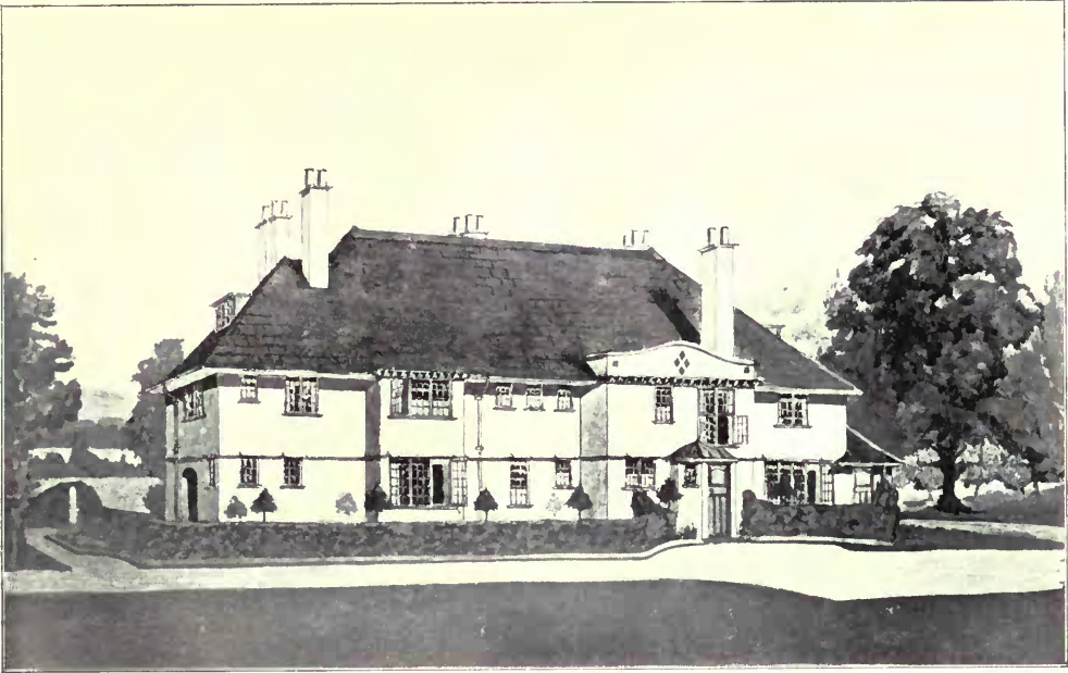
House at Limpsfield, North Front.
