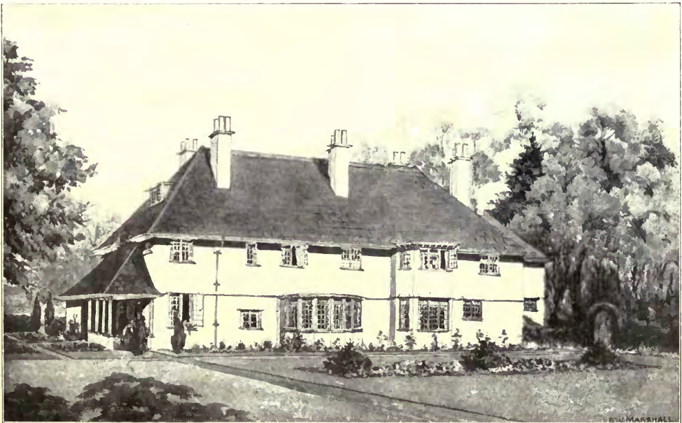
House at Limpsfield, South Front , ERNEST W. MARSHALL, Architect. (For Plans, see p. 114.)
