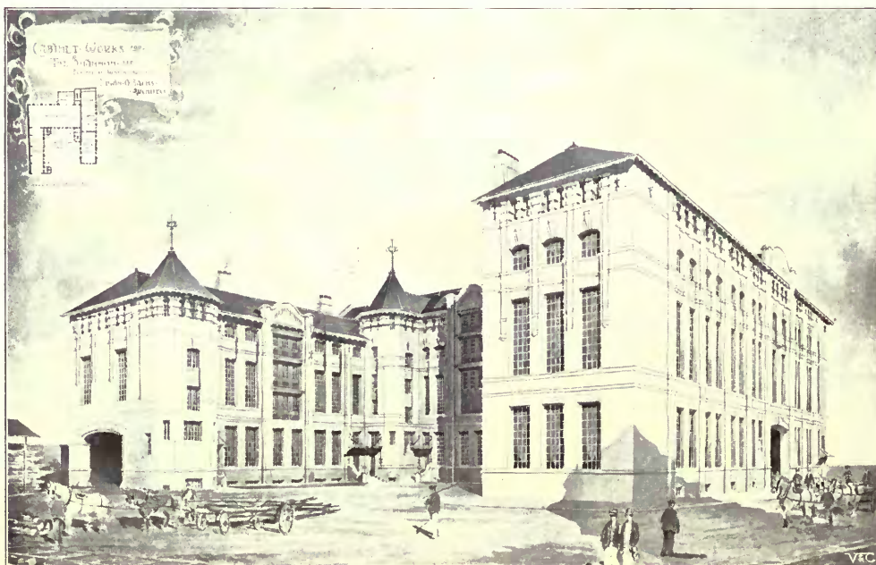
1404. The Shannon Factory, Dalston , EDWIN O. SACHS, Architect.
