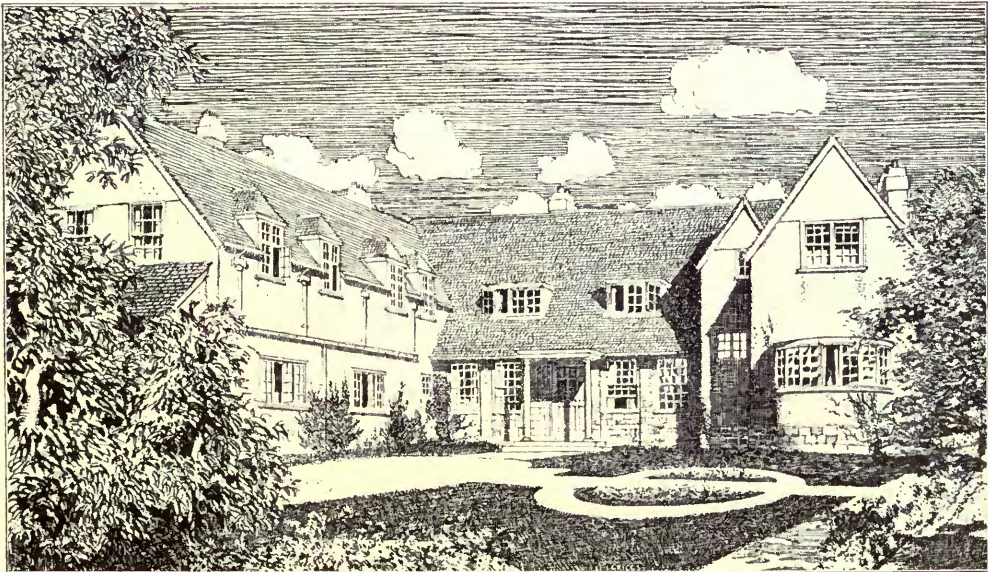
House at Forest Row, Entrance Front, E. M. P. FISHER, Architect. (For Plans, see p. 94.)
