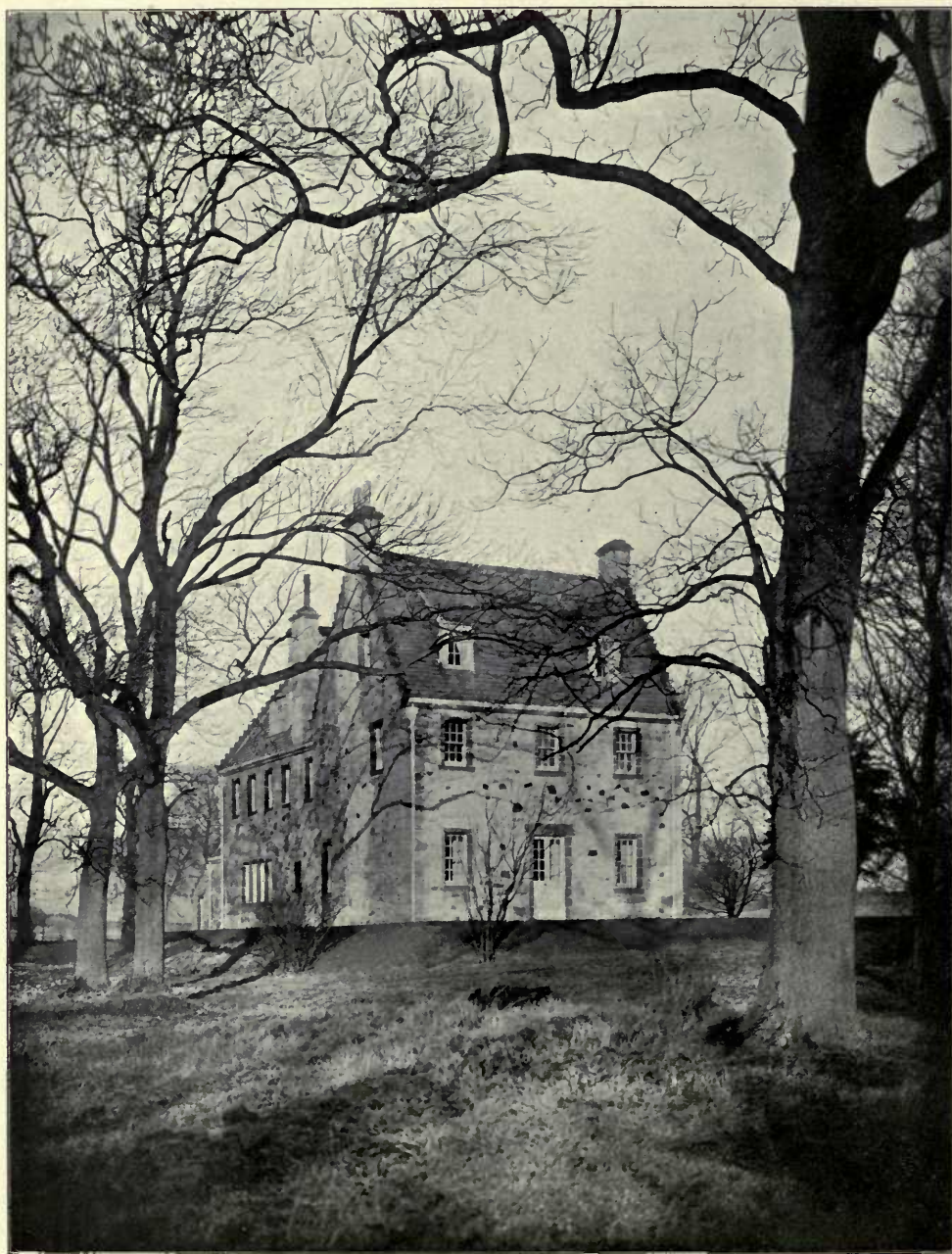
703. Boghall, Baldernock , GARDNER AND MILLAR, Architects. (For Plans, see p. 71.)
