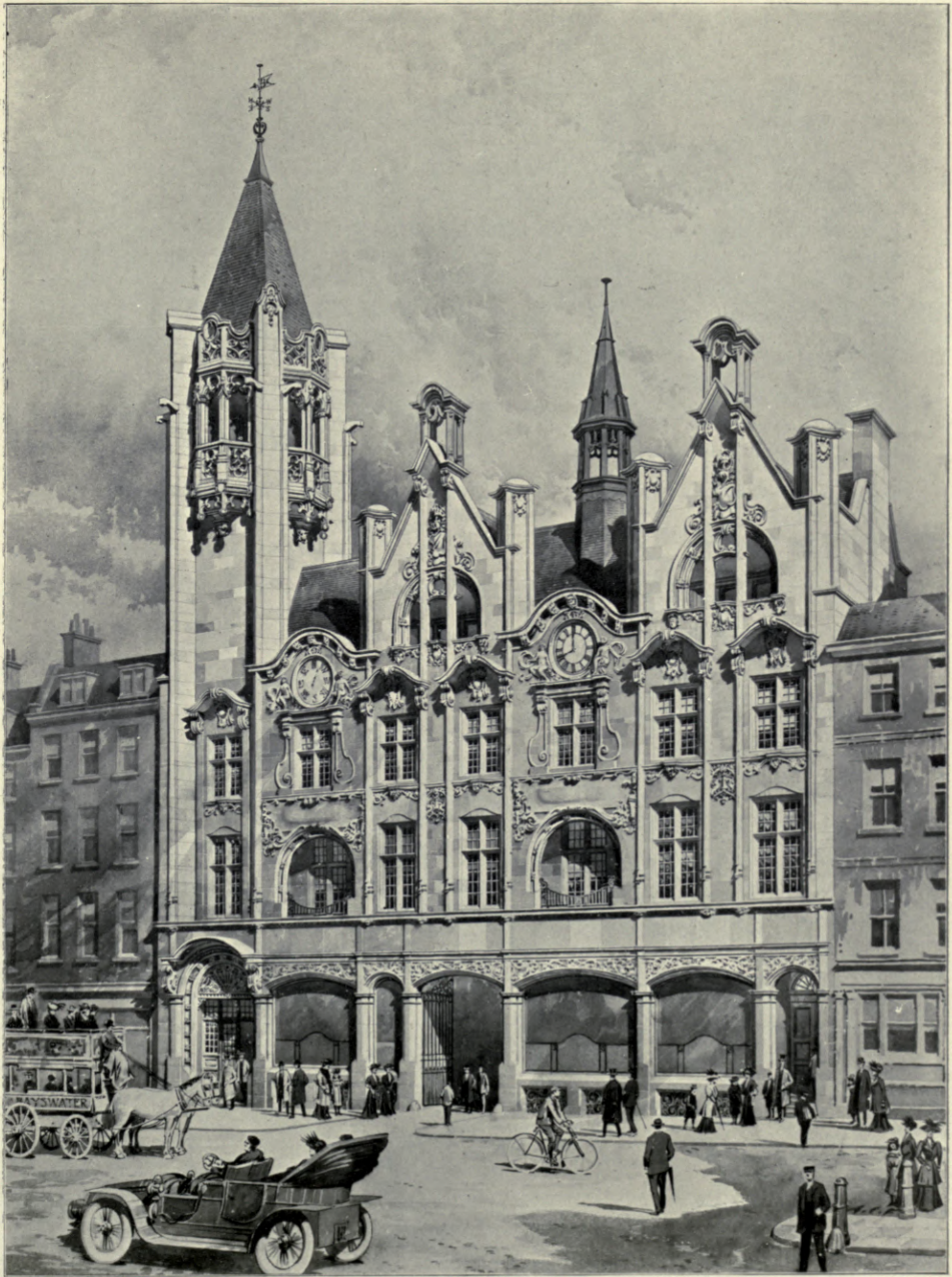
Additions to Messrs. Buchanan's Premises, Holborn, W.C., TREADWELL AND MARTIN, Architects. Contractor: F. G. Minter, Ferry Works, High Street, Putney, S.W. Constructional Steelwork and Fire Resisting Floors on the "Smith Walker" System by: Smith Walker and Co., 11 Tothill Street, Westminster, S.W. The Purbeck-Portland Stone Front up to First Floor level by: The Purbeck Portland Stone Co., Ltd., 11 Tothill Street, Westminster, S.W.
