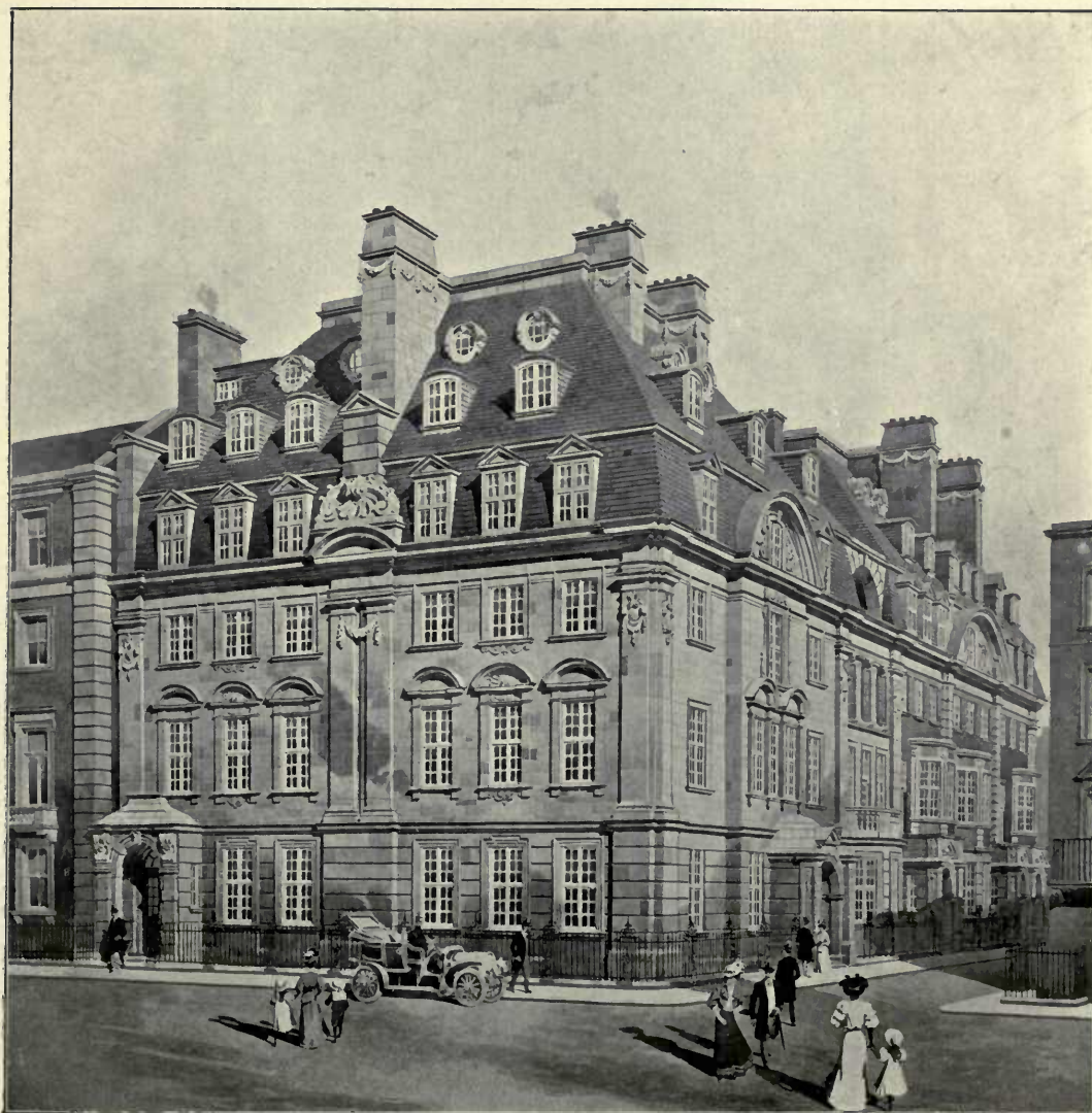
1503. Rebuilding in Upper Grosvenor Street, Mayfair, W. D. CARÖE, Architect. Building Owners: Higgs and Hill, Ltd., Crown Works, South Lambeth Road, S.W.
