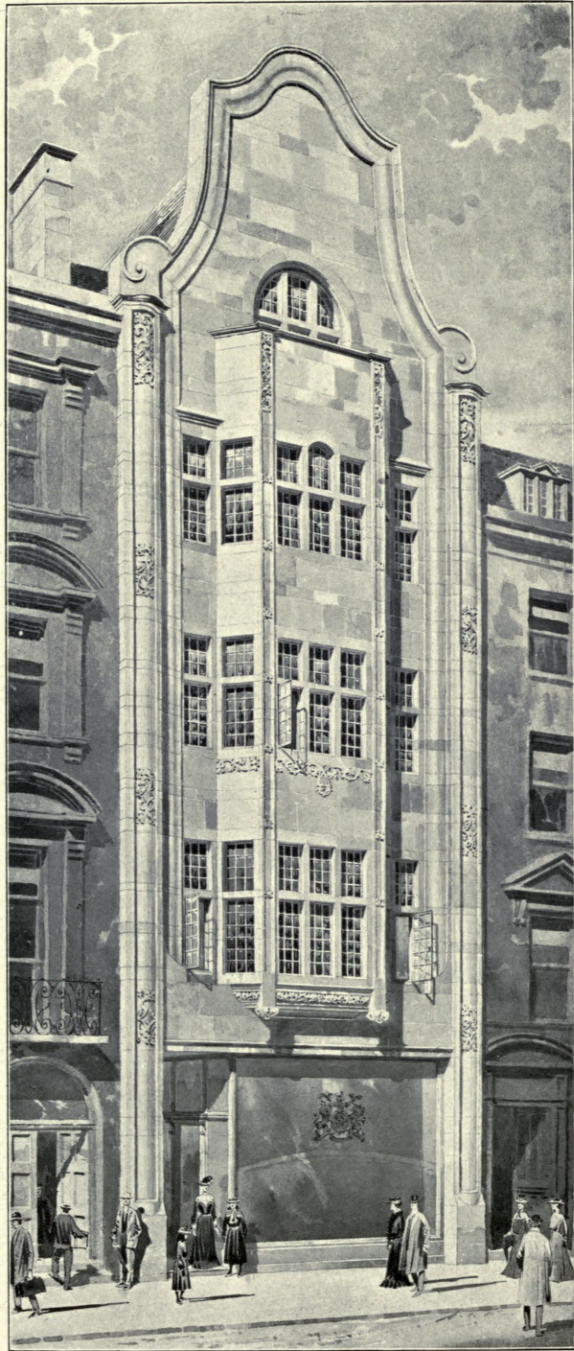
No. 20 Conduit Street, W., TREADWELL AND MARTIN, Architects. Steel Construction; Smith Walker and Co., 11 Tothill Street, Westminster, S.W.
