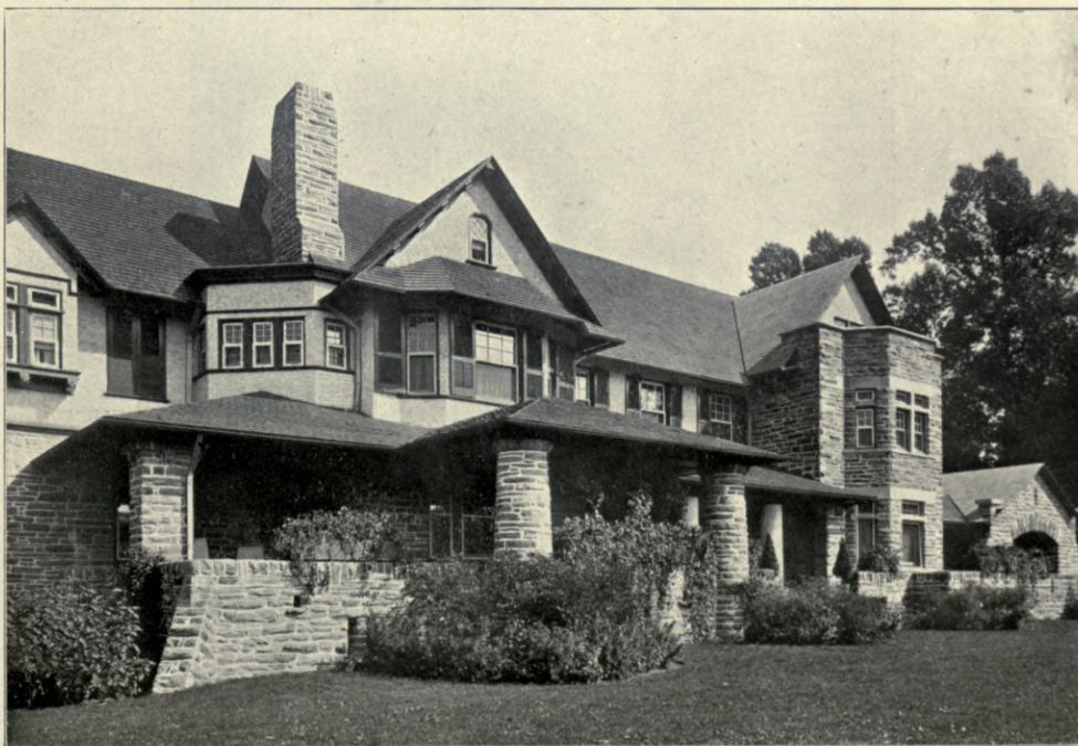
Residence at Bryn Mawr, Pa., D. KNICKERBACKER BOYD, Architect. (For Plans, see p. 125.)
