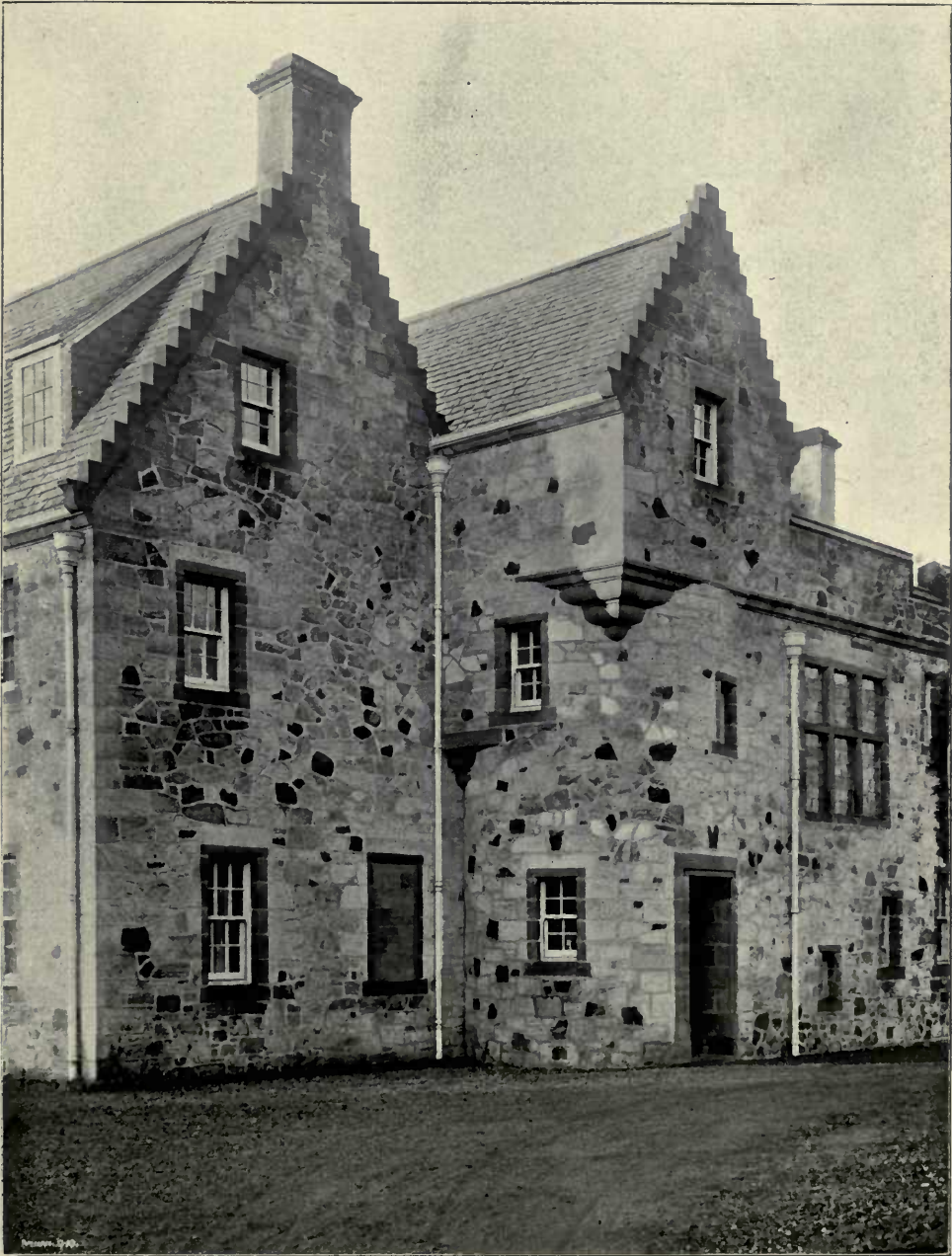
703. Boghall, Baldernock, GARDNER AND MILLAR, Architects. (For Plans, see p. 71.) Builders ; R. and A. Anderson, 2 and 3 Parliamentary Road, Glasgow.
