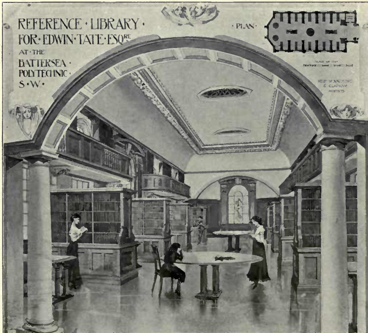
1374. Reference Library for Edwin Tate, Esq., at the Battersea Polytechnic, F. DARE CLAPHAM, Architect.
