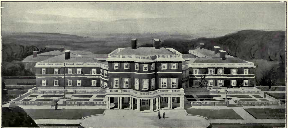
1463. Bicton Hall , Devon, WALTER TAPPER, Architect. (For Plans, see p. 35.) Oak and Pine Joinery and Stone Mantel Pieces: J. Jarvis and Sons, Ltd. , 253 Hackney Road, London, N.E.
