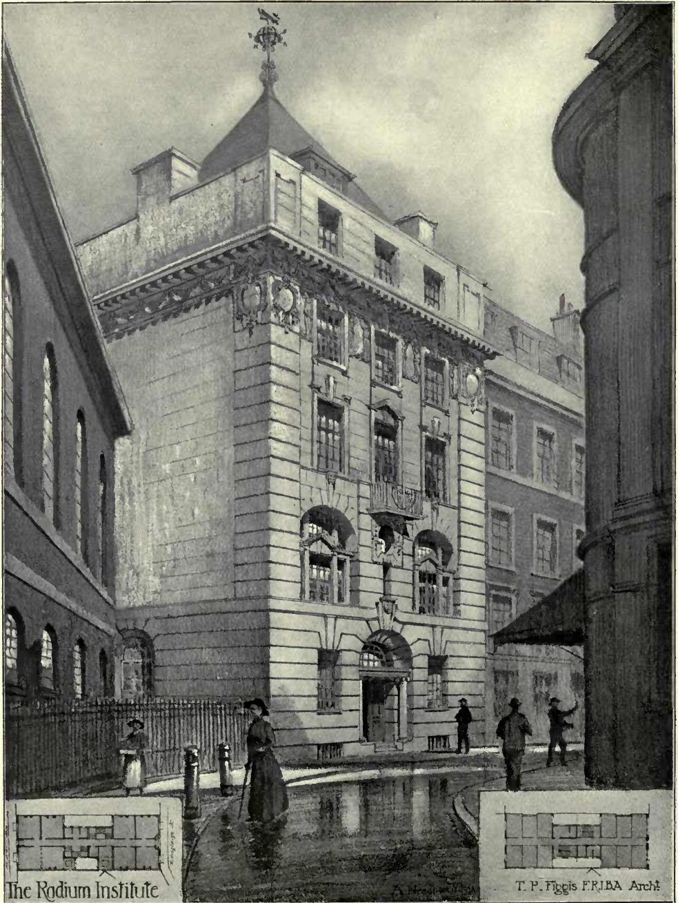
The Radium Institute, T. P. FIGGIS, Architect. Contractors and Engineers: W. J. Fryer and Co., Brawingdon Works, Paddington, W. Heating: Rosser and Russell, 22 Charing Cross, S.W. Electric Light, Duncan Watson and Co., 62 Berners Street, W. Lifts: Otis Elevator Co., Ltd., 4 Queen Victoria Street, E.C.
