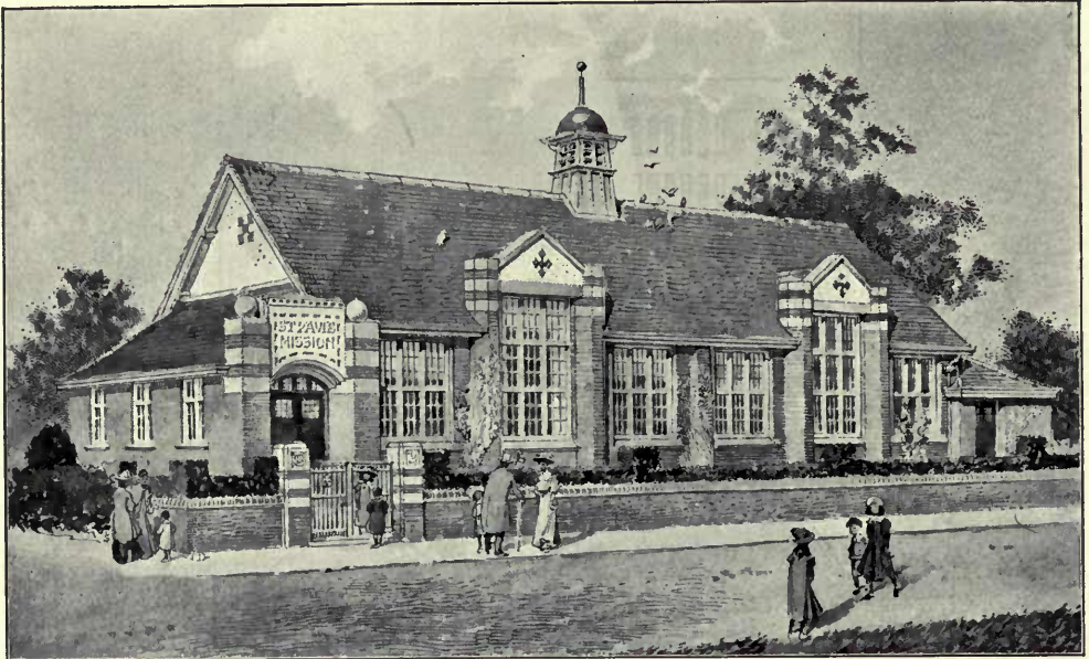
1488. St. Paul's Mission Hall , DAVID BIRD, Architect. (For Plans, see p. 33.) Contractors, W. Thorpe and Sons , Chester Road, Manchester.
