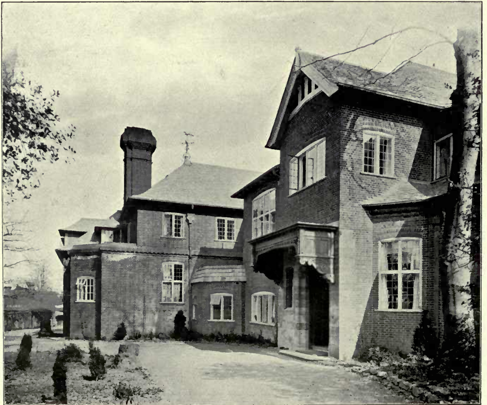
330. Pattishall House, Northamptonshire, View of Main Entrance, HAROLD O. TARBOLTON, Architect. General Contractors: Henry Martin, Ltd., Thenford Street, Northampton. Stone Slating fixed by: Wm. Close and Son, Colleyweston, Stamford.
