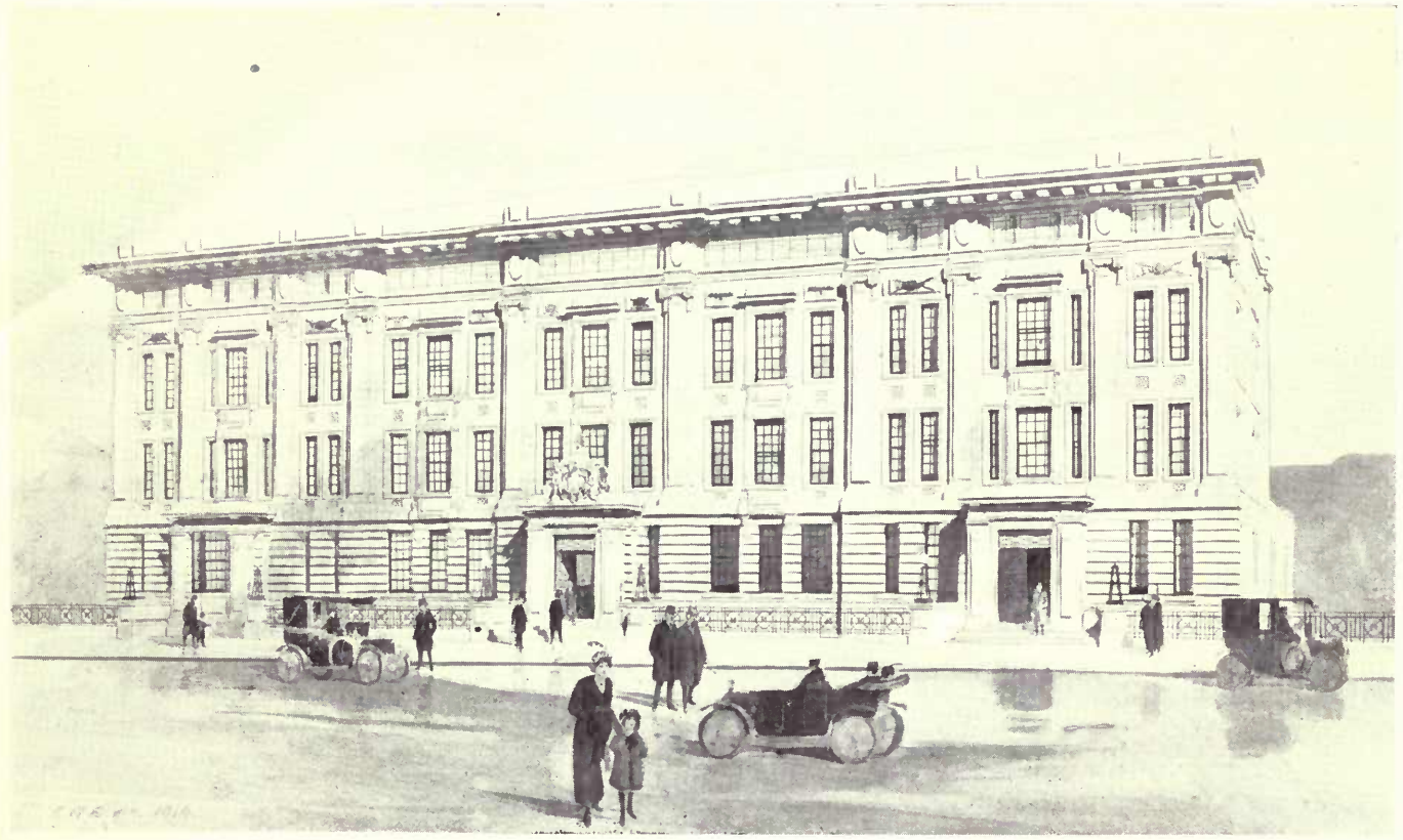
New General Offices, Metropolitan Railway, Baker Street Station, N.W.
