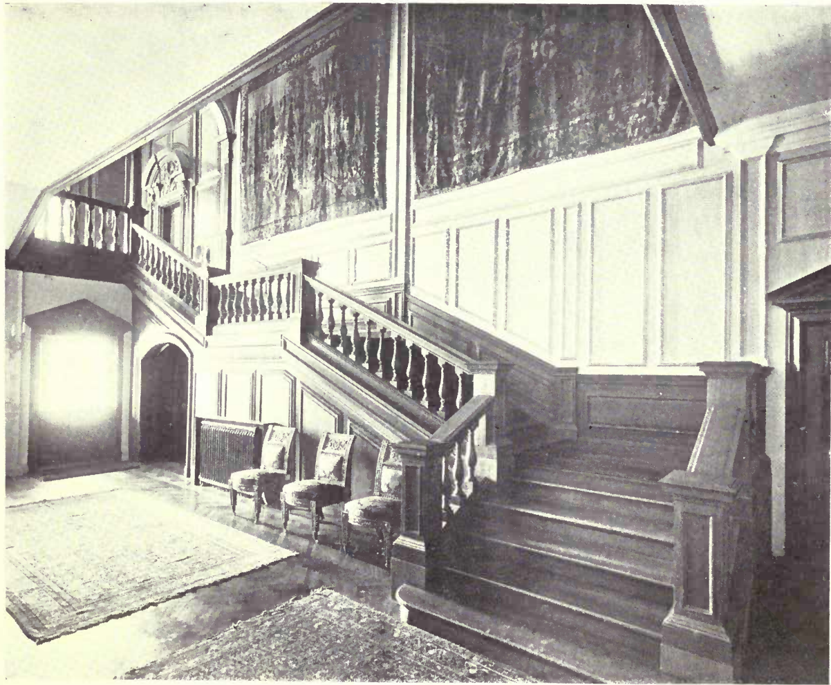
South Hill Park : The Staircase.
