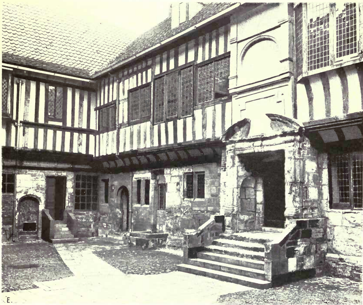
Restoration of St. William's College, York: The Court.
