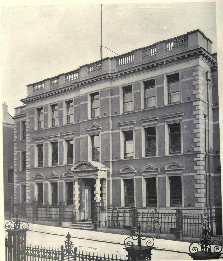
Council Offices Extension, Derby.
