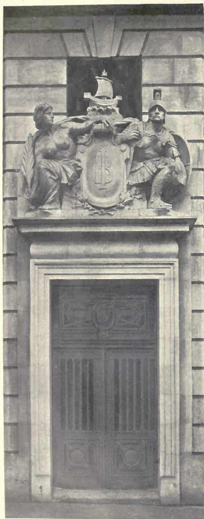
Imperial Buildings, Kingsway.
