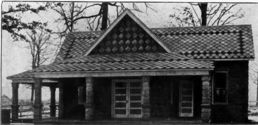
This Building, on the Wapakoneta Fair Grounds, is Covered With U. S. Cement Roofing
