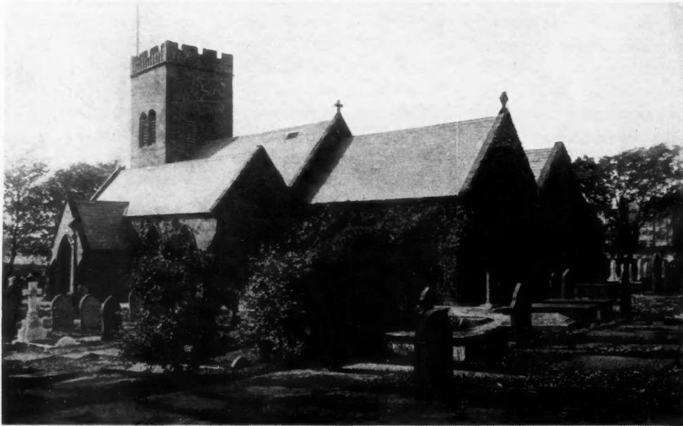
Parish Church, West Kirby
