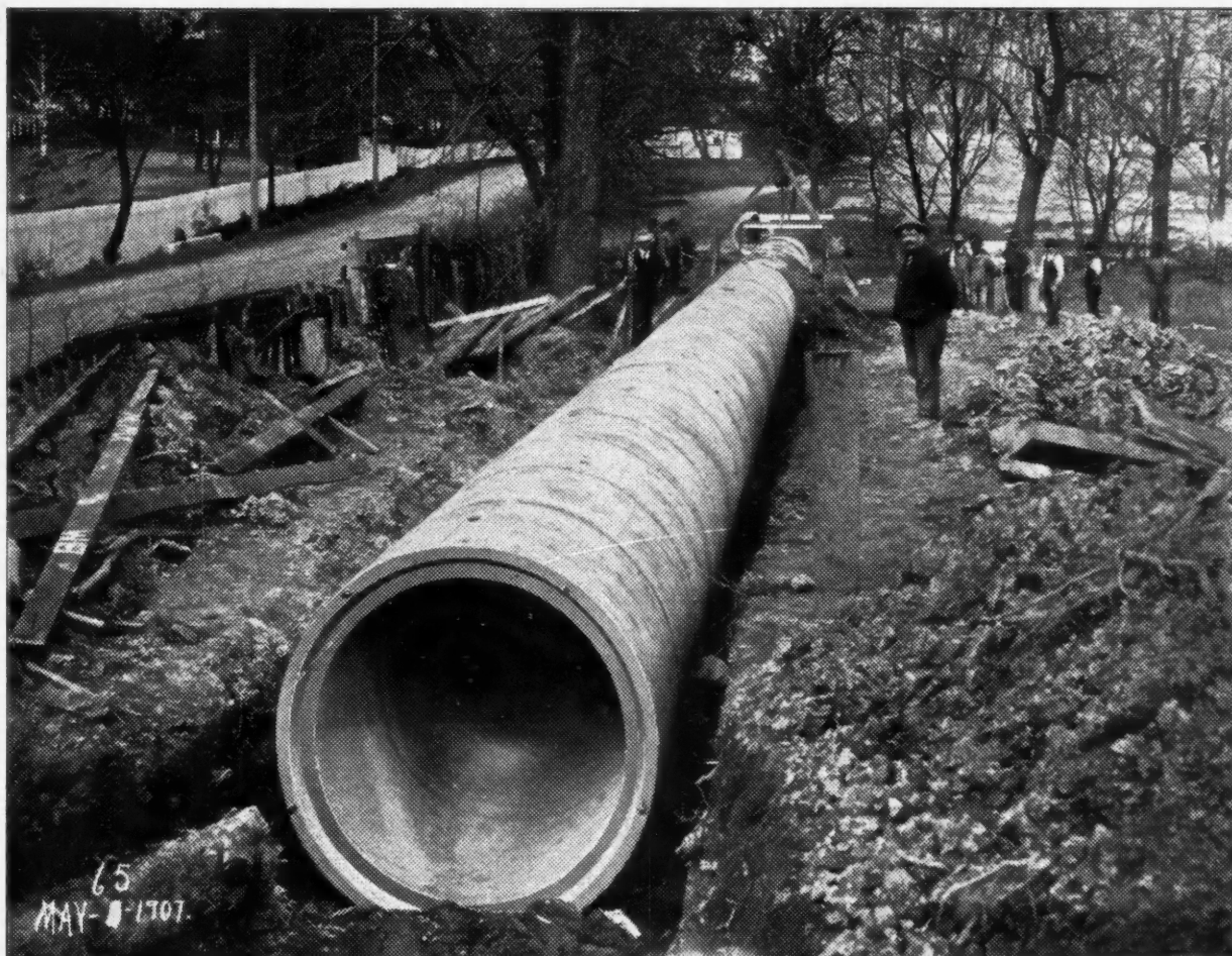
Forty-eight inch Reinforced Concrete Pipe used in the Baltimore Sewerage System, now in course of construction at Baltimore, Maryland.
