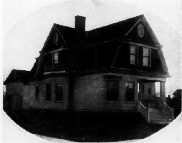
No. 32. Front Elevation, Home of A. H. Estes, Mendon, Mich. Chas. Blue, Architect.
