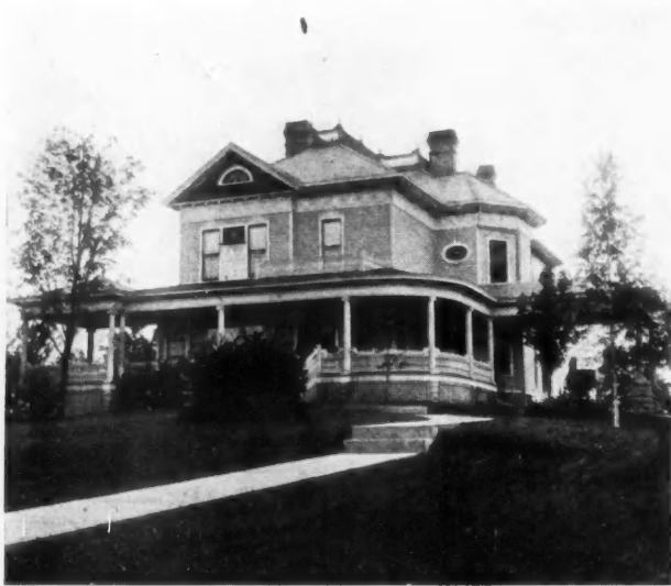
No. 30. Home of C. G. Shepard. L. D. Malone, Builder, Shelby, Ohio.
