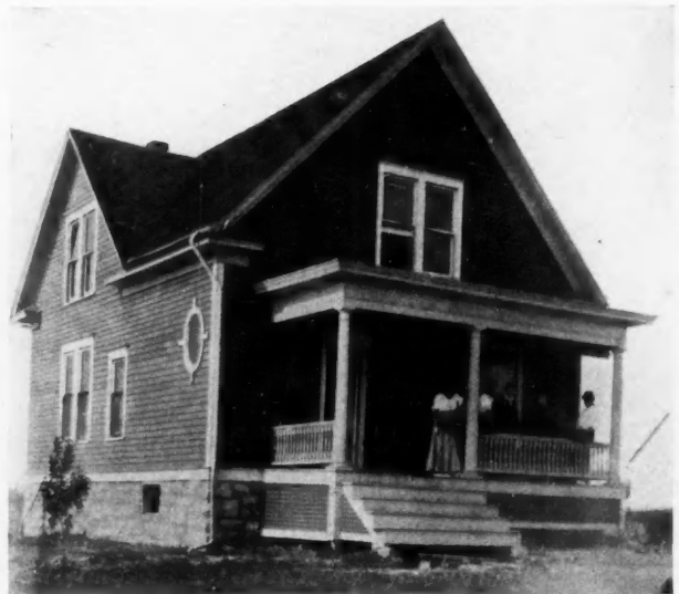
No. 76. Home of C. W. Phillips, Columbia, Mo. F. O. Kirby, Architect. Cost $1,980.
