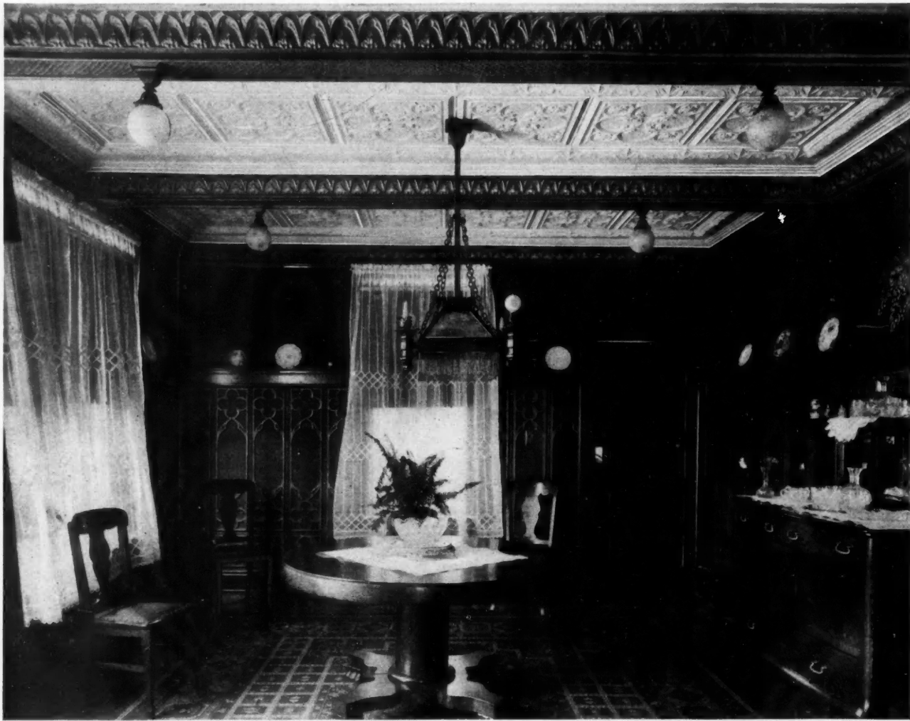
Dining Room with Metal Ceiling and Side Walls
