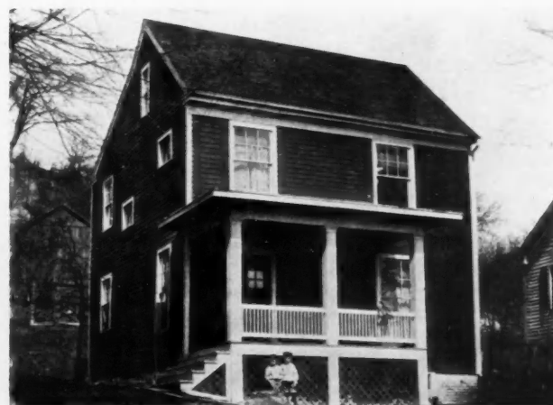
No. 80. Built by Mark A. Stewart, Louisiana, Mo.
