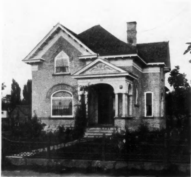
No. 94. Residence of W. A. Jones, Spanish Fork, Utah. Robertson Stebbins, and E. Hanson, Contractors.
