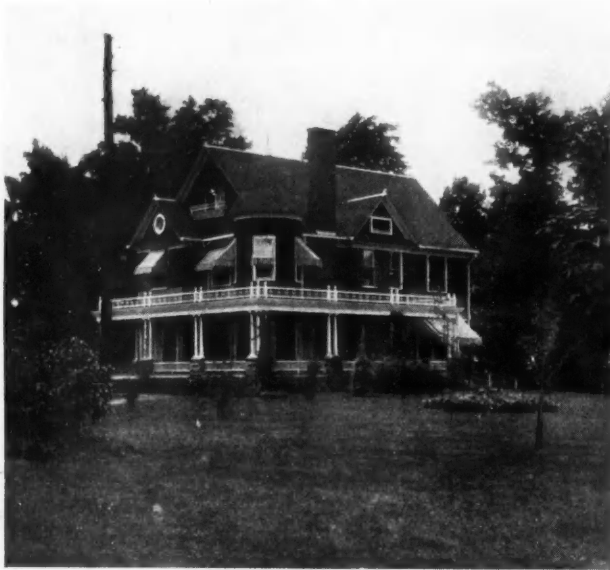
No. 31. Home of W. H. Skiles, Shelby, Ohio. L. D. Malone, Builder.
