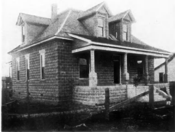
No. 71. Concrete Block House. Built by Noah Norman, Blodgett, Mo.
