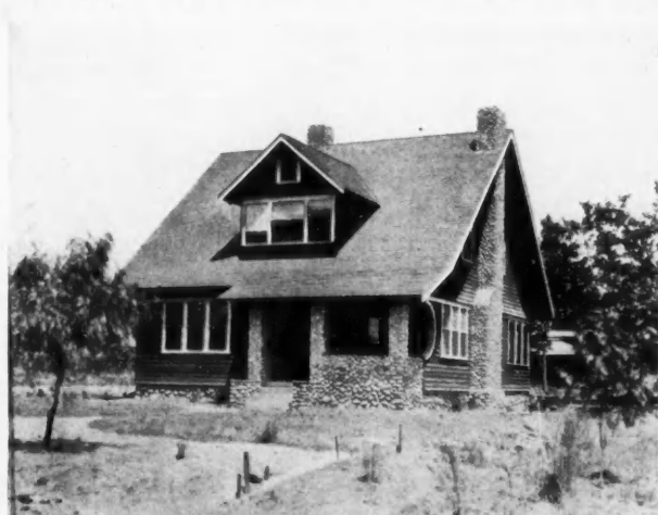
No. 100. Home of W. H. Stinson, Claremont, California. ers, and was designed and built by E. E. Thomas, at Pasadena, Cal. The dimensions of the same are 32 by 38. There is also a large porch, 8 by 28 feet, across the entire front of the house. There are six rooms
