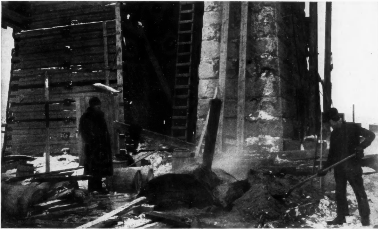
Sheet Iron Kiln for Heating the Sand and Cement for the Mortar
