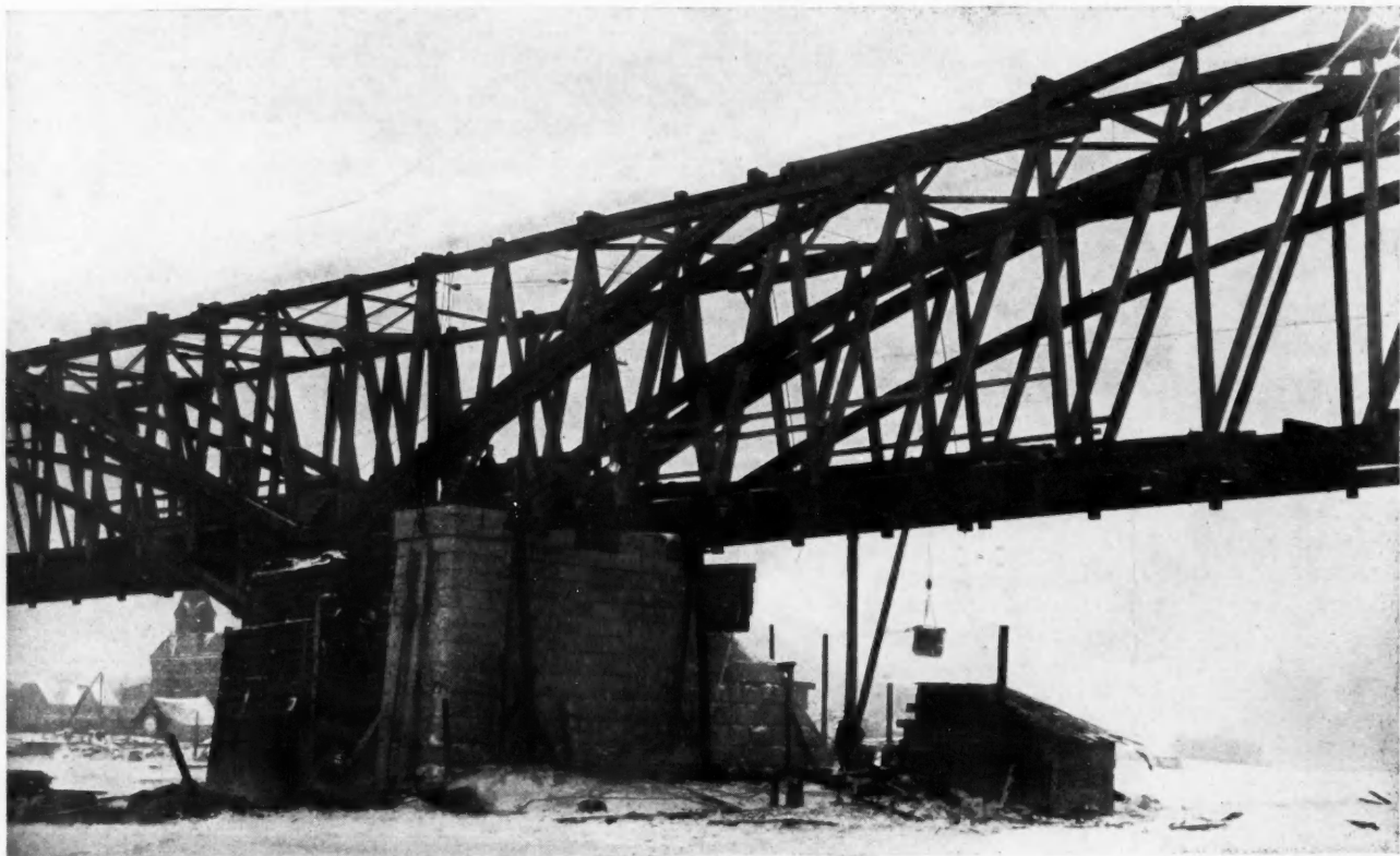
General View Showing New Granite Pier Alongside Old Cribwork Pier
