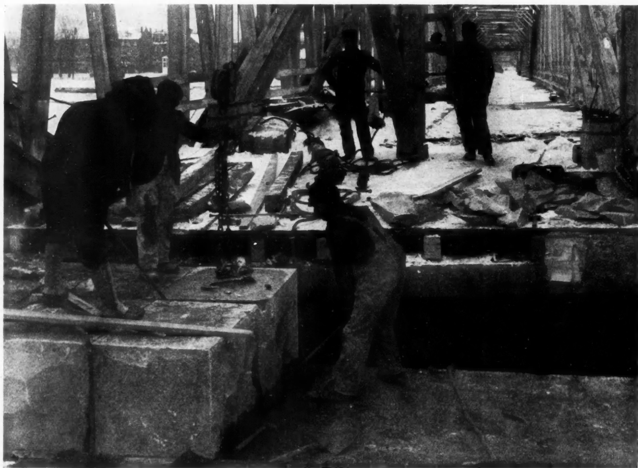
Laying the Top Course of Pier
