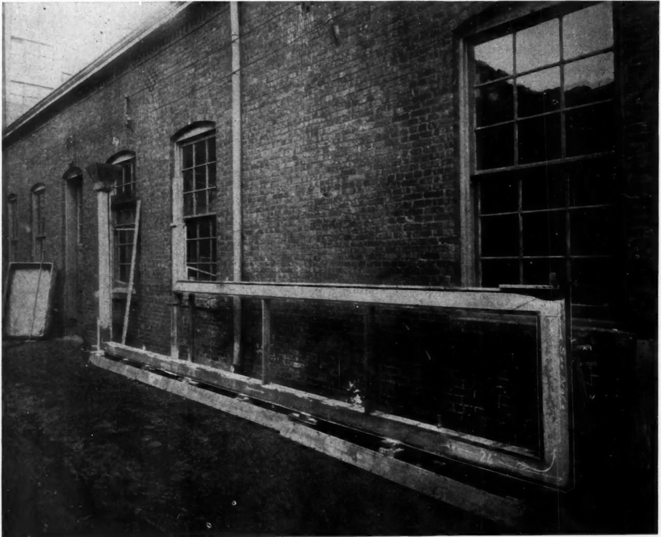
Test of the Edison Mixture—Note the Funnel Where Pouring Was Done
