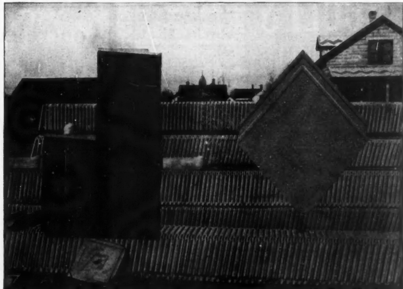
Europa and New Era Concrete Roofing Tile, Showing Different Size and Form of Tile
