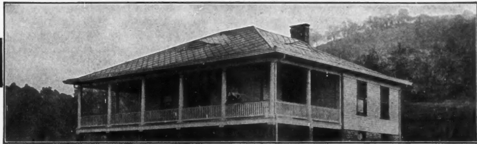
Asbestos "Century" Shingle Roof—Dayton Gun Club, Dayton, Ky.; William Lampe, Newport, Ky., Architect; R. L. Brown, Covington, Contractor
