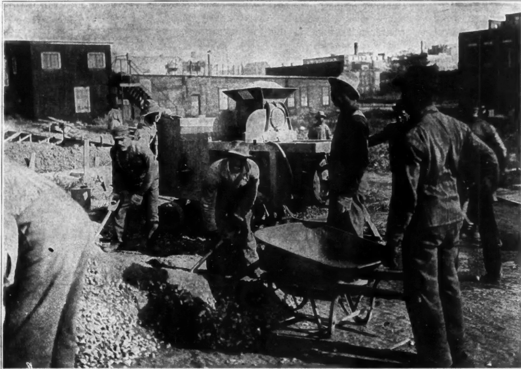
No. 9 Coltrin on Foundation Work, Kansas City, Mo.
