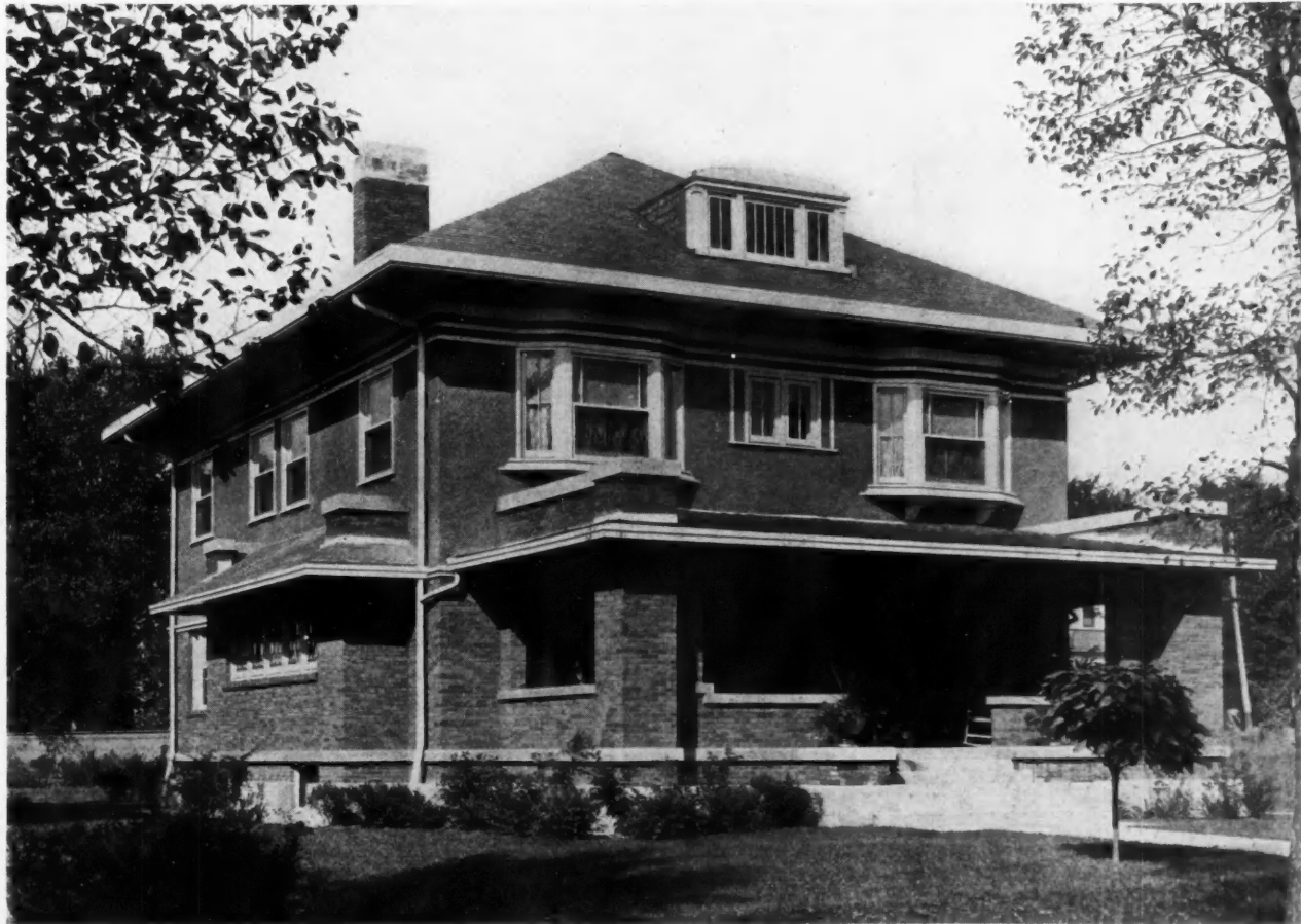
Cement Plaster Is Popular for the Very Highest Class of Work, Often in Combination with Face Brick—Jas. A. Dick's Residence, Oak Park, Ill.
