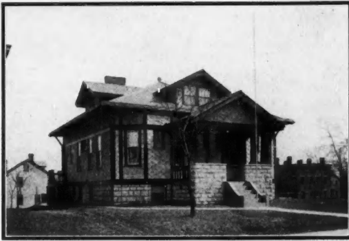
Asbestos "Century" Shingle Roof and Sheathing—Residence of W. E. Crawford, Evanston, Cincinnati, Ohio: Fasse & Reed, Cincinnati, Architects; Bryen, Vane & Anderson, Cincinnati, Contractors.
