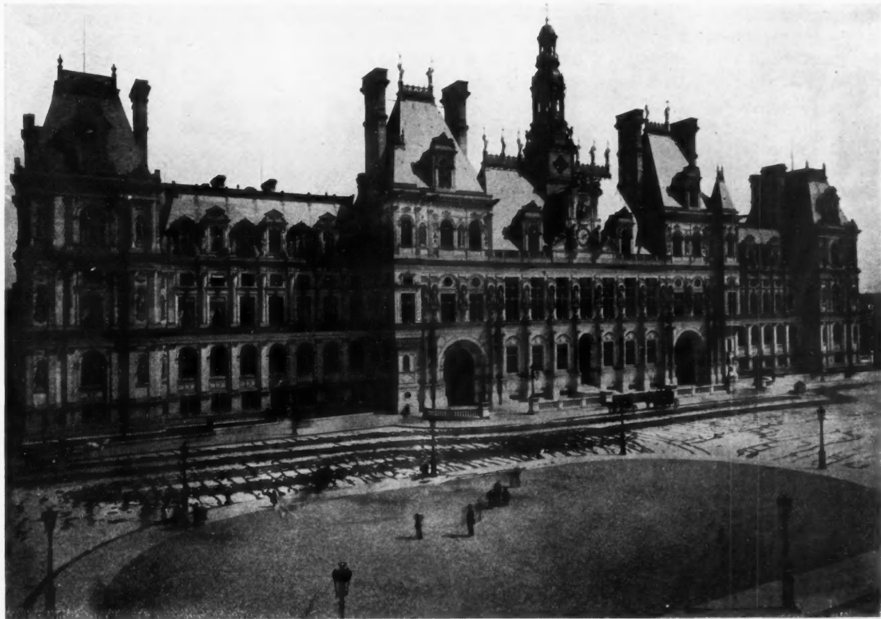
Principal Facade of the Hotel de Ville, Paris
