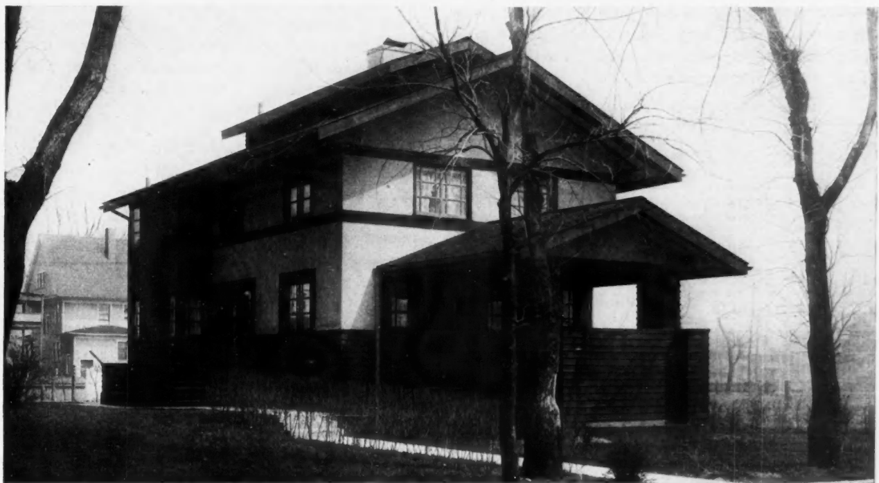
An Artistic Combination of Rough Boards and Plaster; Inexpensive, Attractive and Substantial
