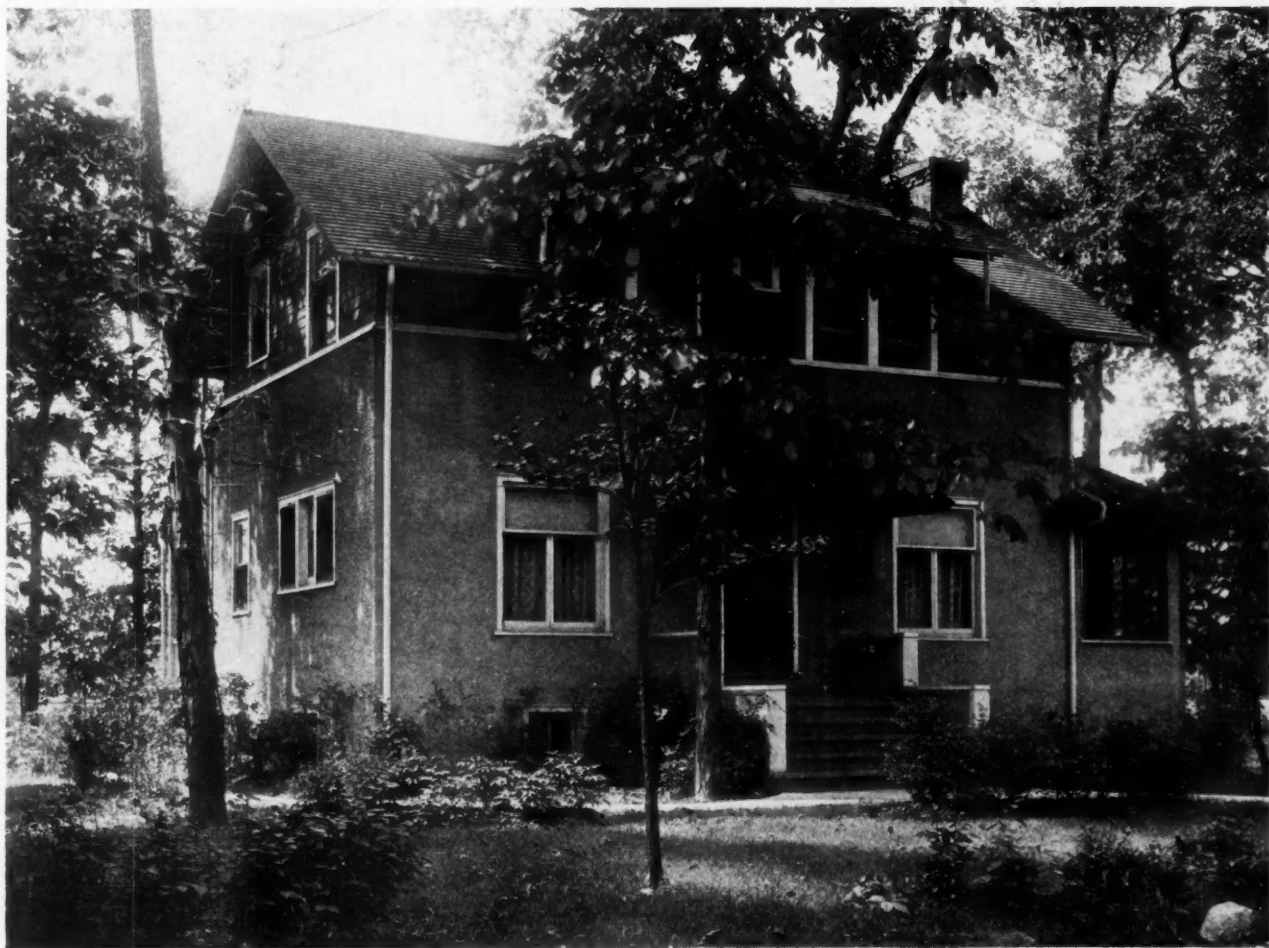
Rough Cast Stucco from Grade to Second-Story Windows, Shingles Above—Residence of Chas. Van Deursen, Kenilworth, Ill.
