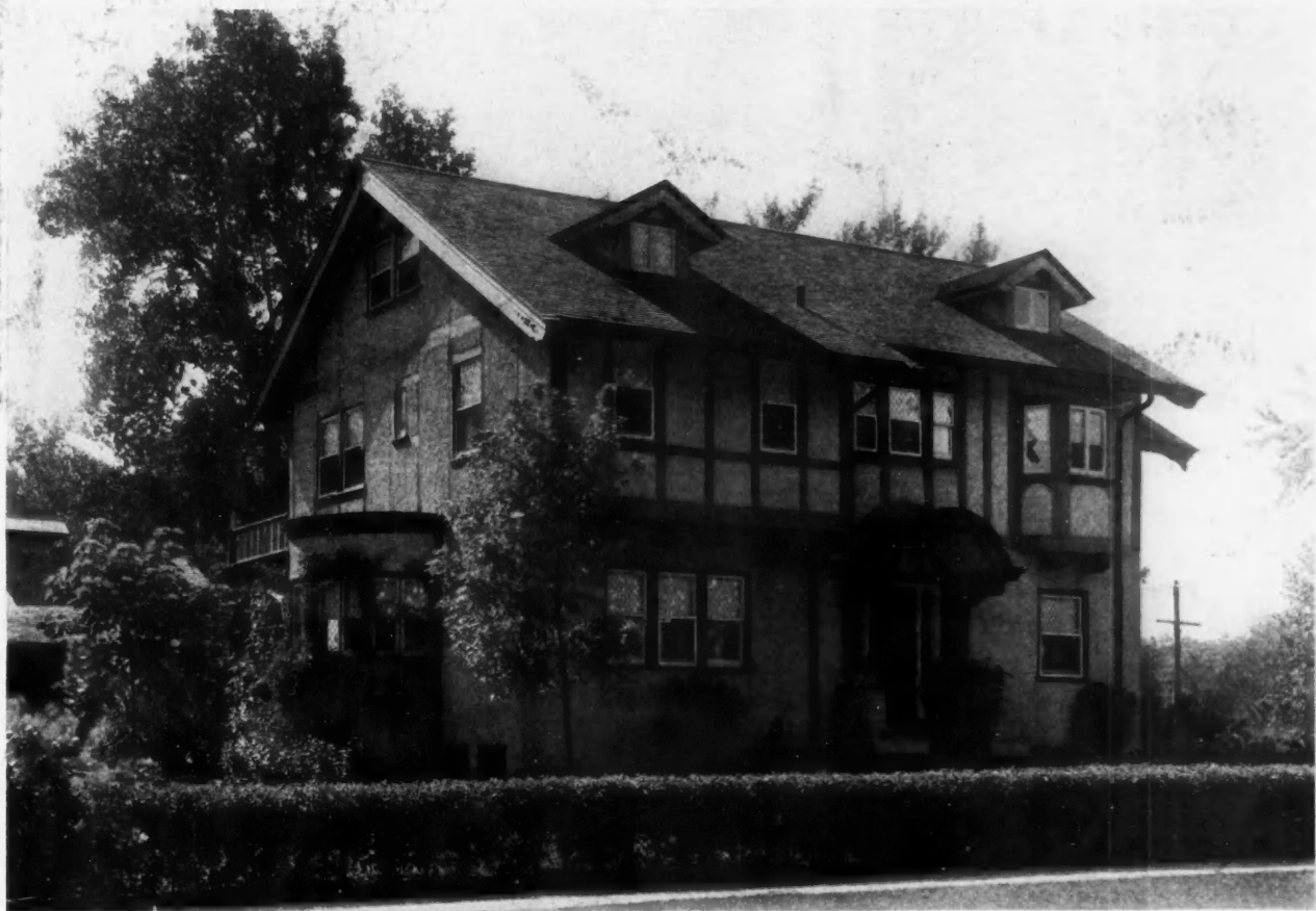
Delightful Use of Cement Plaster with Exposed Timbers in the True English Style—Residence of A. H. Aylesworth, Wilmette, Ill.
