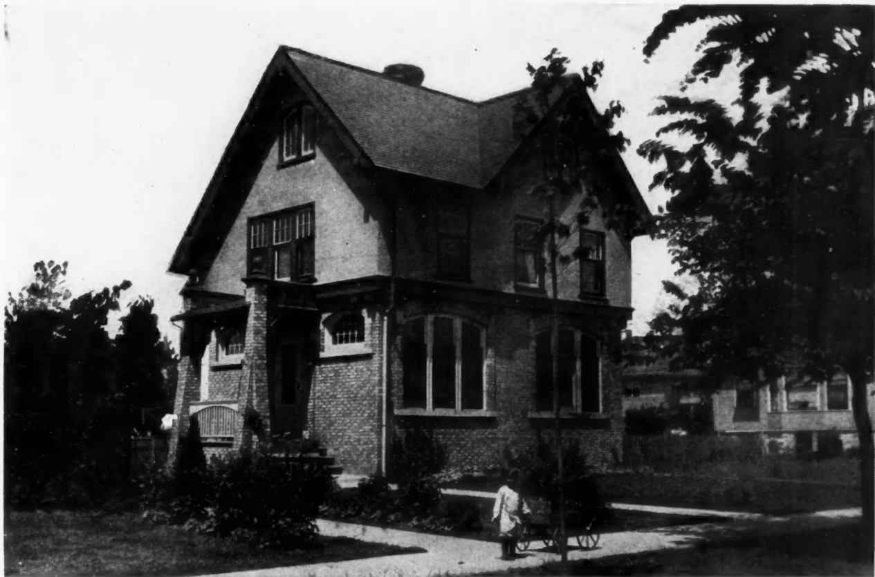
Beautiful Home of Mr. Harry Hobbins, Oak Park, Ill., Barfield and Herr, Chicago, Architects
