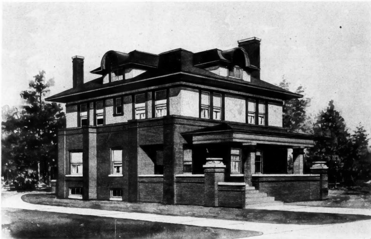
Beautiful Residence of Brick Veneer and Cement Plaster Designed for F. W. Schooly, Kansas City, Mo.
