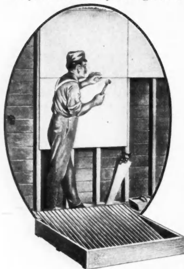
Showing application of Bishopric Wall Board to studding as a substitute for lath and plaster. Finished surface exposed, ready for decorations.
