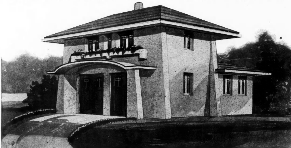
Two Story Private Garage with Living Quarters on Second Floor. Cost $2500.
