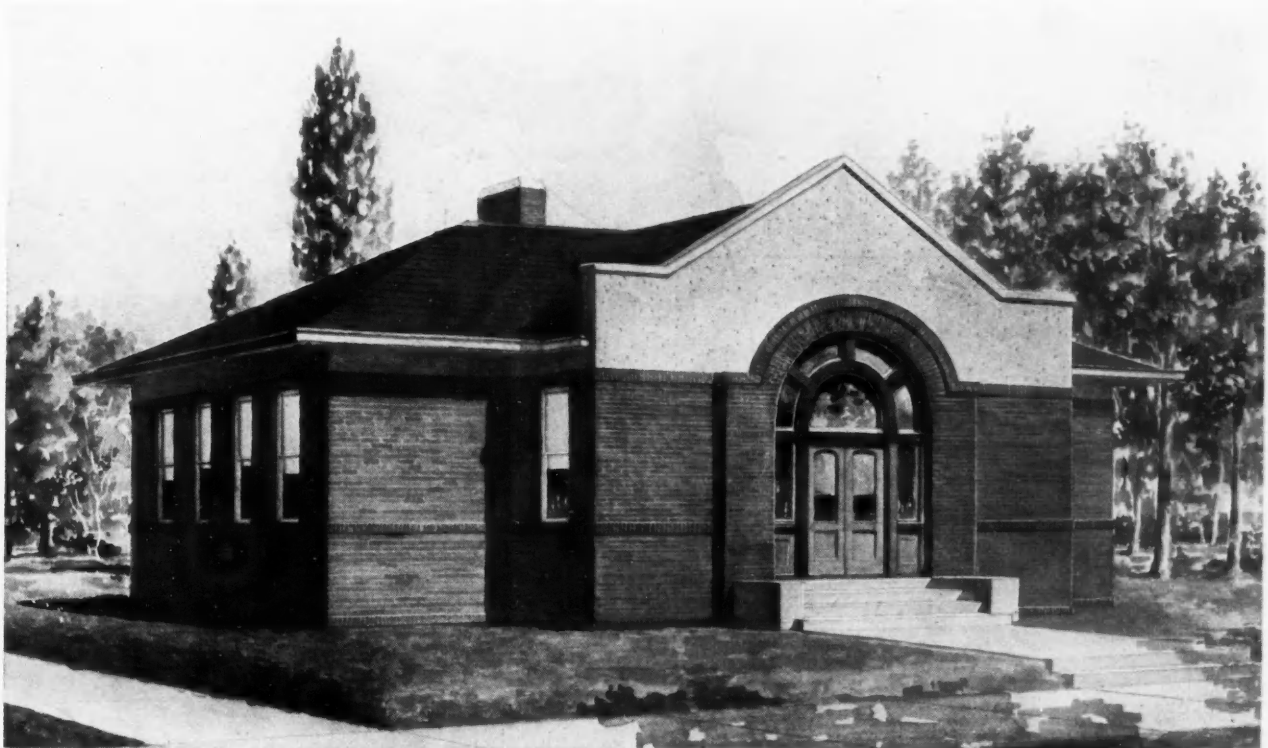
Well built Rural School Building of Brick Veneer and Cement Plaster, G. W. Ashby, Chicago, Architect
