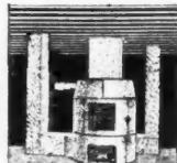
BASEMENT VIEW OF 1 ROOM PLANT. BEST WAY TO HEAT A ONE ROOM BUILDING
