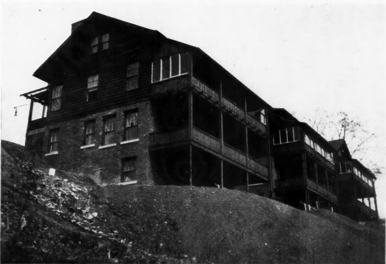
Rear View—Lots are Terraced—First Floor With Dining Room and Kitchen is Below Street Grade
