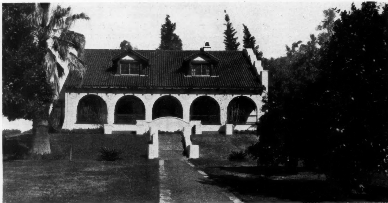
Simple Mission Design—Circle Arches, Cream Stucco and Tile Roof
