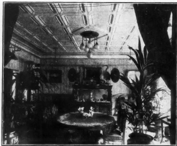
Beautiful Metal Ceiling in Modern Residence
