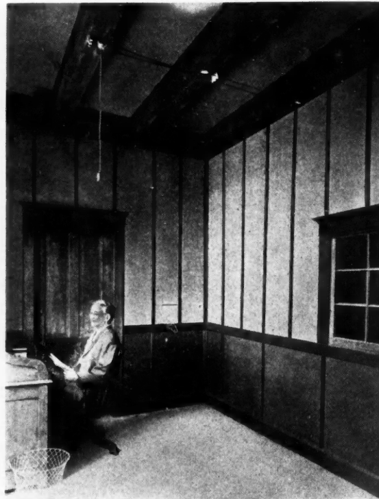
Paneled Interior Using Utility Wall Board
