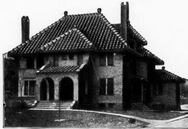
The Edwards Metal Spanish Tile Roof
