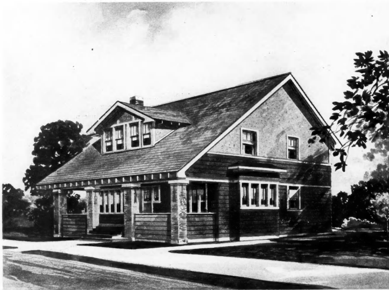
Eight Room Dwelling Sided with Rough Boards and Stucco.
