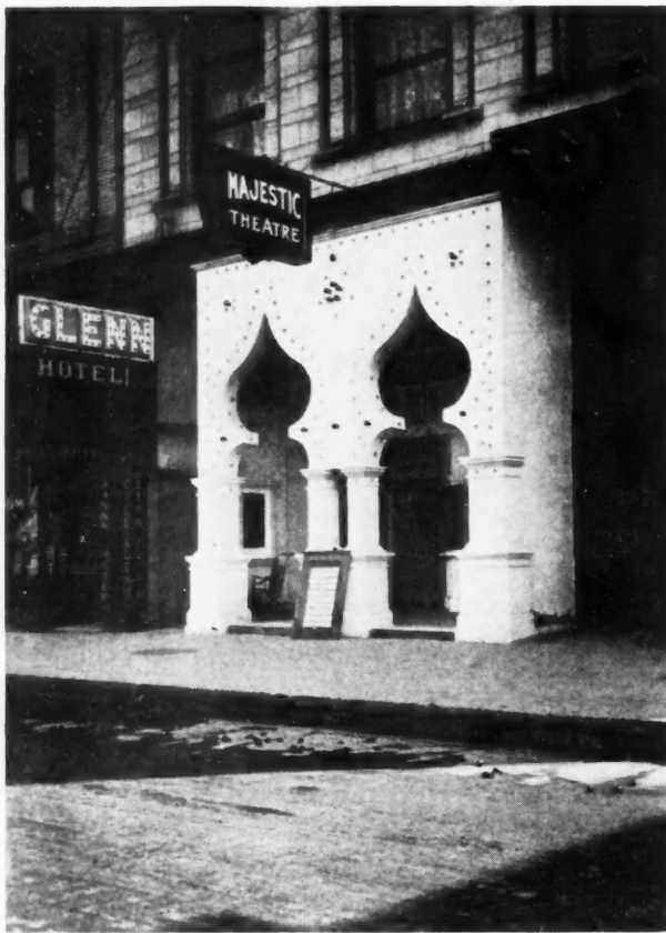
Fig. 1. Entrance Designed to Hide Center Supporting Post entrance will counteract the effect of any amount of decoration. Frequently the posts are spaced irregularly, which makes the trouble worse. This is some-
