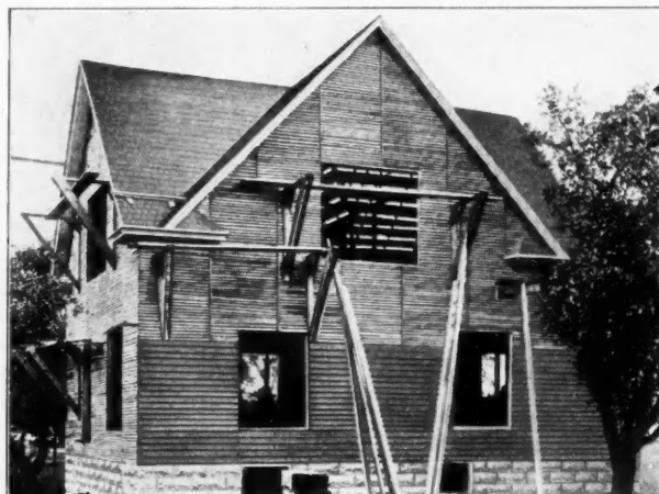
House With Clapboards Over Bishopric Sheathing
