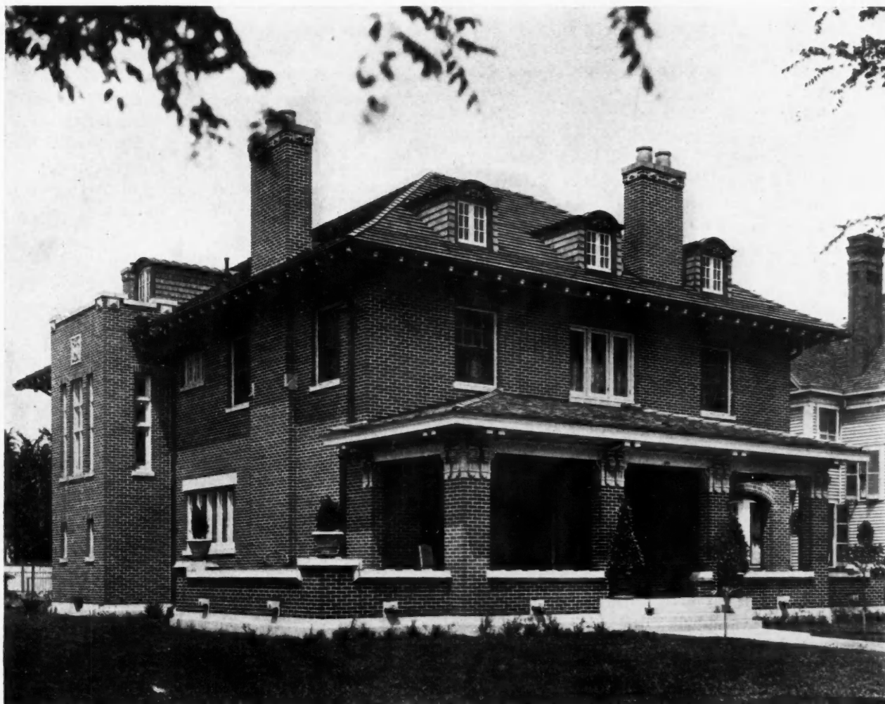
Beautiful Residence of John J. Cain, Columbia, S. C., Built of Rough Texture Brick with Wide Mortar Joints
