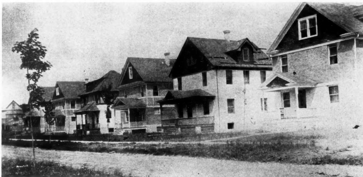
Row of Six Hollow-Wall Concrete Houses on Pullman Ave., W. N. Britton Addition, Rochester, N. Y. Finished Outside in Various Styles, but Built at Same Figure, $1,971.50—See Itemized Bill of Costs for Materials and Labor
