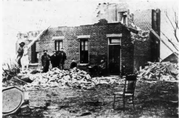
Brick House Wrecked by Tornado
