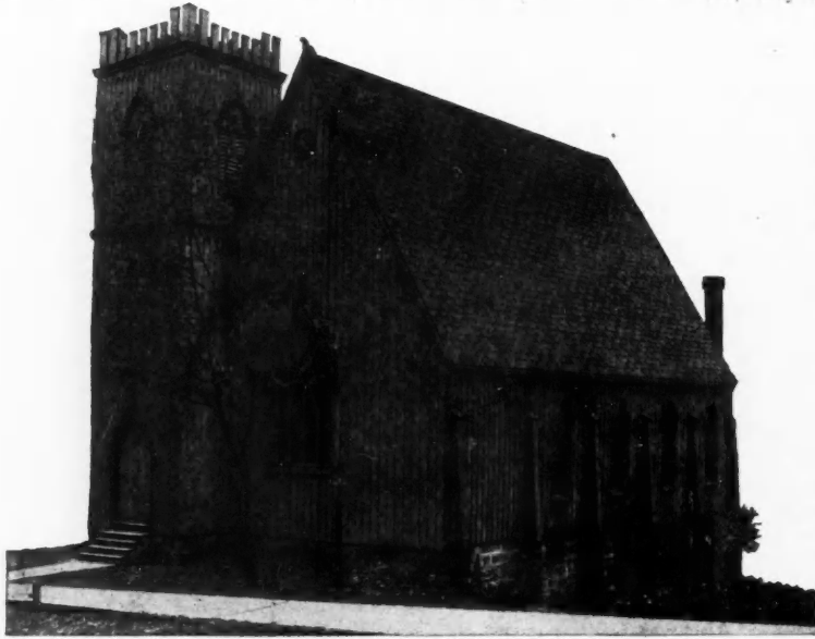
Shingled with "Eastlake" Shingles in 1889—Not One Cent for Repairs Since
