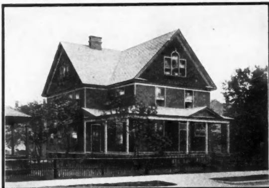
Asbestos "Century" Shingle Roof—Residence of George Jacka, Calumet, Michigan; Architect, Paul Humphrey MacNeil, Calumet, Michigan; Contractor, Edward Ulseth, Calumet, Michigan.
