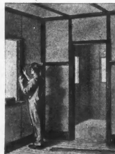
Before putting on decorative strips. Panels are painted at this stage.
