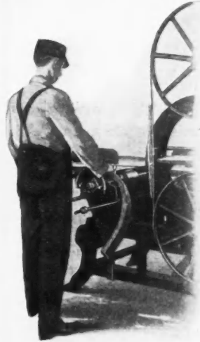
FAMOUS Universal Woodworker operated as Felloe Rounder.
