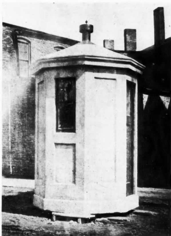
Erie Railroad Switchman's House. Monolithic Reinforced Concrete Construction.
