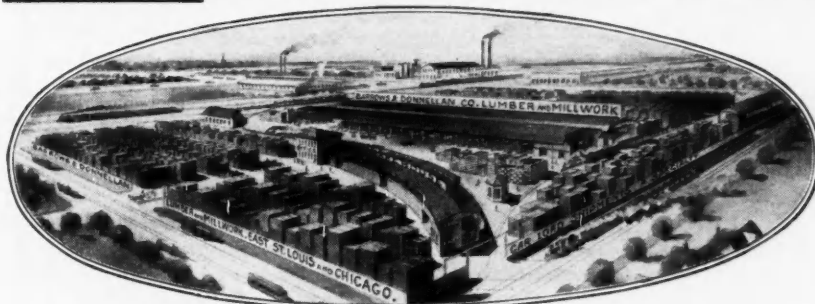
Nearly 10,000,000 feet in sight. This cut shows our big Southern Illinois Plant, situated where 27 Trunk Lines and 3 Interurban and Traction Systems have their terminals. Our customers get as prompt service as they could from their home lumber yard, and many other advantages which the local yard cannot offer them.
