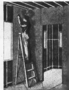
Nailing up panels.
