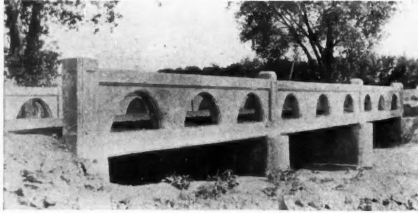
Reinforced Concrete Bridge in Webster County, Nebraska
