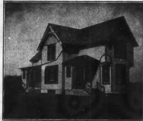
Farm Home of Mr. and Mrs. Robert Boston, Rollo, Illinois. Lighted for the past seven years by a Davis Acetylene Lighting System.
