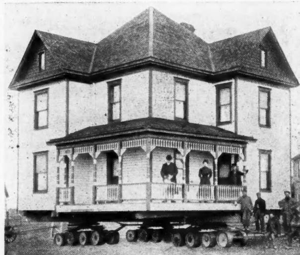
**Fig. 5 House Being Easily Moved on La Plant Trucks**
