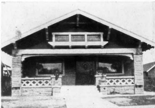
Four-Room Cottage Designed and Built by Edwin L. Markel, New Orleans, La.
