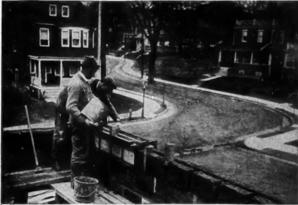
Making ready to insert the floor beams.
