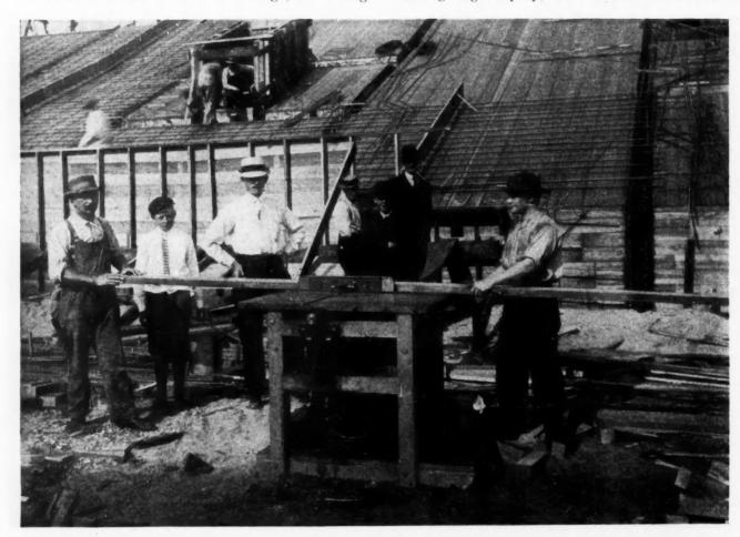
Portable Saw Rig With Contained Gasoline Engine at Work for Contractor Edw. L. Scheidenhelm of Chicago, Cutting Up Form Lumber on the University of Chicago Reinforced Concrete Grand Stand Job
