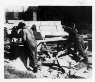
Portable Saw Rig Sawing Form Lumber on Big Reinforced Concrete Job for the Hanson Construction Co., Milwaukee, Wis.
