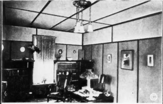
The walls and ceiling of this library in the home of Mr. F. S. Green, Nashville, Tenn., are made entirely of Beaver Board.
