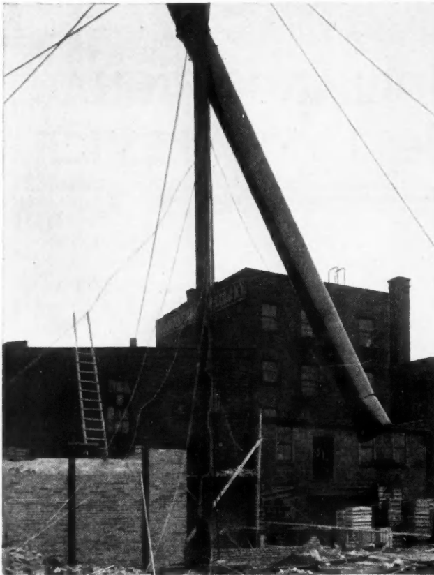
White Three-ton Truck Used to Hoist an 80 Foot Sheet Iron Smokestack Into its Cradle, Twenty Feet Above the Ground
