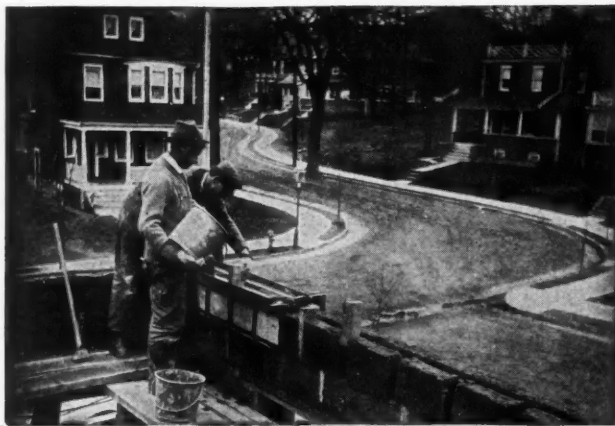
Making ready to insert the floor beams.
