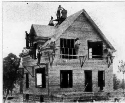
Reliable Folding Scaffold Brackets in Use. These brackets are made by the Elite Mfg. Co., Ashland, Ohio
