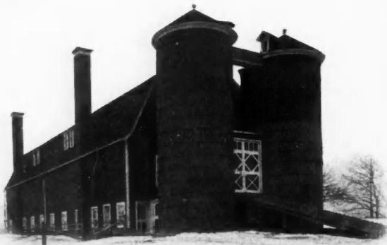
This Part Was Built First; Size 40 by 220 Feet, 22-Foot Posts
