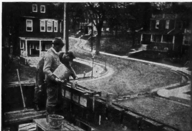
Making ready to insert the floor beams.
