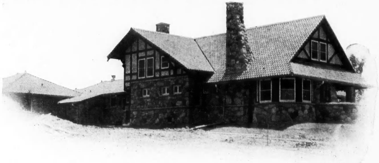
Striking Work With Field Stone on Residence of Mr. M. Ford, at Cedar Rapids. Chimney, Laid up by Frank Klepach, is especially good
