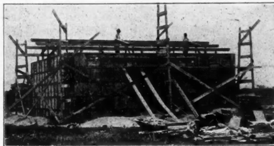
Building Being Erected by the One-Day Process
