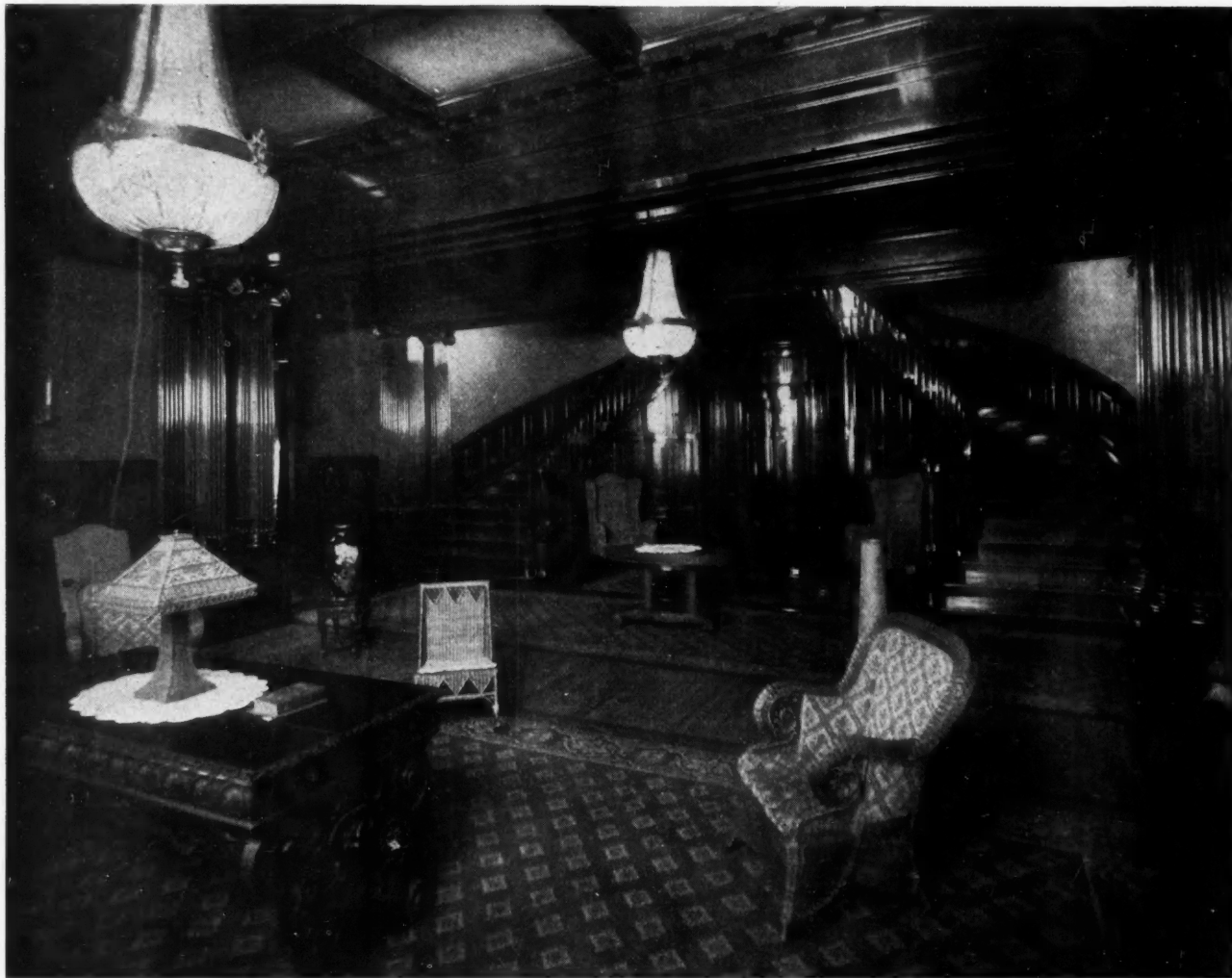
Main Hall and Stairway in Mitchell Residence, Finished in Quartered White Oak, Hand Rubbed
