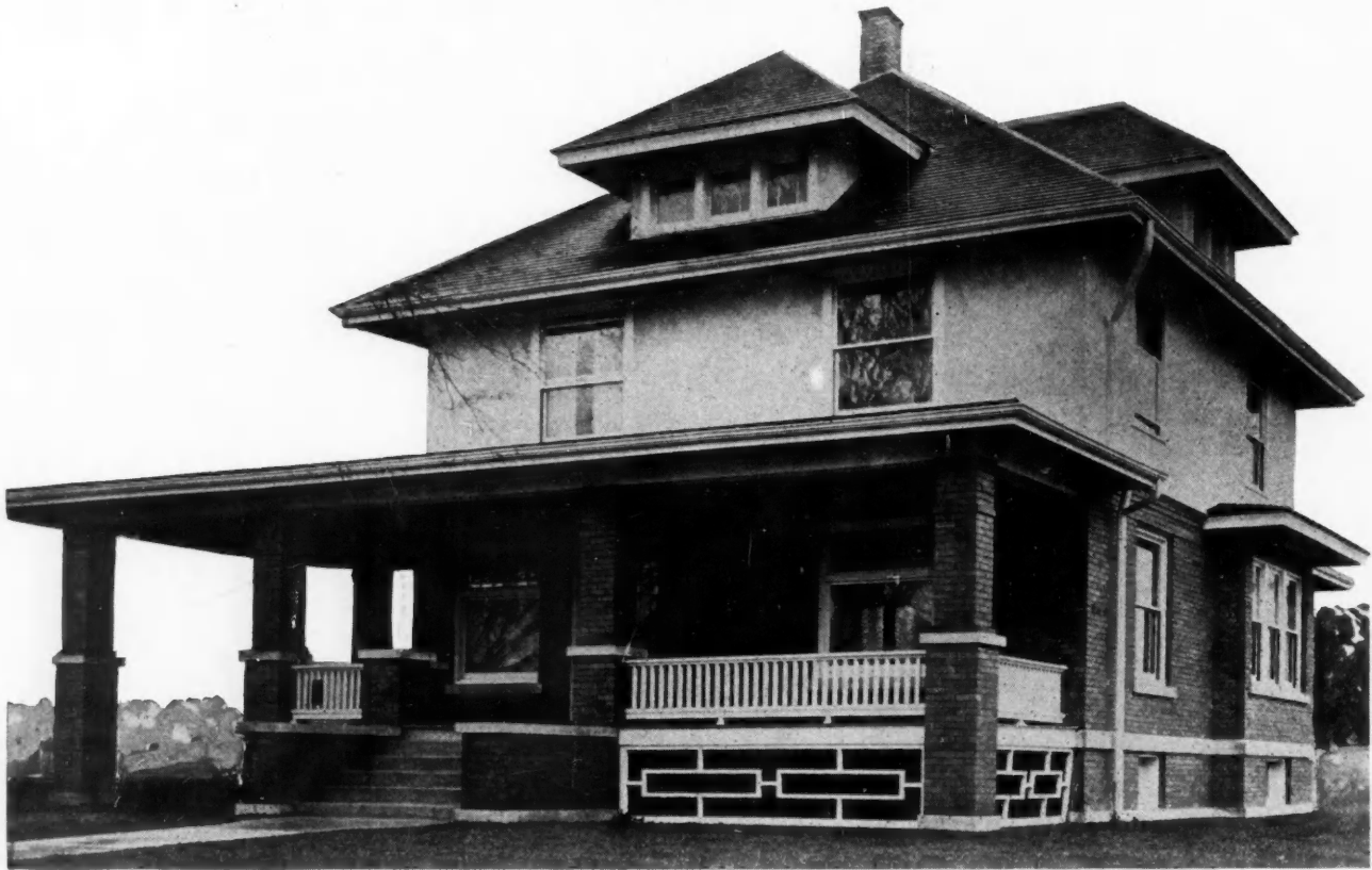
Another View of Builder Danielsen's 1st Prize Winner. He States He Is Designing and Building Many Such Residences in Davenport, that Growing City of 45,000 People
