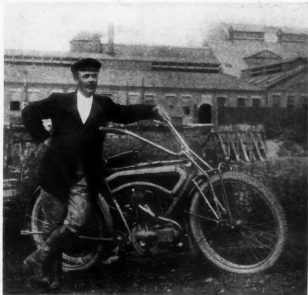
SUPERINTENDENT OF CONSTRUCTION USES MOTORCYCLE M. C. Schanck, Superintendent of the Street Department, Kings County Lighting Co., Brooklyn, N. Y. He finds the motorcycle a great time saver as well as an economical means of rapid transit.
