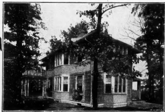
Residence of L. R. Hoff, Paterson, N. J. Roofed with J-M Transite Asbestos Shingles, Sided with J-M Stucco. F. J. Parsons, Architect, N. Y.
