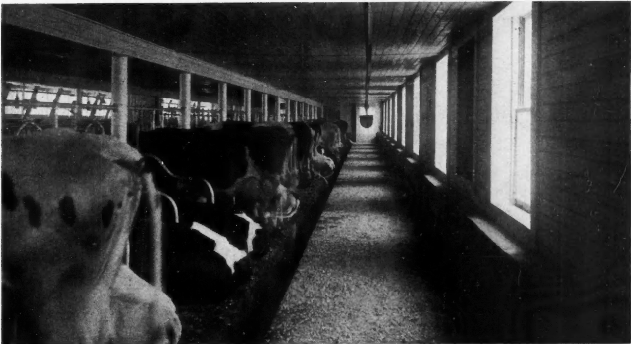
Interior View of Dairy Stable Section. Manure Carrier Runs on Overhead Track to All Parts; Sanitary Metal Stanchions Provided; Interior Tight Ceiled
