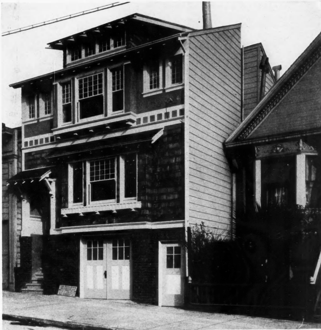
Clever Handling of a Hard Problem—An Attractive Dwelling on a Narrow Lot in a Closely Built Up City Street—Designed and Built by Edw. A. F. Carson, at San Francisco; Cost $4,000
