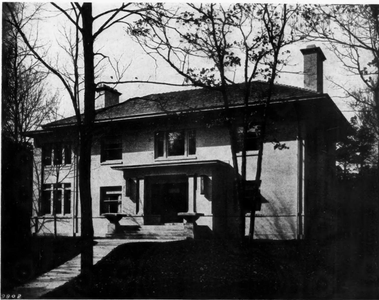
Residence of D. S. Pate (Geo. W. Maher, Architect), Highland Park, Chicago.
