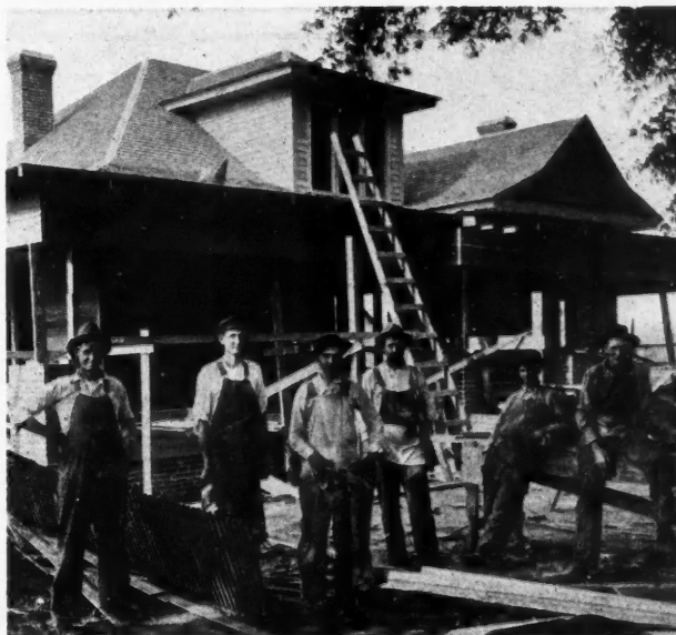
R. P. Finley and Crew Remodeling a Southern Cottage
