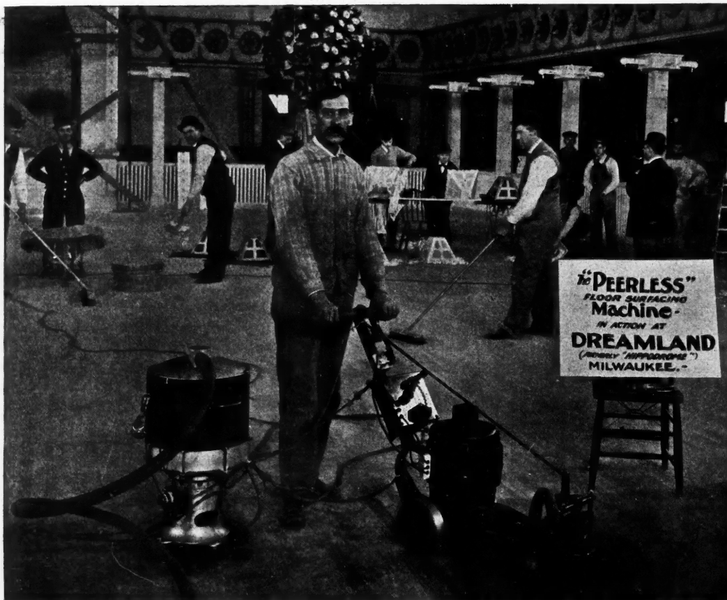
"Peerless" Floor Surfacer at Work
