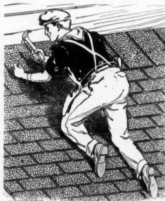
Shingles nailed on in the ordinary way.
