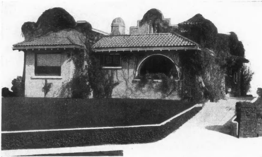
A Mission Type Bungalow of Five Rooms, Walled with Gravel-Coated Stucco; Cost Said to have been $3300.
