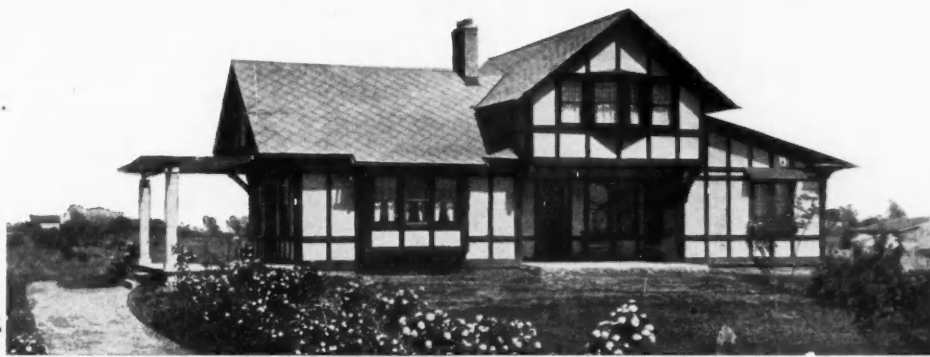
Bungalow of Albert E. Small, Amherst, N. Y. Sheathed Asbestos Building Lumber, and roofed with Asbestos "Century" Shingles by Robert Demest, Contractor, Williamsville, N. Y.
