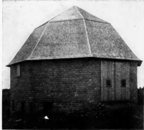
Concrete Block Barn of Unusual Design, Octagon with Gambrel Roof.
