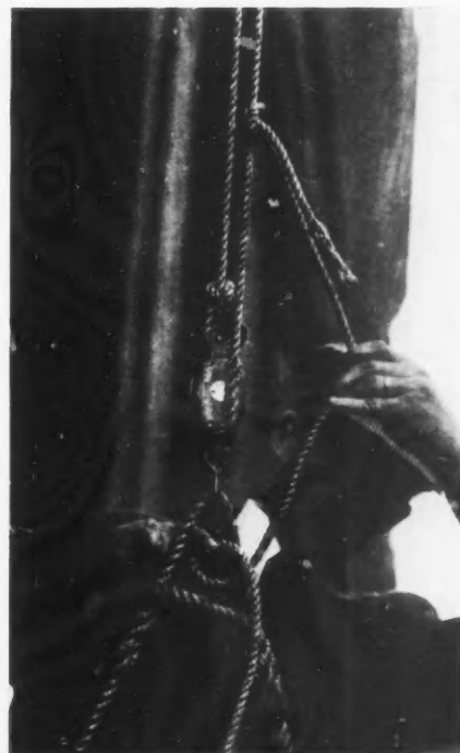
Fig. 5. Safety rope supporting all the weight; the workman easily forms a Blackwall knot and "ties up".
