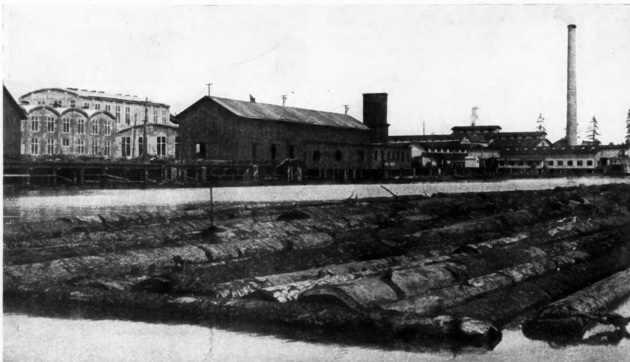
Huge Reinforced Concrete Paper Mill at Marshfield, Ore., the First Paper Mill in the U. S. to Utilize Saw Mill Waste for Paper Pulp Making.
