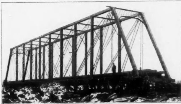
Large Steel Railroad Bridge Successfully Moved About 1,000 Feet on Railroad Trucks.
