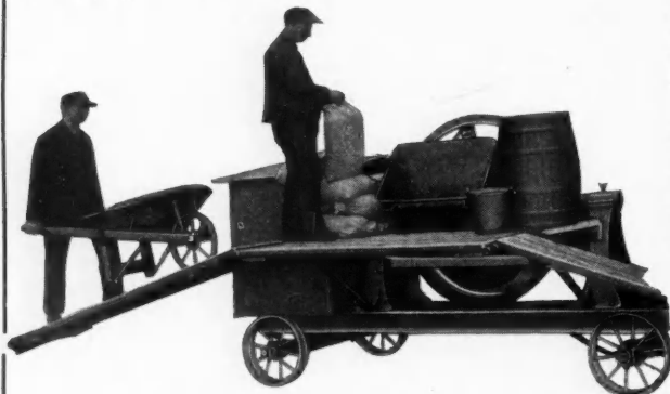
"Clover Leaf Mixer with Folding Loading Platform."
