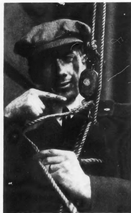
Fig. 1. Author seated in boatswain's chair, points at safety rope spliced to eye of block.
