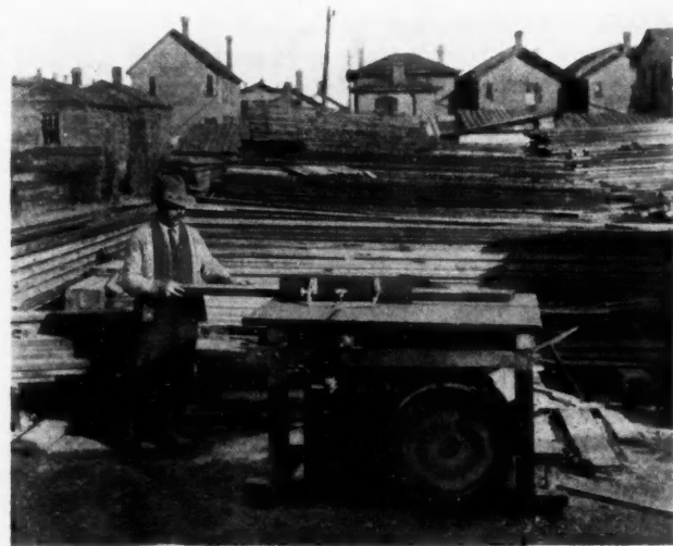
"Wonder" Saw Rig Working up Form Lumber.
