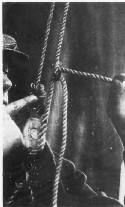
Fig. 4. Half-hitches tighten down and safety rope takes the weight.
