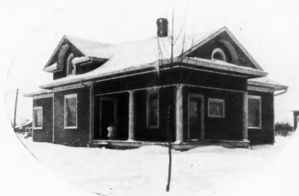
Neat Little Six-room Bungalow Designed and Built During Spare Time at Bluffton, Ind.
