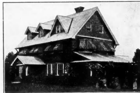
Residence of D. T. Dickson, Wayne, Pa., Covered with J-M Transite Asbestos Shingles. Francis Gogert, Wayne, Pa., Architect.
