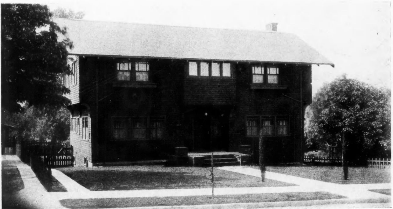
Eight-room Shingled Swiss Chalet Style Dwelling, Built for $4,500 at Pasadena, Calif.
