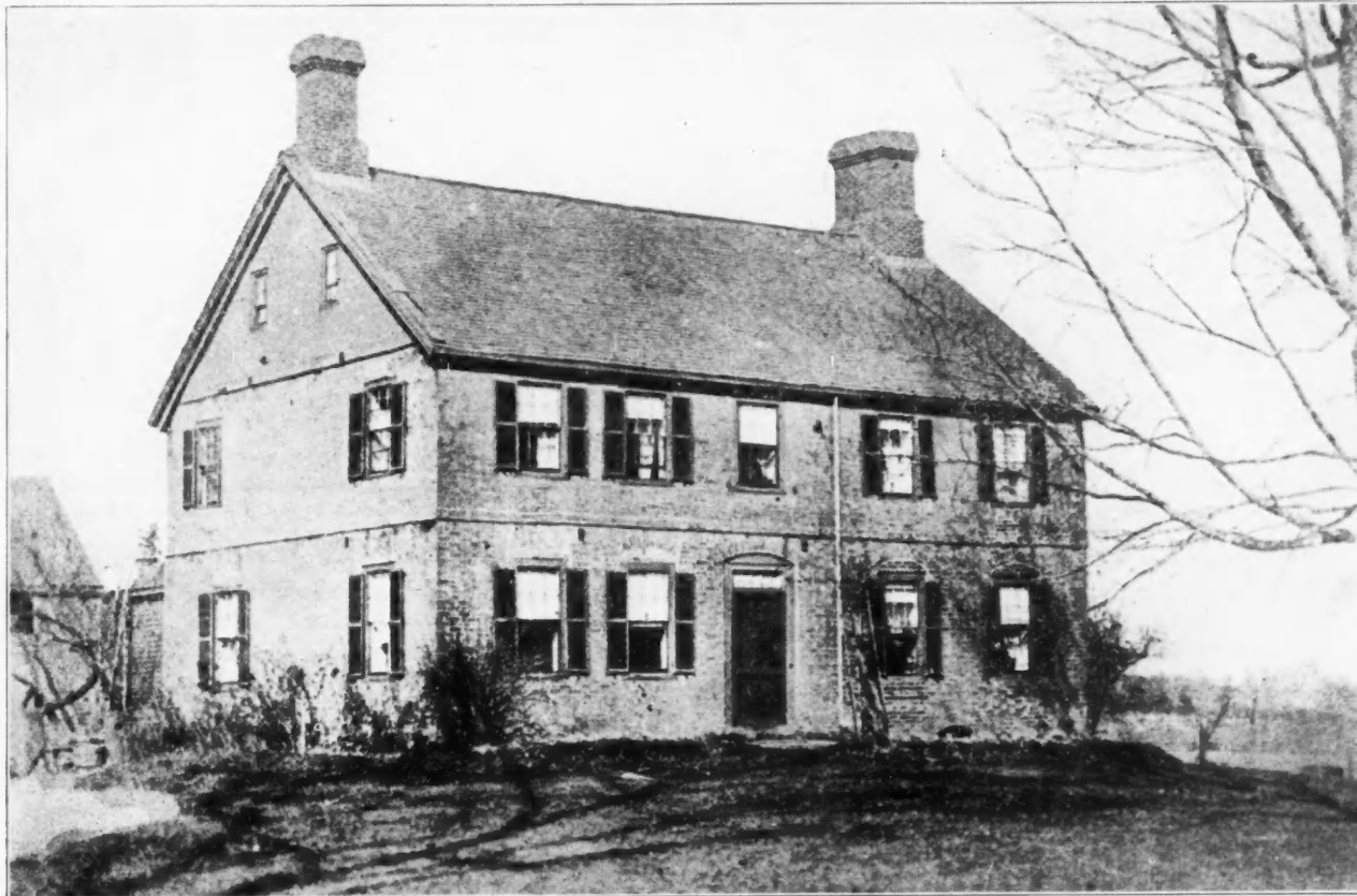
The old Weeks house at Greenland, N. H., the Oldest Brick House in New Hampshire, Built in 1638, and still in excellent state of repair.
