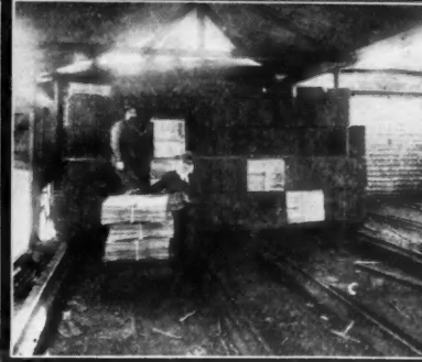
Shingles just out the kiln
