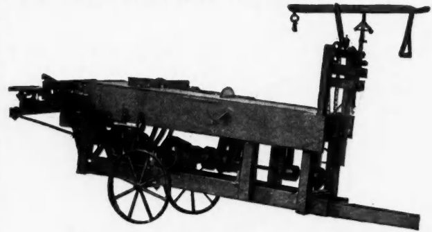
Side View of Henderson Portable Power Shop.
