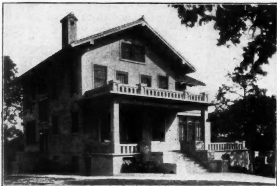
Residence of C. A. Mangold. Oak Cliff, Dallas, Tex. Stucco on RIB LATH.
