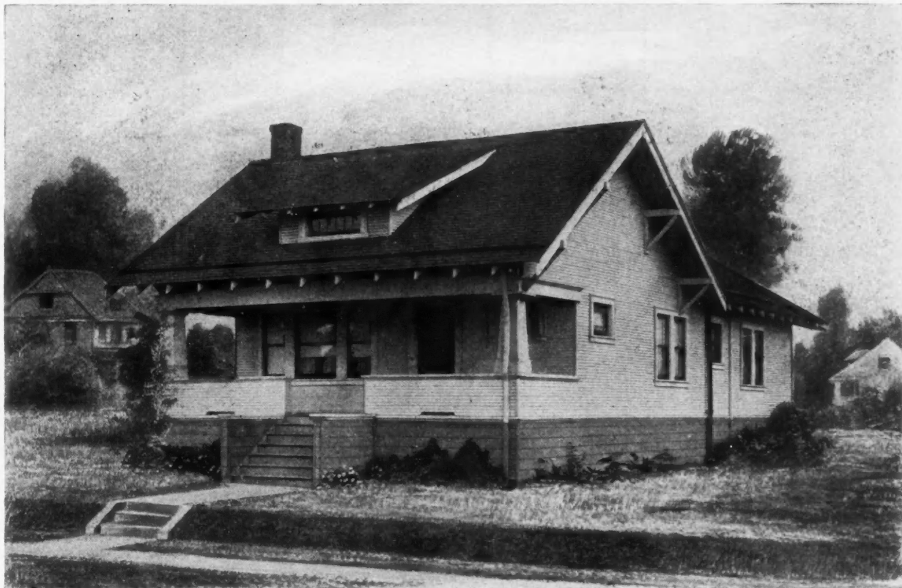
Gable End Cottage house of five rooms. Size 27 feet 6 inches by 37 feet 6 inches. We can furnish complete set of blue-printed working plans and typewritten specifications for only $6.00 per set. Blue-prints consist of basement plan; roof plan; main floor plan; front, rear, two side elevations; wall sections; and all necessary interior details. Specifications consist of twenty-two pages of typewritten matter. When ordering, ask for Design No. 6669.
