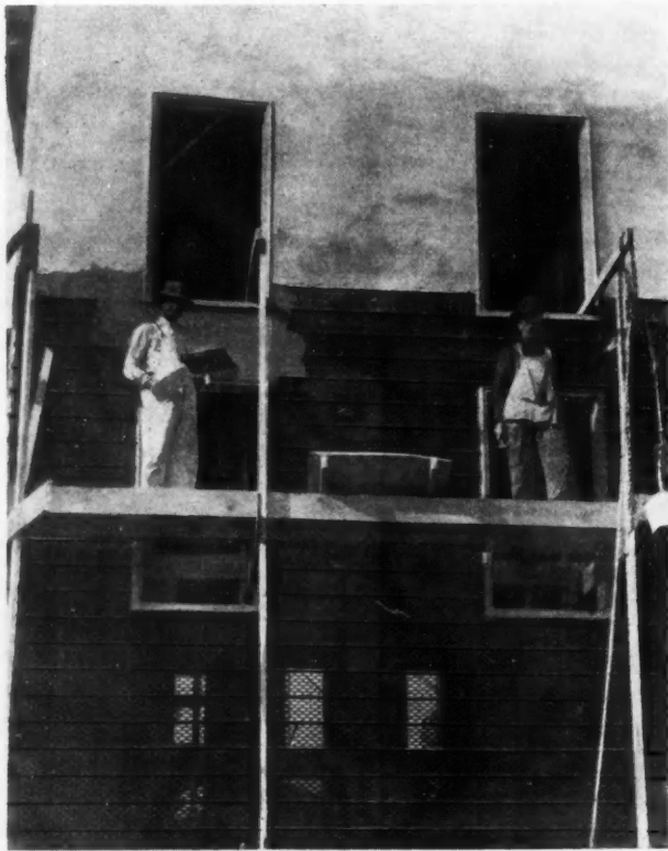
The Workmen Like Metal Lath Because It Presents such a Fine Plastering Surface. Photo shows Bostwick's "Truss Loop" Lath.
