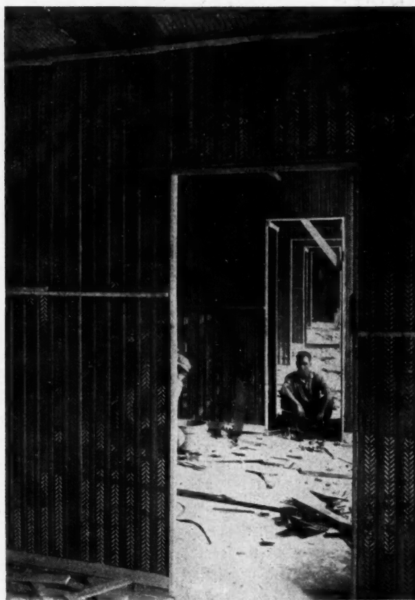
"Keyridge" Metal Lath and Stud Combined as Furnished by Edwards Mfg. Co. Used in New Hotel Metropole, Cincinnati.
