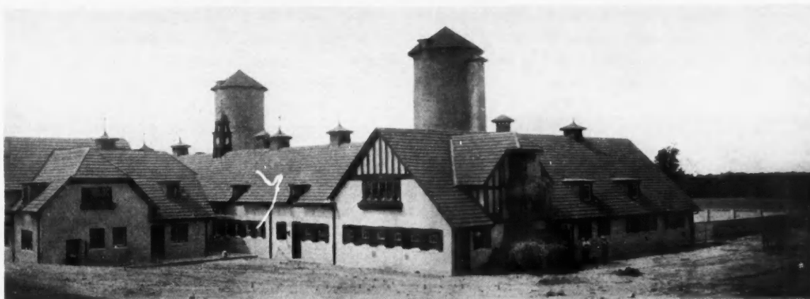
Notable Buildings on Farm of James Couzens, Bloomfield Township, Mich. Trussed Concrete Steel Co.'s "Hy-Rib" Used to Reinforce Silos, Fences, Partitions, etc. Albert Kahn, Arch., Ernest Wilby, Associate.
