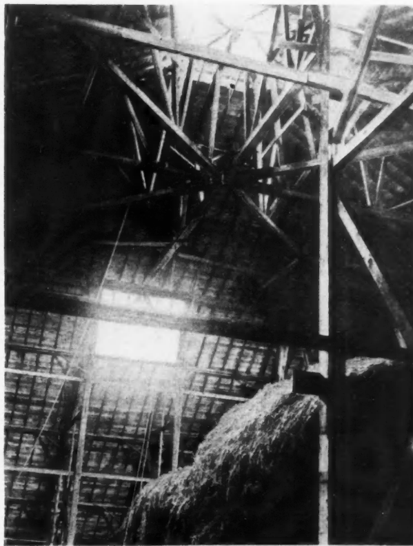
Interior Photo Showing Framing Underneath the Cupola.
