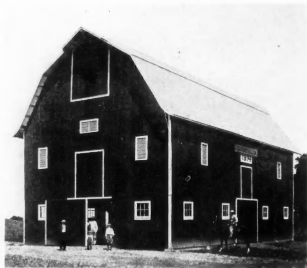
Anderson Barn Completed.
