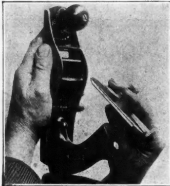
Plane Has Instant Setting Screw.
