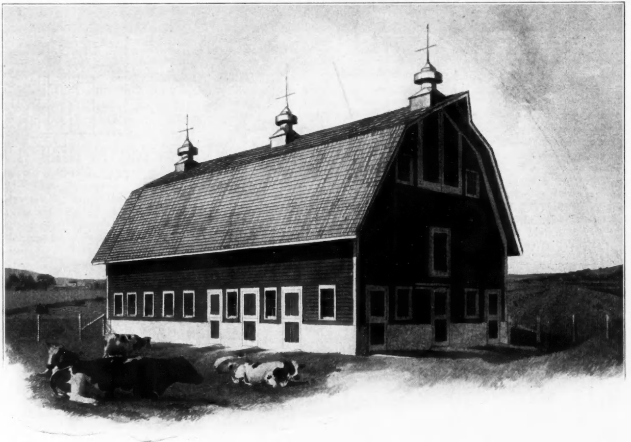
A modern gambrel-roof barn for 22 cows and 6 horses, besides three large box stalls. Cows are stanchioned in two rows, facing in. Size of barn 74 by 36 feet. We can furnish complete set of blue-printed working plans and type-written specifications for only $8.00 per set. When ordering, ask for Design No. A284.
