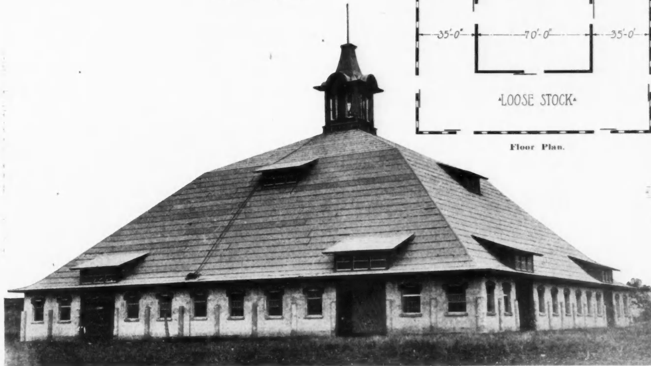
Unusual Type of Stock Barn. 140 Feet Square, Built at Geneva, Ill., by Fred Hillquist, the local contractor. His carpenters worked 1 year on this job.
