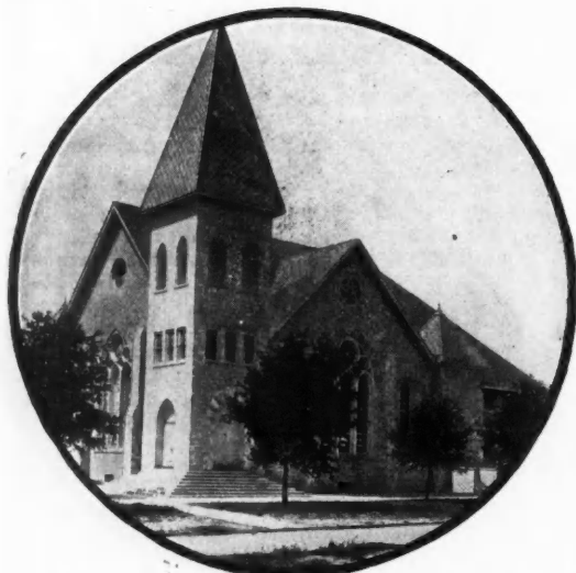
First Congregational Church, St. Petersburg, Fla., covered with J-M Transite Asbestos Shingles.
