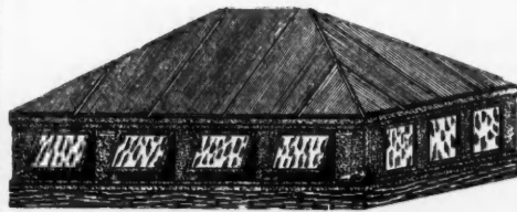
One of the Galesburg Skylights.
