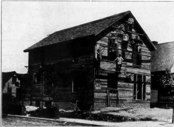
PORCH BUILDER'S AND PLASTERER'S TRESTLE
