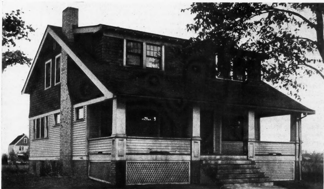
Front View of $4,000 Residence of Chas. K. Turney. Note the Dormer Windows that Promise Bright, Cheery Bedrooms.
