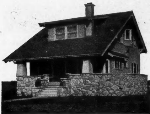
Residence of C. A. Gormley, Kansas City, Mo. Covered with J-M Transite Asbestos Shingles
