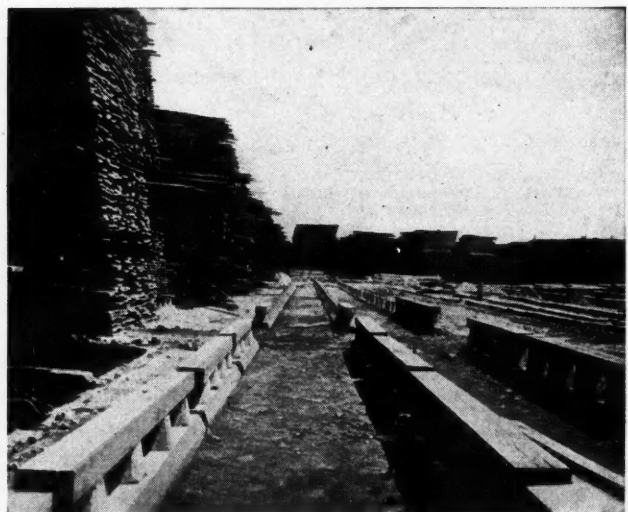
View of Lumber Yard Near Toronto, Showing Concrete Pile Supports.
