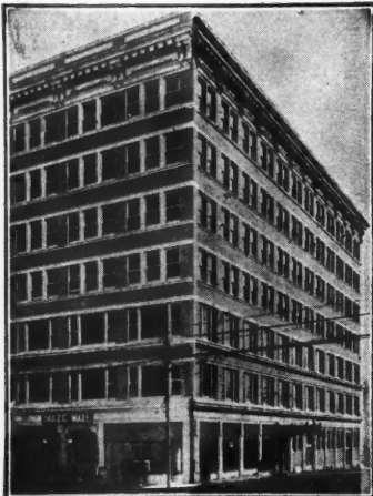
Kling Building, Kansas City, Mo. Sanneman & Goold, Architects Berger's Metal Lumber Used On 20-Ft. Spans
