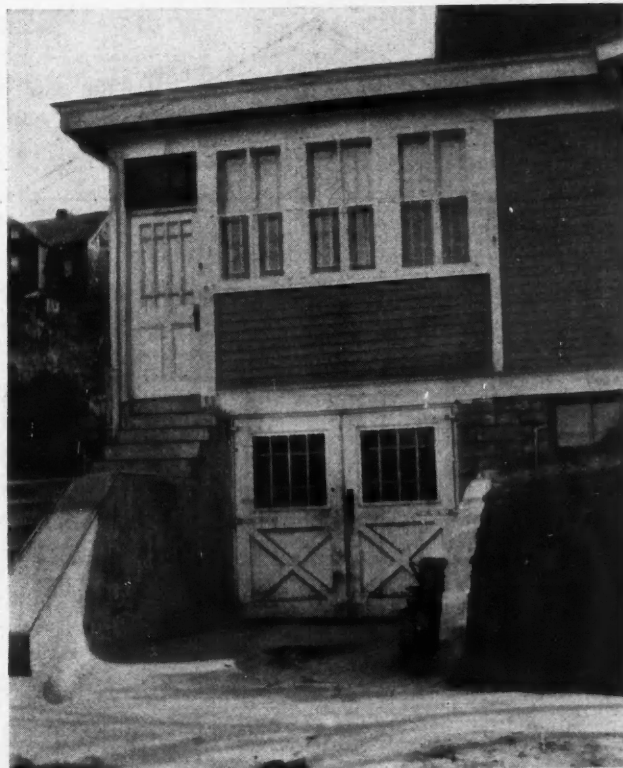
Garage in Cellar of Corner Lot House.
