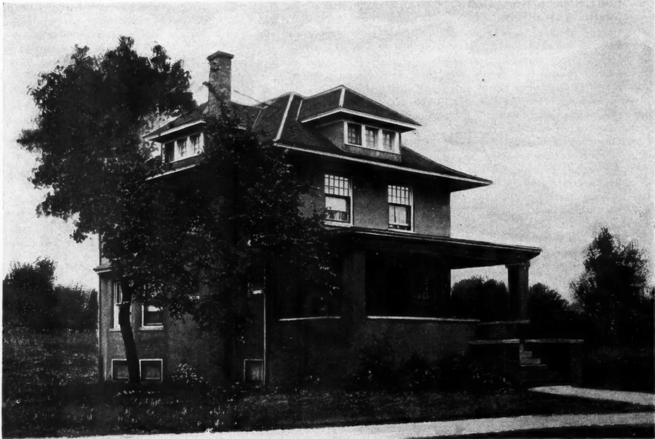
Square, hip-roof cement stucco house of eight rooms. Size, 27 ft. 6 in. by 30 ft. 6 in. We can furnish complete set of blueprinted working plans and typewritten specifications for only $7.00 per set. Blueprints consist of basement plan; roof plan; first and second floor plans; front, rear, two side elevations; wall sections; and all necessary interior details. Specifications consist of twenty-two pages of typewritten matter. When ordering, ask for Design No. 6723.
