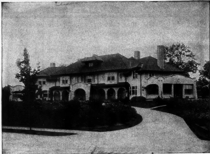
A House at Chestnut Hill, Mass. Chapman & Frazer, Architects. Clinton Wire Lath Used.
