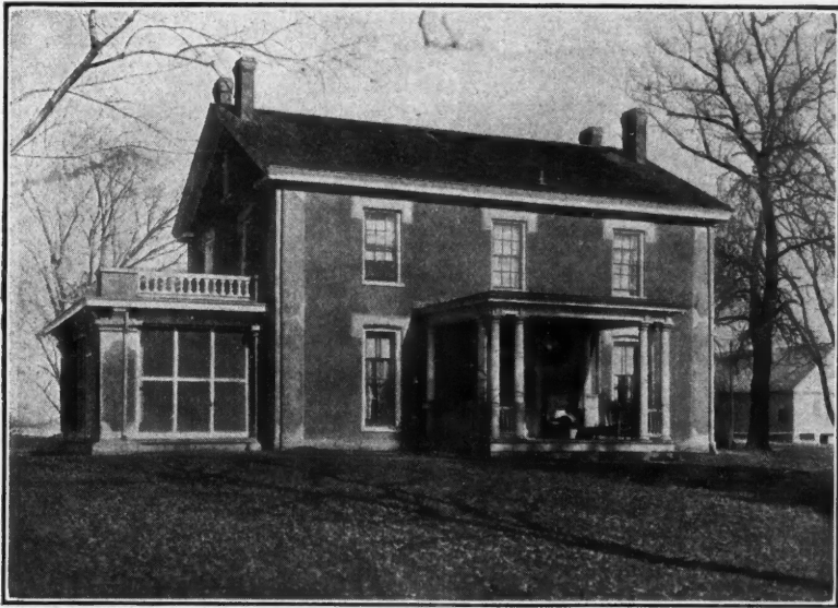
A Brick House Built at State College, Ames, Iowa, in 1862. Becoming Dilapidated, it was Restored with Stucco, as Shown.
