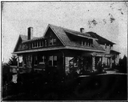
Residence of J. A. Curry, Portland, Ore. Covered with J-M Transite Asbestos Shingles
