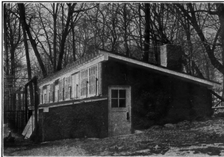
A Poultry House with Stucco Finish. This Attractive Structure Illustrates the Adaptability of Stucco to Farm Buildings.
