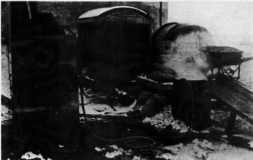
Heating the Water by Steam From a Boiler.
