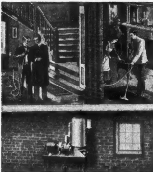
Thurman No. 2 Electric-Driven Stationary Vacuum Cleaner Installed in Basement of a Residence. The machine is started by pushing electric button on each floor. These machines are made in all sizes.
