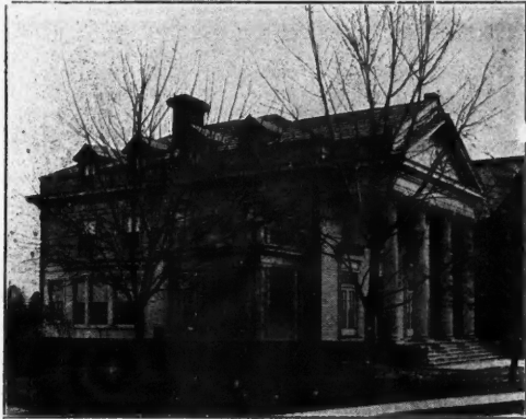
Residence of G. U. Tompers, Brooklyn, N. Y. A. D. Isham, Arch., New York City Covered with J-M Transite Asbestos Shingles
