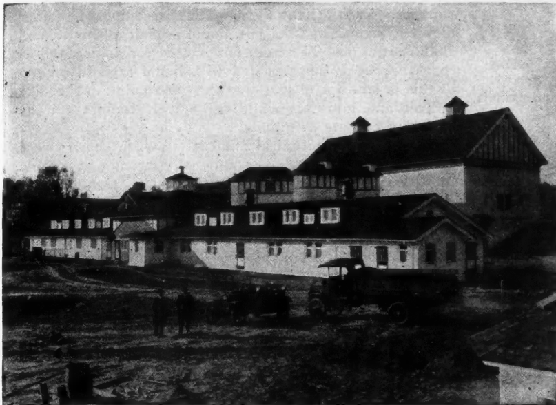
Delchester Farms, Malvern, Pa. Contractor: Jacob Myers & Son, Philadelphia
