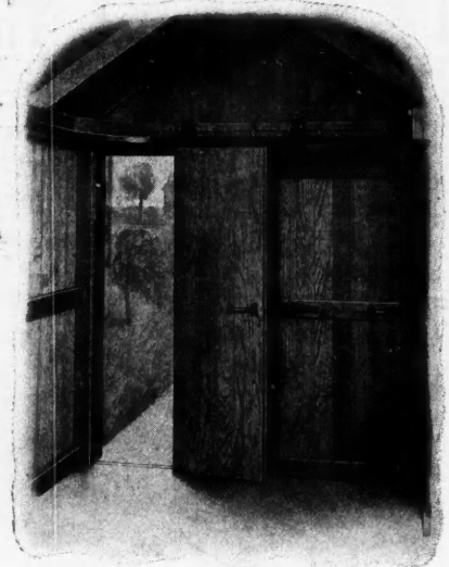
When You Want to Enter the Garage, it is Necessary to Open Only One Section of the Door.
