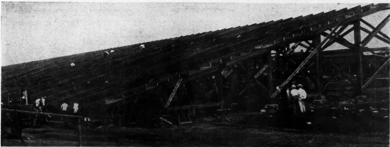
Bleachers of Wood Construction on Back Stretch Sheepshead Bay Speedway.
