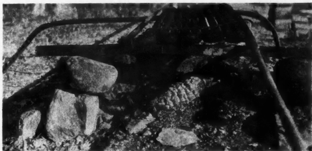
Heater Coil Over Open Fire for Heating Mixing Water.
