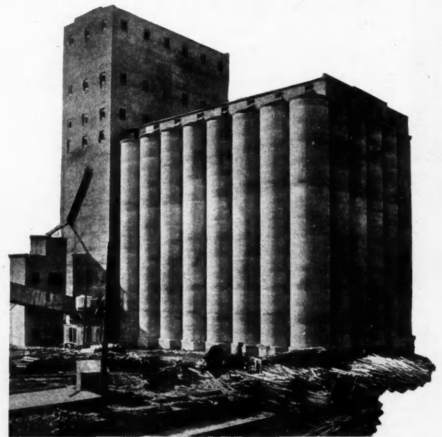
Large Concrete Grain Elevator of the Southern Pacific R. R. at Galveston, Texas. Passed Thru Recent Hurricane Unharmful. Construction Completed June, 1915, by James Stewart & Co., Builders; 22,000 Barrels of "Alpha" Cement Used.
