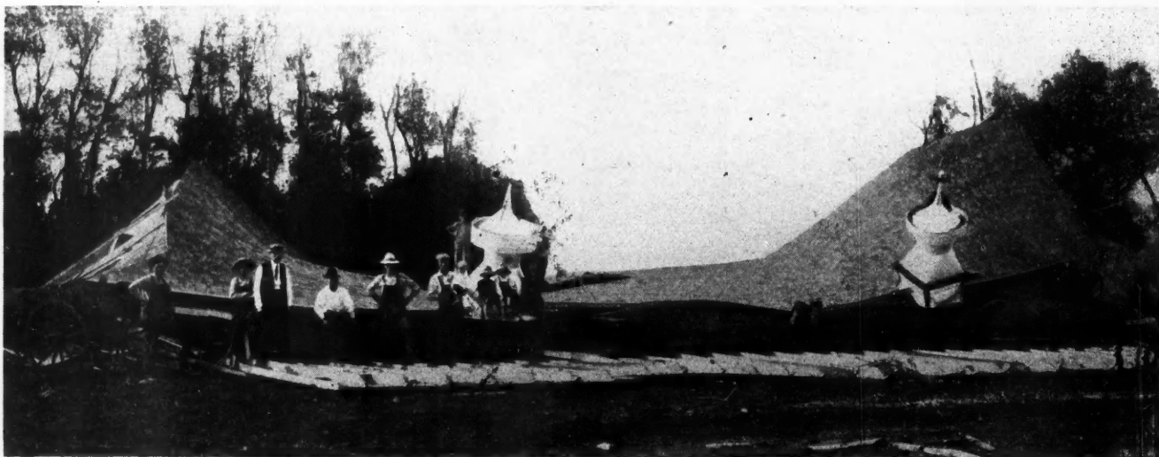
The Only Part of This Barn to Weather the Tornado Was the Metal Ventilators—They Will be Used Again Without Repair.
