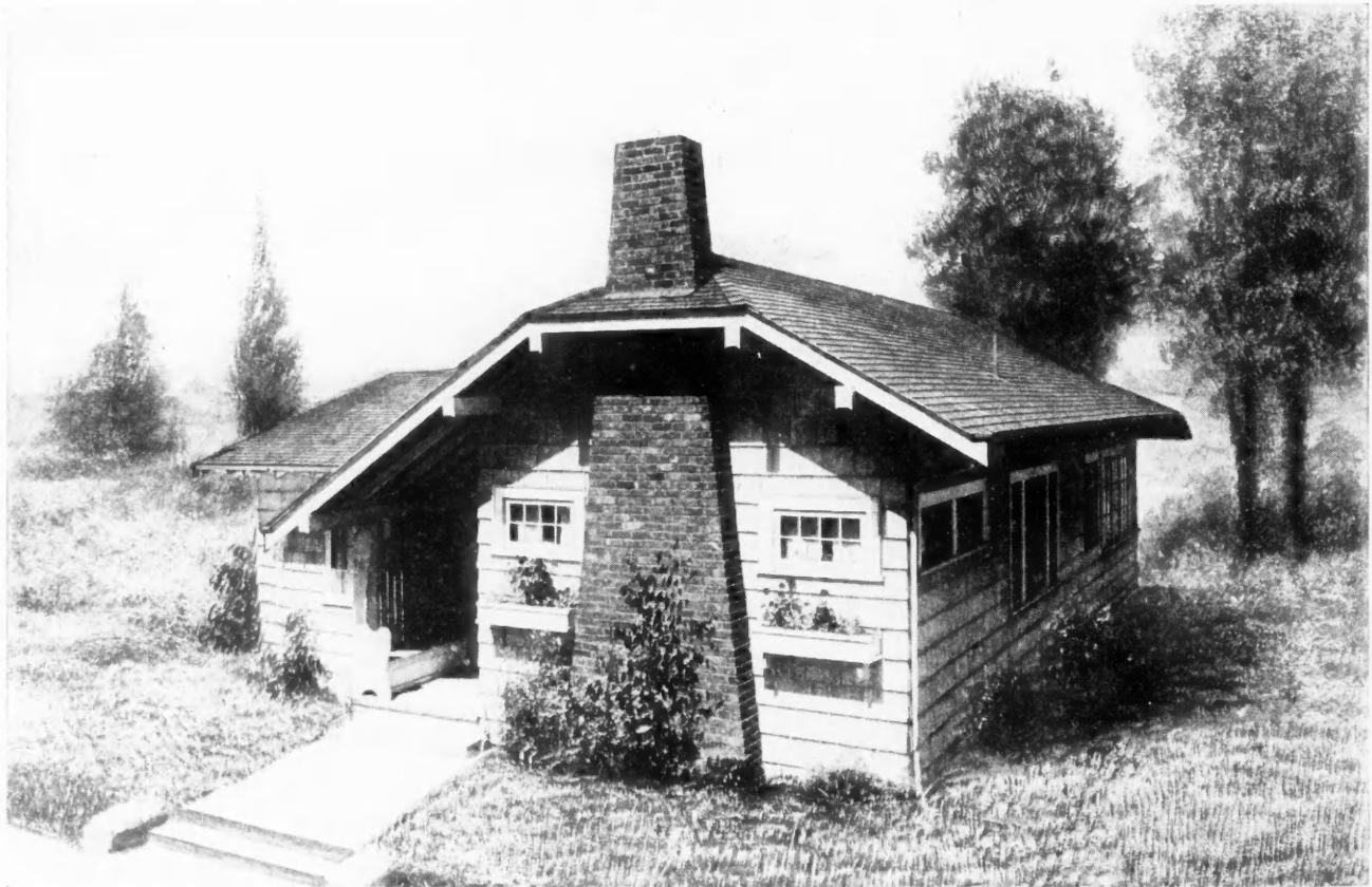
Plan "A," Size 24 by 36 feet, Four Rooms. Plan "B," Size 28 by 40 feet, Five Rooms.
