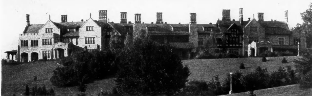
EAST AND WEST HILL, RESIDENCES OF WM. L. GLATFELTER AND PHILIP H. GLATFELTER, SPRING GROVE, PA. J. A. Dempwolf, Architect
