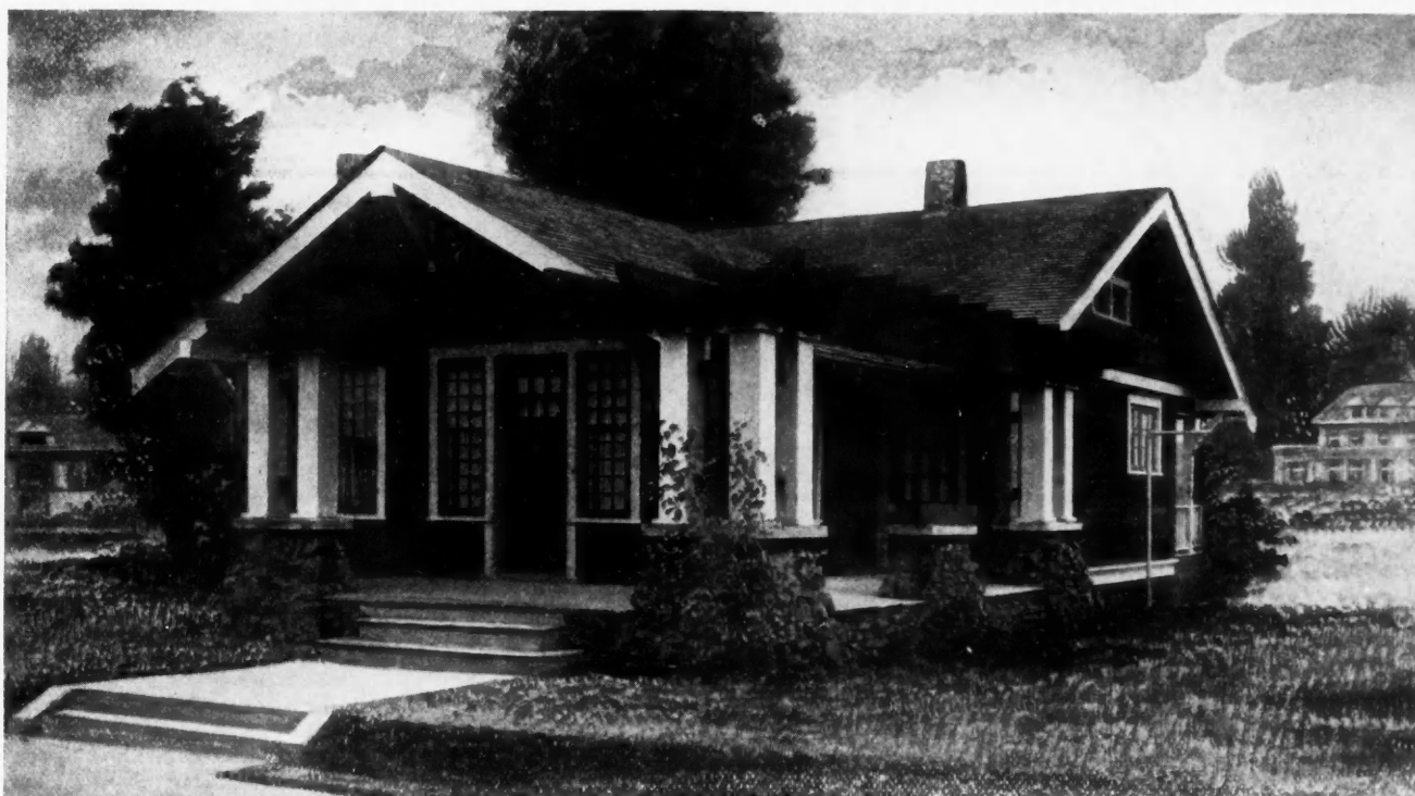
Well-arranged bungalow of four rooms. Size, 27 feet 6 inches by 36 feet. We can furnish complete set of blue-printed working plans and typewritten specifications for only $6.00 per set. Blueprints consist of basement plan; roof plan; main floor plan; front, rear, two side elevations; wall sections; and all necessary interior details. Specifications consist of twenty-two pages of typewritten matter. When ordering, ask for Design No. 6769.
