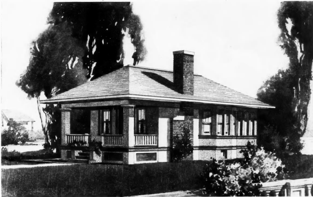
The Five-Rooms-in-Three Bungalow. Design No. 6815. Planned for Modern Efficiency in Sleeping Arrangements. This Bungalow Measures Only About 20 by 35 Feet and Makes a Snug, Satisfactory Home.
