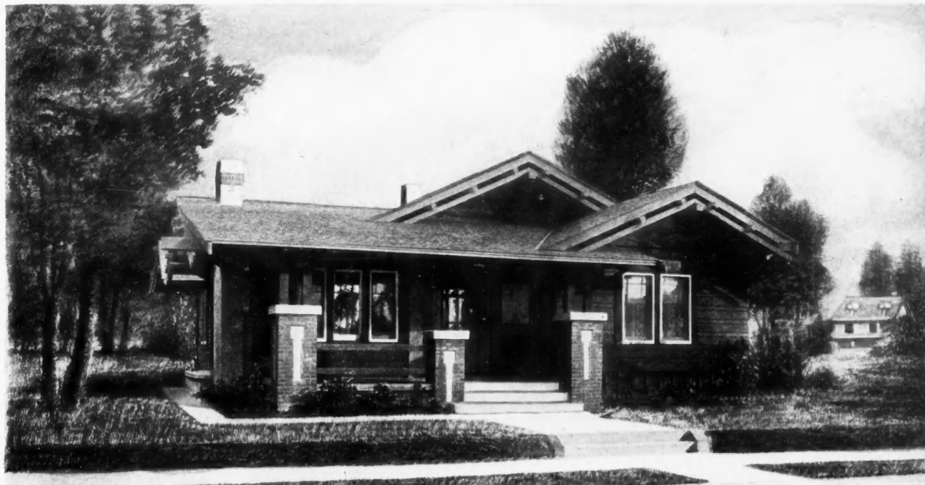
Five-room bungalow with distinctive roof construction. Size, 31 by 44 feet. We can furnish complete set of blueprinted working plans and typewritten specifications for only $7.00 per set. Blueprints consist of basement plan; roof plan; main floor plan; front, rear, two side elevations; wall sections; and all necessary interior details. Specifications consist of twenty-two pages of typewritten matter. When ordering, ask for Design No. 6759.
