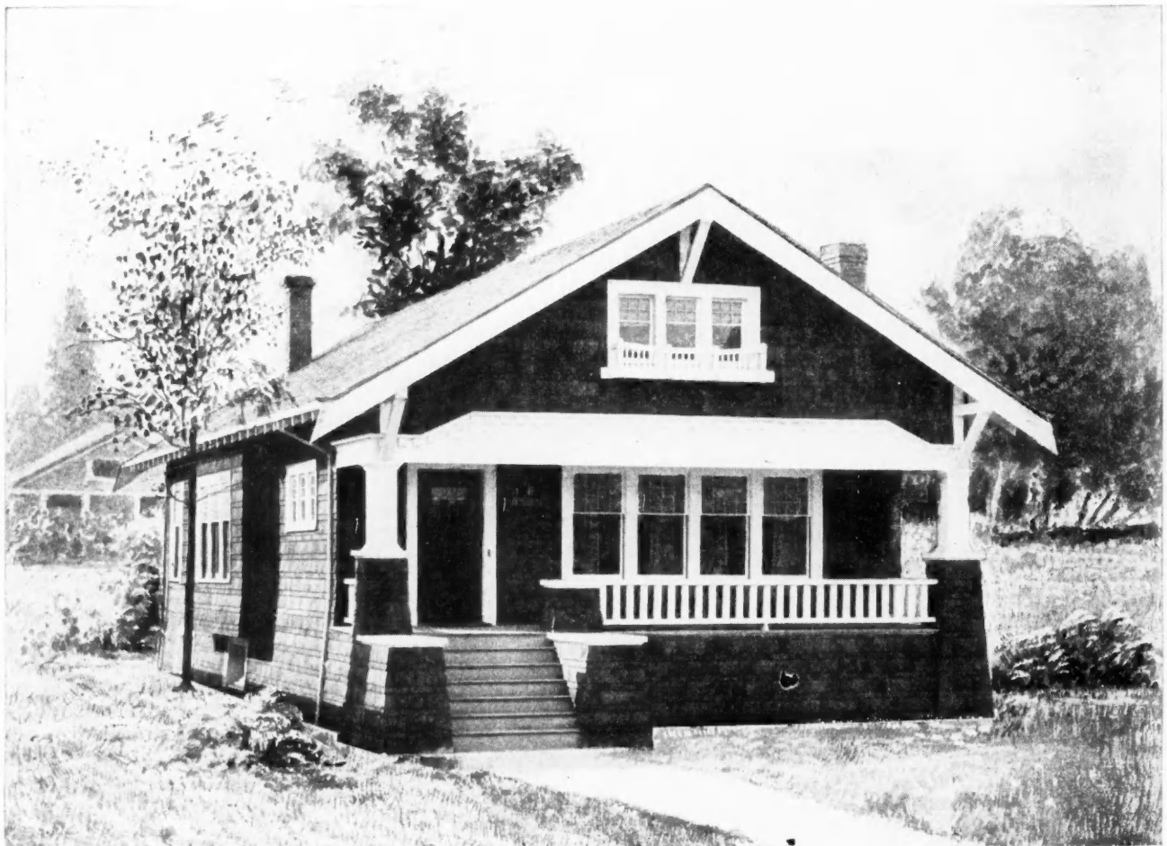
Six-Room Bungalow Featuring Space and Labor-Saving "Pantryette." Design No. 6630. A Thorough Practical Design. Size, 26 by 35 Feet. Space is Saved and the Kitchen Work Facilitated by Doing Away with the Pantry and Providing a Large Built-in Kitchen Cabinet in Its Place.
