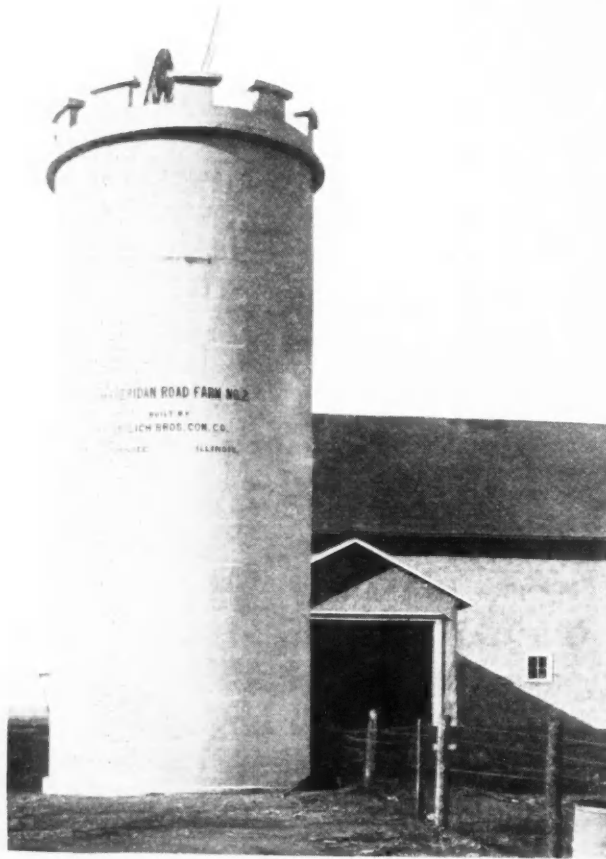
Poured Concrete Water Tank, Size 12 by 30 Ft., Capacity 27,000 Gals. Standing on Farm Just North of Chicago.
