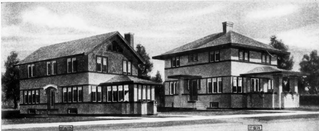
Perspective View of Designs No. 6773 and No. 6774. Both Houses are Finished in Cement Stucco Trimmed with Dark Stained Woodwork. Plans and Specifications for Either of These Designs Can be Furnished for $8.00 per set. No. 6773 Has Four Rooms on the Second Floor and Three on the First, and No. 6774 Has Three on Each Floor. A Feature of Each Design is the Large Living Room with the Adjoining Porch.
