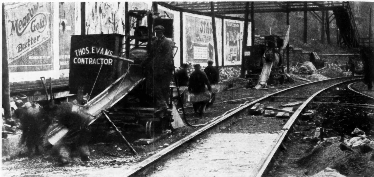
Two Ideal Cincinnati Tractor Paving Mixers at work on Colerain Ave., Cincinnati, Ohio, since May, 1915. These mixers were adopted because of their compact construction and because they prevented the tying up of the trolley service on that busy thoroughfare.
