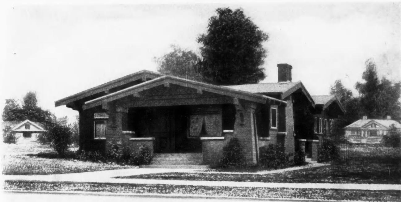
Well arranged bungalow of five rooms. Size, 28 feet by 39 feet 6 inches. We can furnish complete set of blue-printed working plans and typewritten specifications for only \$6.00 per set. Blueprints consist of basement plan; roof plan; main floor plan; front, rear, two side elevations; wall sections; and all necessary interior details. Specifications consist of twenty-two pages of typewritten matter. When ordering, ask for Design No. 6758.
