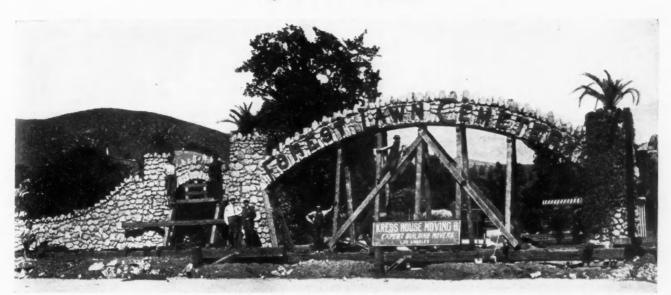
Fig. 1. An Unusual Moving Job at Los Angeles. Span of Stone Arch is 38 Feet.
