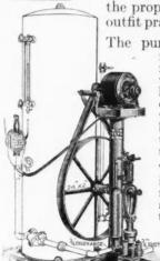
The pump tank and motor are mounted complete on one base, making the entire equipment very easy to install. The pumps have an air compressor and the discharge carries both air and water to the tank. The air after having been compressed in the top of the tank drives the water through the distributing lines.
