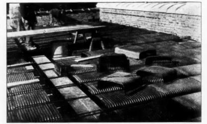
Method Used in Placing Pressed Steel Cores in Concrete Floor Construction.
