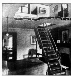
Installation of the Bessler Movable Stairway.
