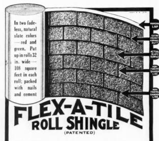
WE had in mind, when we designed this new Flex-A-Tile Roll Shingle, the growing demand for asphalt shingle roofs that would cost little to lay. How nicely we have accomplished this economy is surprising—this full size, 32-inch wide roll of asphalt shingles takes no more labor to apply than ordinary roll roofing.
