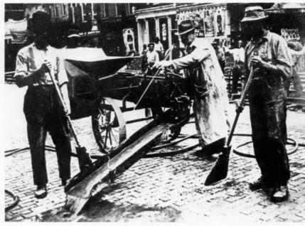
This Machine May be Used in Paving Work as An Auxiliary Mixer for the Grouting
