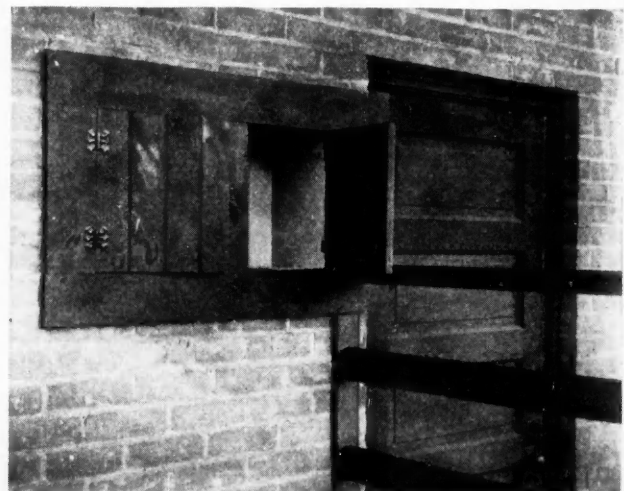
Fig. 2. Box for Sliding Cupboard Which May be Drawn up to the Second Floor.
