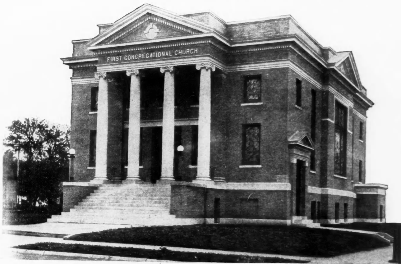
The First Congregational Church at Beatrice, Neb., Which is Built of Gray Face Brick with White Cement Stone for Trimmings.
