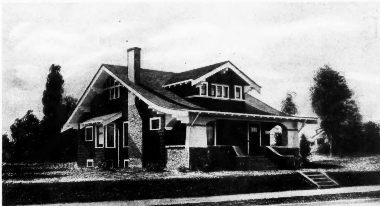
Seven-room home with many special features. Size, 26 feet by 41 feet. We can furnish complete set of blue-printed working plans and typewritten specifications for only $10.00 per set. Blueprints consist of basement plan; first and second floor plans; front, rear, two side elevations; wall sections; and all necessary interior details. Specifications consist of twenty-two pages of typewritten matter. When ordering, ask for Design No. 6803.
