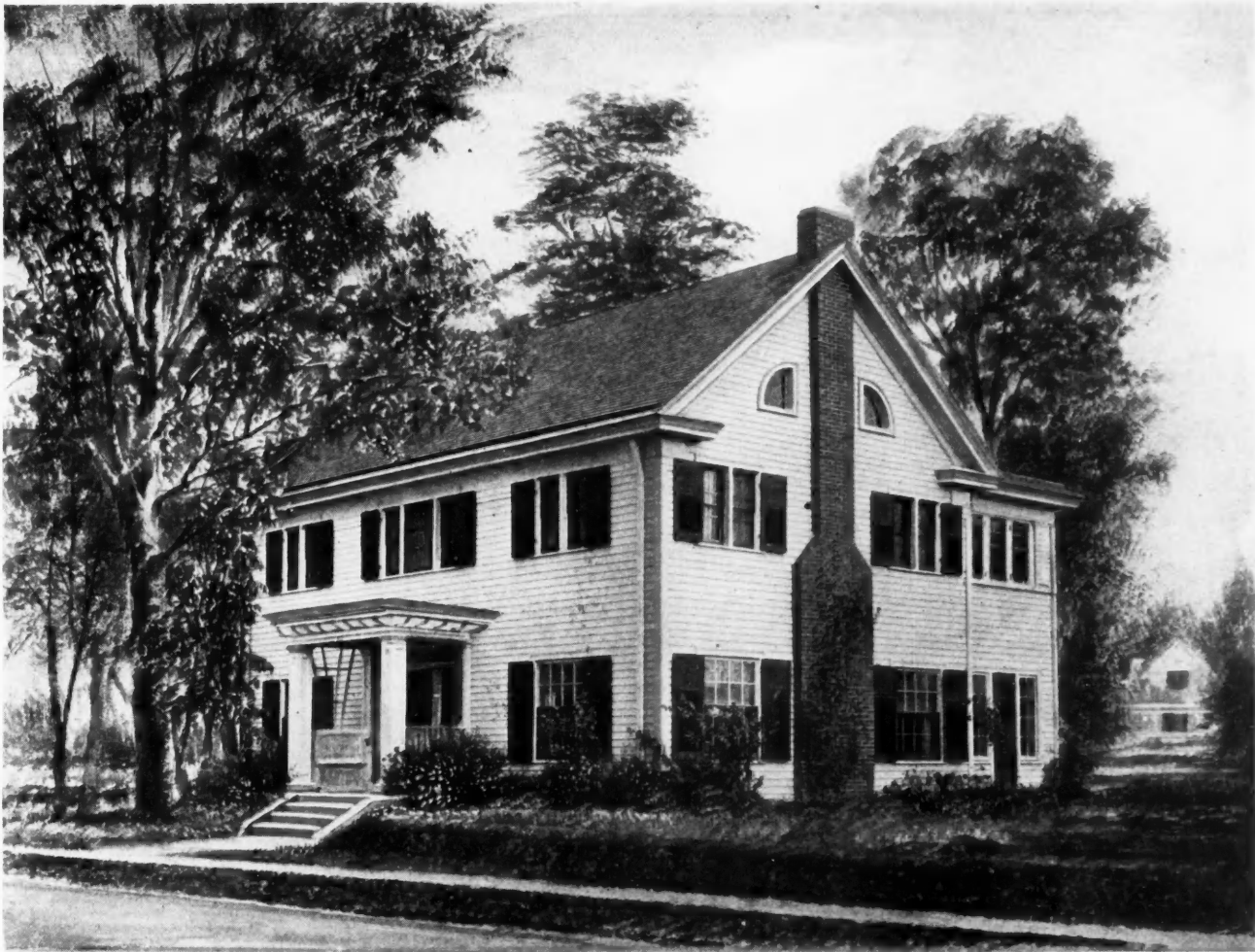
Comfortable Eight-room Home. Size, 37 feet by 32 feet 6 inches. We can furnish complete set of blueprinted working plans and typewritten specifications for only $12.00 per set. Blueprints consist of basement plan; roof plan; first and second floor plans; front, rear, two side elevations; wall sections; and all necessary interior details. Specifications consist of twenty-two pages of typewritten matter. When ordering, ask for Design No. 6826.
