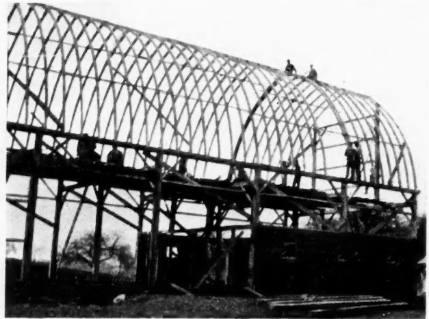
Mr. Hahn calls this a "Horse Shoe" Roof; But if the Two Curves Come Together at an Angle at the Peak as it Seems in the Photo, it Should be Called a "Gothic" Roof.
