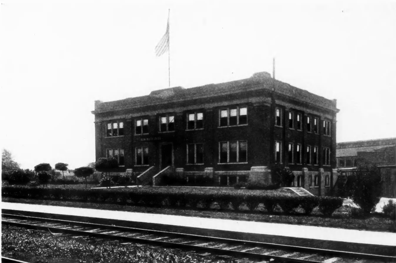
Factory Office Building of the Illinois Glass Co., at Alton, Ill.
