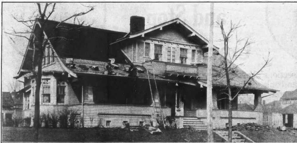
A home in Waterloo, Iowa, less than five years old, originally roofed with wooden shingles, now being roofed with Winthrop Tapered Asphalt Shingles
