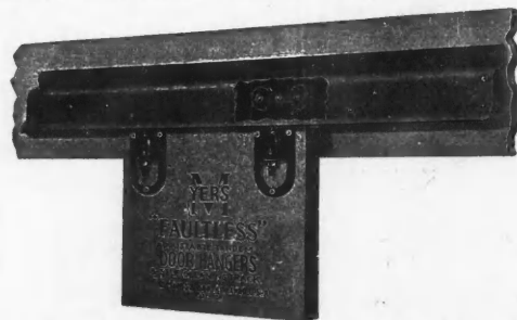
View of Barn Door Hung on Myers "Faultless" Door Hanger.
