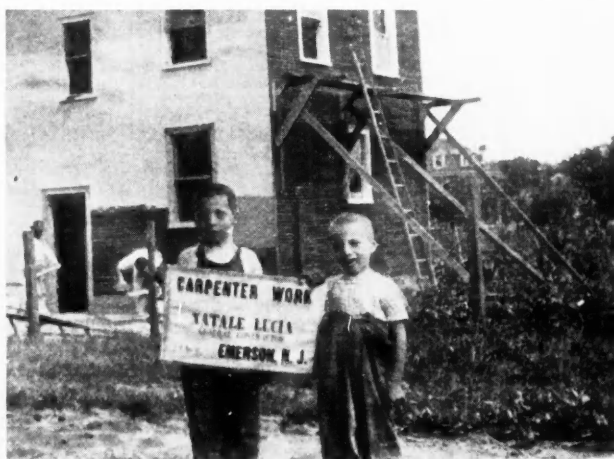
In the Background are Shown Three Braced Scaffold Brackets.
