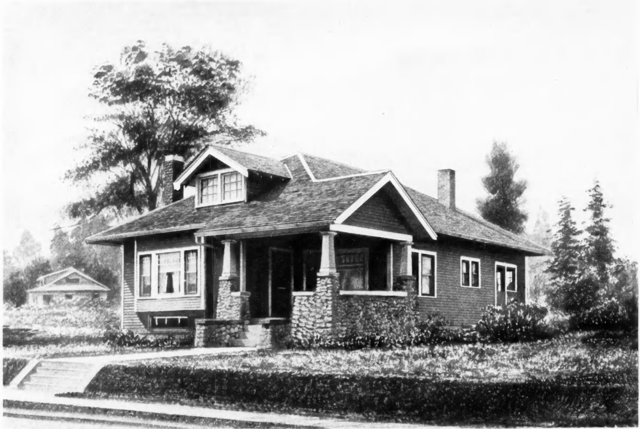
Attractive Five-room Home. Size, 24 feet by 40 feet. We can furnish complete set of blueprinted working plans and typewritten specifications for only $6.00 per set. Blueprints consist of basement plan; roof plan; main floor plan; front, rear, two side elevations; wall sections, and all necessary interior details. Specifications consist of twenty-two pages of typewritten matter. When ordering, ask for Design No. 6830.
