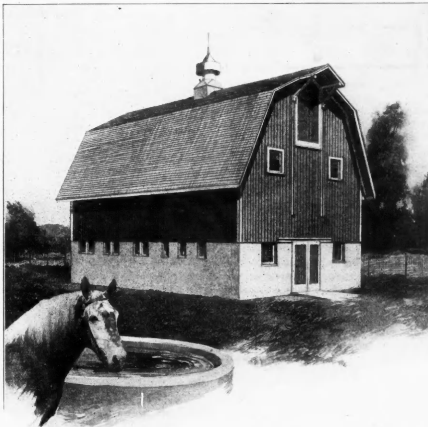
Horse barn with concrete basement and high gambrel roof. Size, 50 by 32 feet. We can furnish complete set of blueprinted working plans and type-written specifications for only $7.00 per set. When ordering, ask for Design No. A310.
