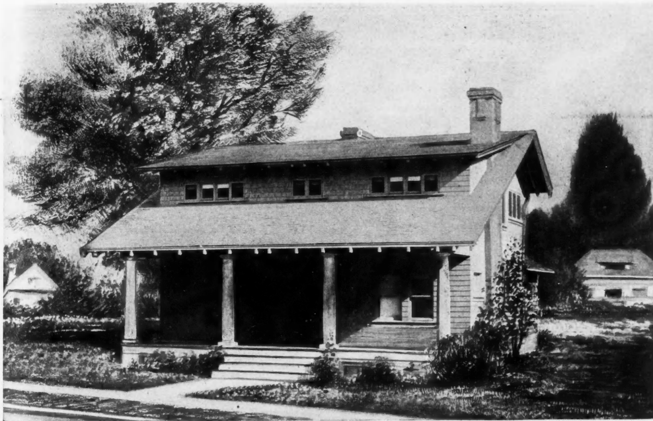
Comfortable Colonial Family House. Size, 28 feet by 41 feet. We can furnish complete set of blueprinted working plans and typewritten specifications for only $10.00 per set. Blueprints consist of basement plan; roof plan; first and second floor plans; front, rear, two side elevations; wall sections; and all necessary interior details. Specifications consist of twenty-two pages of typewritten matter. When ordering, ask for Design No. 6854.
