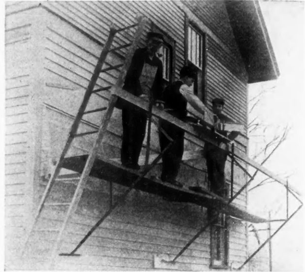
Showing the Guard Rail with Tool Shelf Using "Safety First" Brackets.
