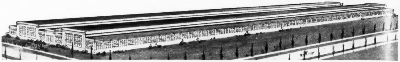
Fireproof Single Story Factory Building of Domestic Engineering Company.
