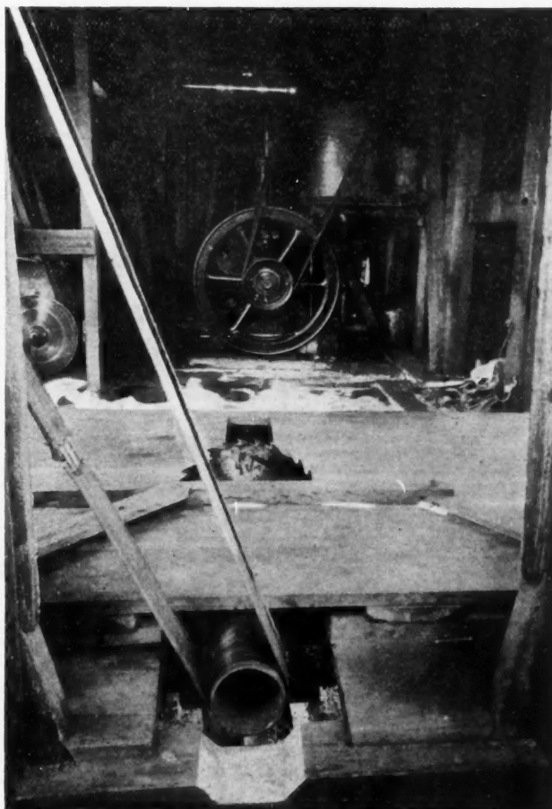
Inside the Brown Portable Power Shop.
