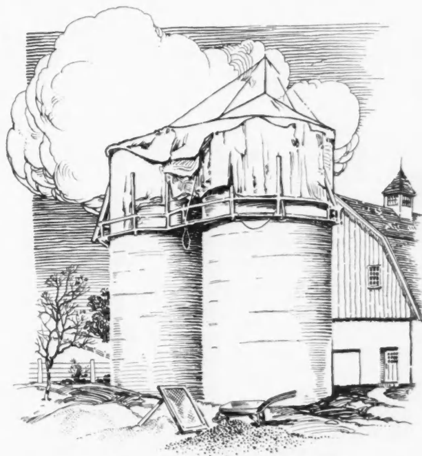
Fig. 5. Protecting Fresh Concrete with Canvas. Note Open Stove Under Flap.
