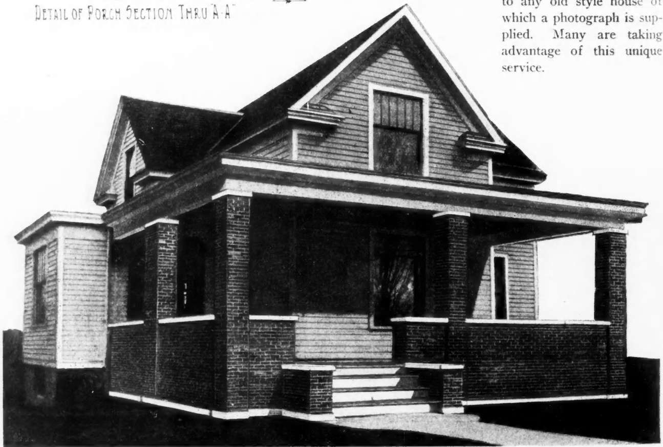
The American Builder Suggestion as to Modernizing the Padgham House by Building on an Attractive, Substantial Face Brick Porch.
