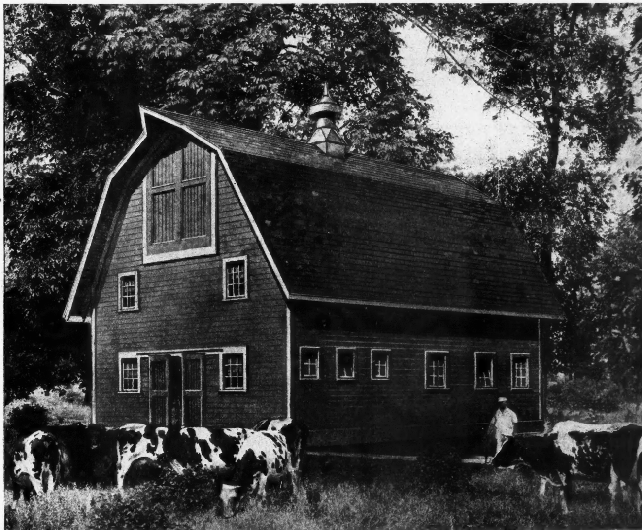
Exterior View Common in Its Principal Points to Each of the Three Arrangements Shown on Opposite Page. We Can Furnish Blueprints and Typewritten Specifications for Any of the Three Plans for Only $7.00 Per Set.
