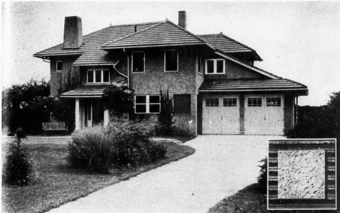
Ten Thousand-Dollar Residence of John G. Meister, Toledo, Ohio. M. M. Stophlet, Architect. Roof is Green Tile, Walls Clay Blocks Stuccoed Rough Cast Finish. Detail of Scoring on Face of Blocks and of Stucco Finish Illustrated in Lower Right-Hand Corner.
