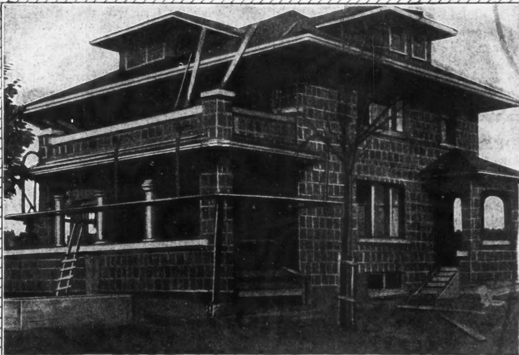
THE KOERBER RESIDENCE, FOREST PARK BOULEVARD, FT. WAYNE, IND. Before the application of the stucco finish, showing the
