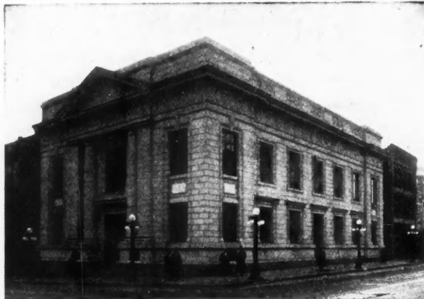
GERMAN SAVINGS BANK, DAVENPORT, IOWA Archts., Clausen & Clausen; Contrs., W. M. Allen Sons & Co.
