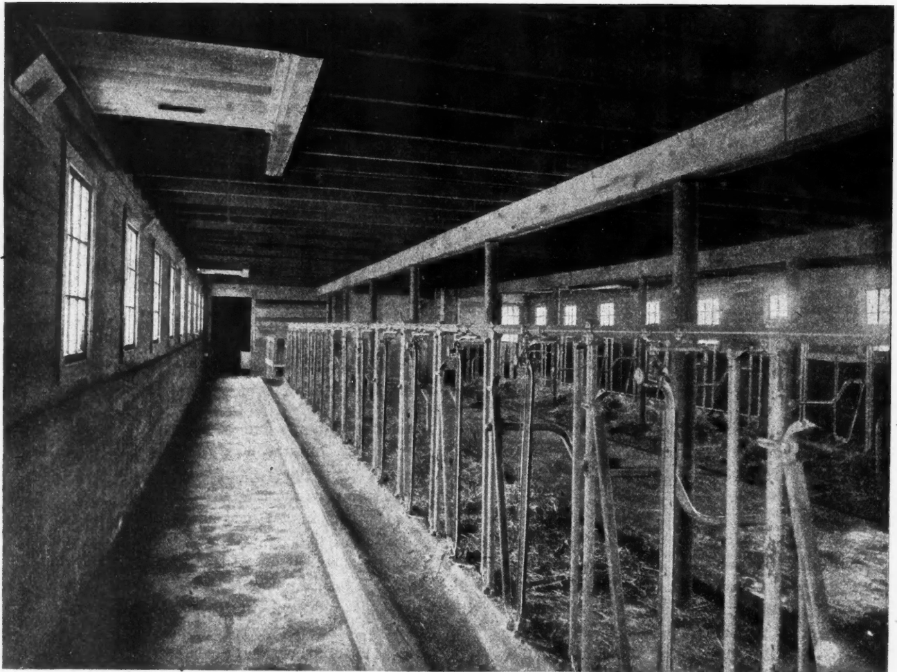
This Interior View Shows One of the Feeding Alleys of the Vaudreuil Lumber Company's Barn. Notice Concrete Manger, Modern Stall Equipment and General Bright and Business-Like Appearance.
