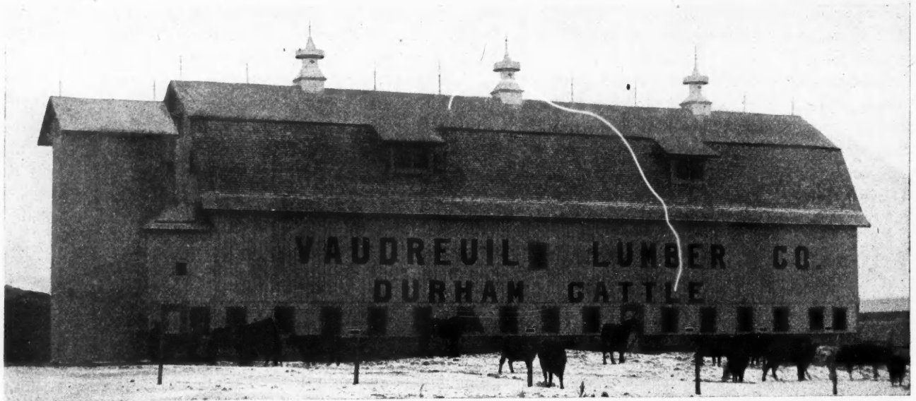
Photographic Perspective of Large General Barn Built from Plans Furnished the Vaudreuil Lumber Company of Chippewa Falls, Wis., by Our Architectural Department. (Design A370.)
