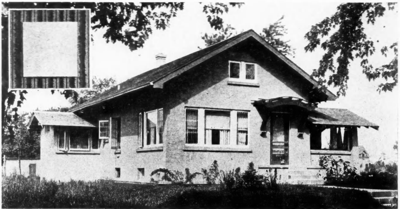
Modern Structural Tile Bungalow in a Chicago Suburb finished very attractively with smooth sand finish stucco. Detail of scored face of block with square of stucco applied is illustrated in the upper left-hand corner.
