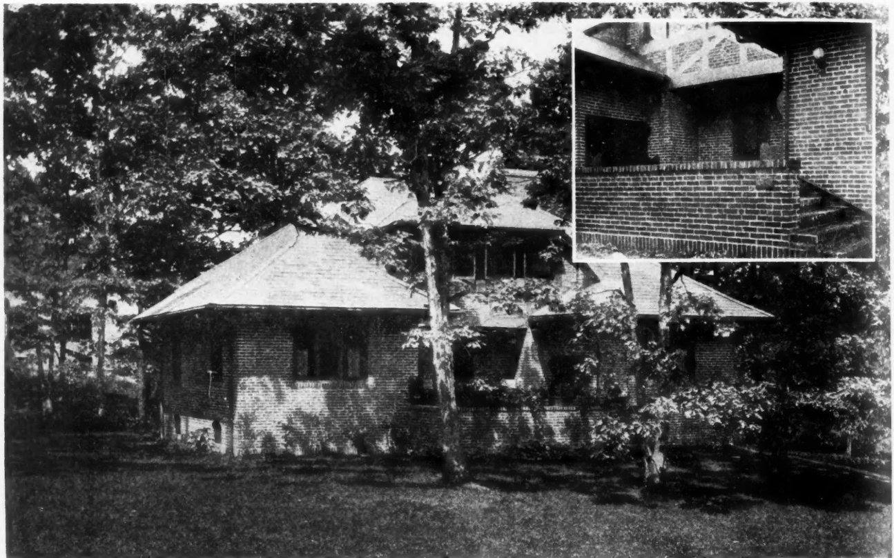
The Natural Beauties of the Wooded Building Site Give Added Attractiveness to the Brick Veneered, Slate-Roofed Dwelling of Mr. Carl S. Dow. Built in a Boston Suburb for a little over $5,000.00. Chalmers S. Clapp, Architect. Square inset shows details of entrance porch with its interesting heavy timber work above the door.
