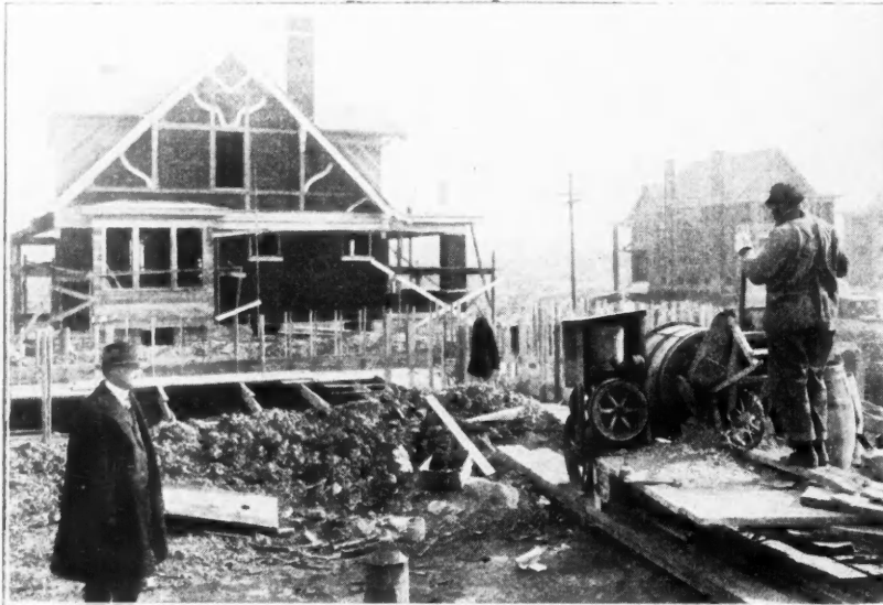
The Ideal Cincinnati No. 5 on a Foundation Job.
