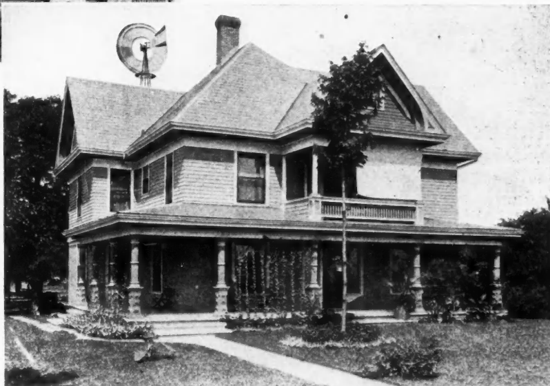
Modern Farm House Designed for Convenience, Well Built and Equipped with Plumbing, Heating, Electric Light, etc.
