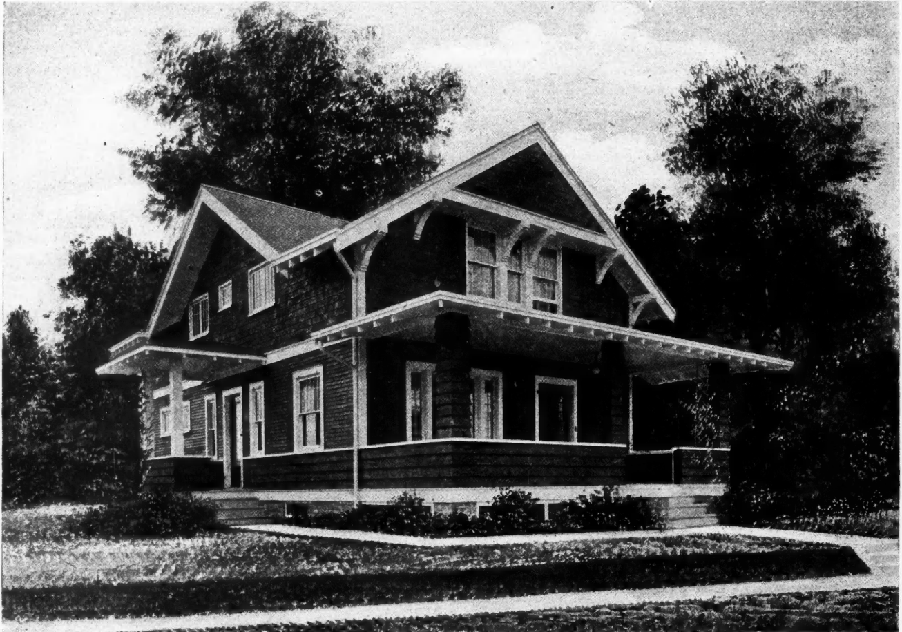
Two-Story Bungalow. Size, 26 feet by 38 feet. We can furnish complete set of blueprinted working plans and typewritten specifications for only $10.00 per set. Blueprints consist of basement plan; roof plan; first and second floor plans; front, rear, two side elevations; wall sections, and all necessary interior details. Specifications consist of twenty-two pages of typewritten matter. When ordering, ask for Design No. 6879.
