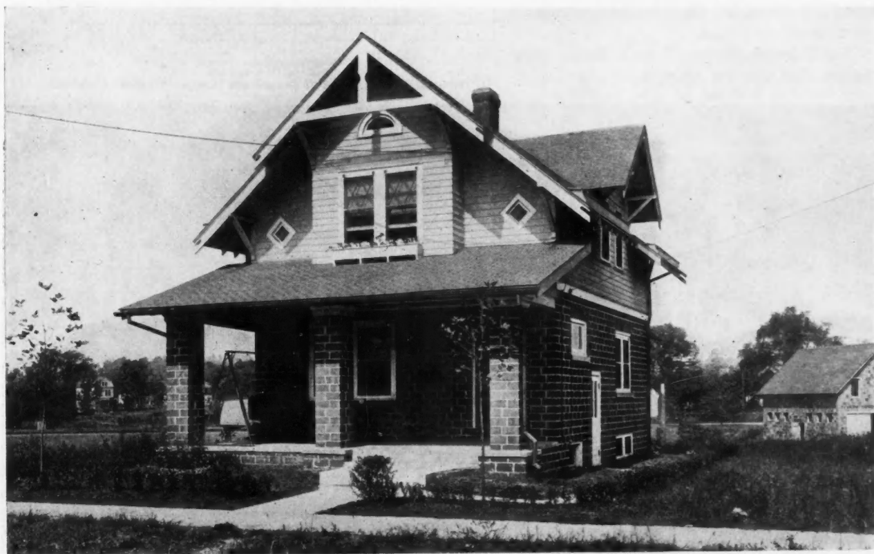
The Sinclair House at Lyons Farm, N. J., is a Good Example of Art-Tile Construction. The Dark Reddish Brown Tile Has a Pleasing Rough Brick Surface, Yet Impervious. The Mortar Joints Come Out in Strong Contrast. The Second Story is Shingled.
