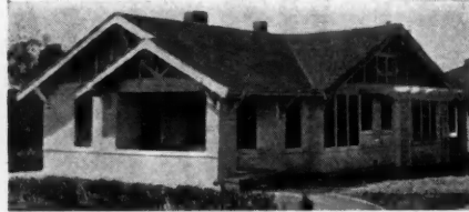
Plastered With Stucco A five-room Interlocking Tile bungalow built for $3,400 in Texas.
