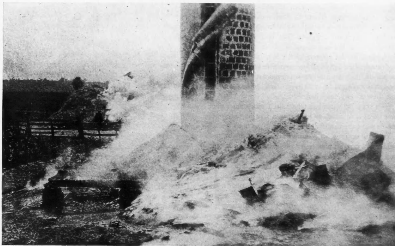
Unusual Photograph of Fire Near Freeport, Mich., Where Two Large Barns and a Straw Stack Burned, Leaving Practically Unharmd the Clay Tile Silo. The Doors and Feed Shute Were Burned Off; That Was All.
