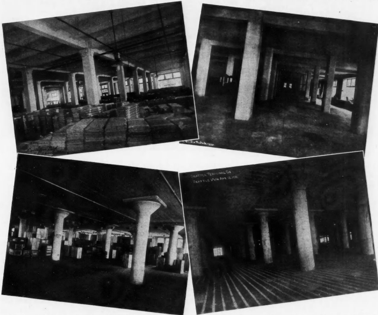
Fig. 1. Group Showing Development of Concrete Building Types. 1a (Upper Left), Beam and Girder Floor; 1b (Upper Right), Girder and Slab Floors; 1c (Lower Left), Flat Slab Floor; 1d (Lower Right), Later Type of Flat Slab Floor with Drop Panel Over Column.
