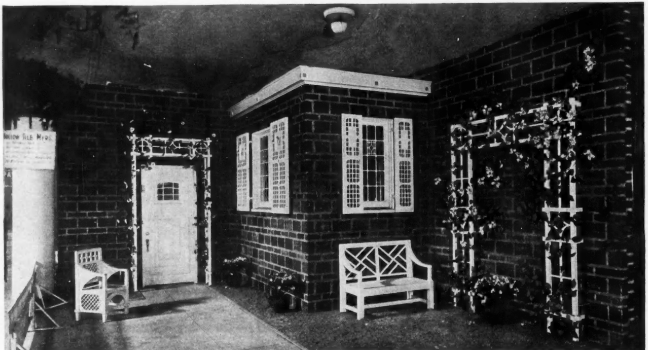
Demonstration of Self-Facing Rough Texture Hollow Building Tile at the Cleveland Complete Building Show.
