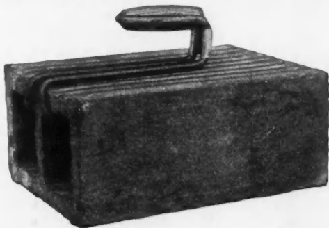
Showing How the Tile Hook is Used.
