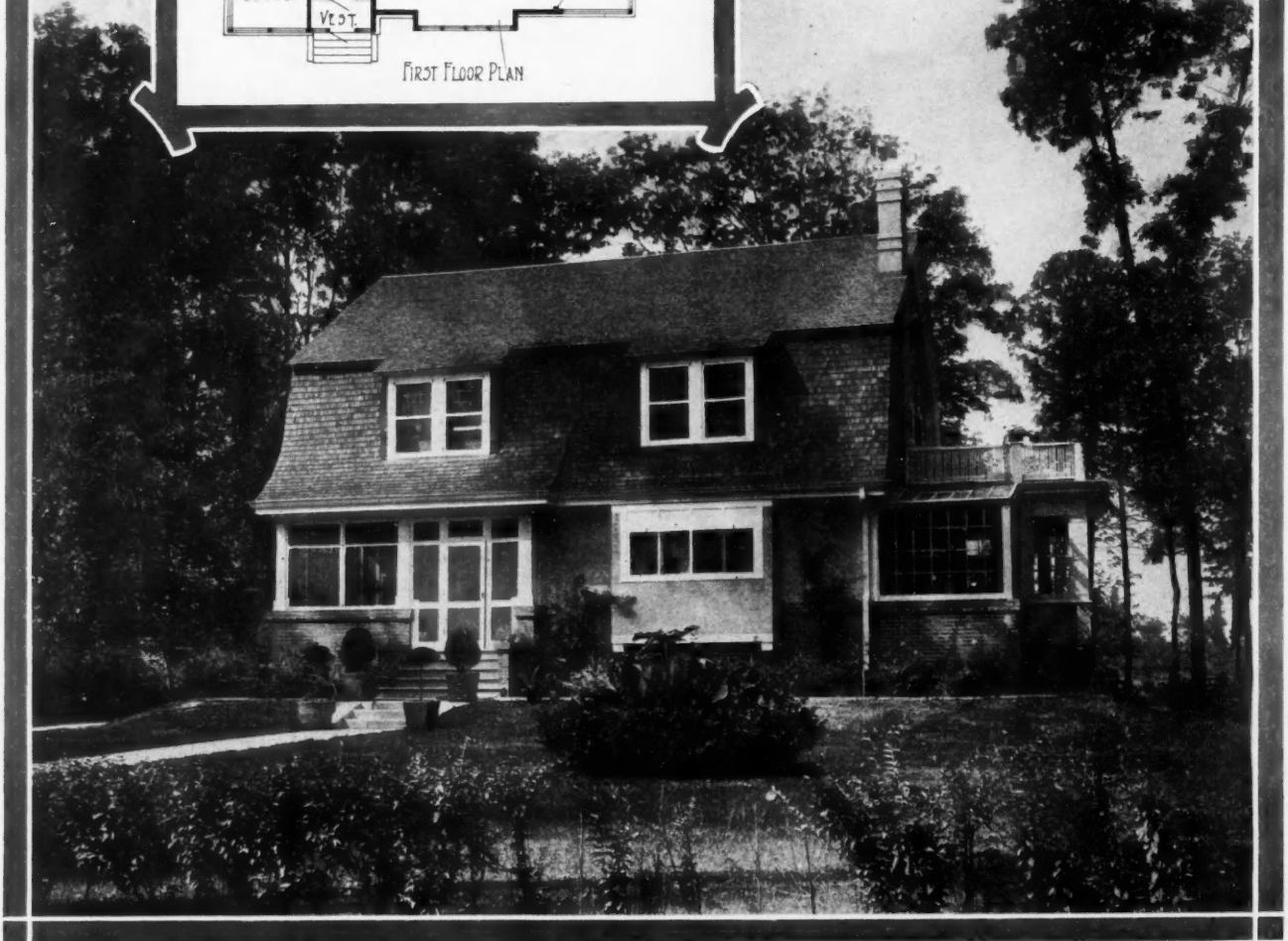
GAMBREL ROOF HOUSE WITH UNIQUE ROOM ARRANGEMENT. The exterior appearance of this house depends largely upon the roof. The walls are finished with brick up to the porch rail copings and with stucco the remainder of the way up to the roof. In the room arrangement, attention is called to the screened porch, sleeping porch, conservatory and balcony. These are features which many people are enthusiastic about. The relative position of living room, dining room and kitchen is commendable. This house is 53 feet by 29 feet 6 inches.
