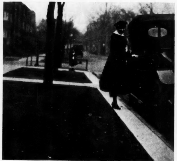
Narrow Concrete Walk Along Curb on Fargo Avenue, Chicago.
