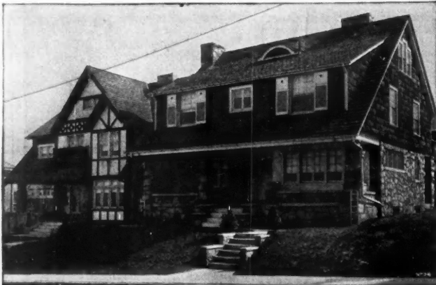
OWNER AND BUILDER, ALBERT BERTALOTT, JR., SQUIRREL HILL, PITTSBURG, PA. "CREO-DIPT" 24' SHINGLES ON SECOND STORY.
