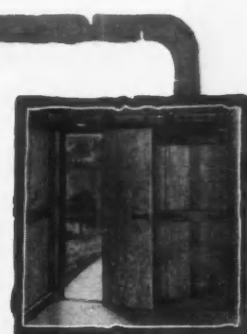
Swinging section of Louden-Hung garage door permits individual entrance and exit without moving entire door.
