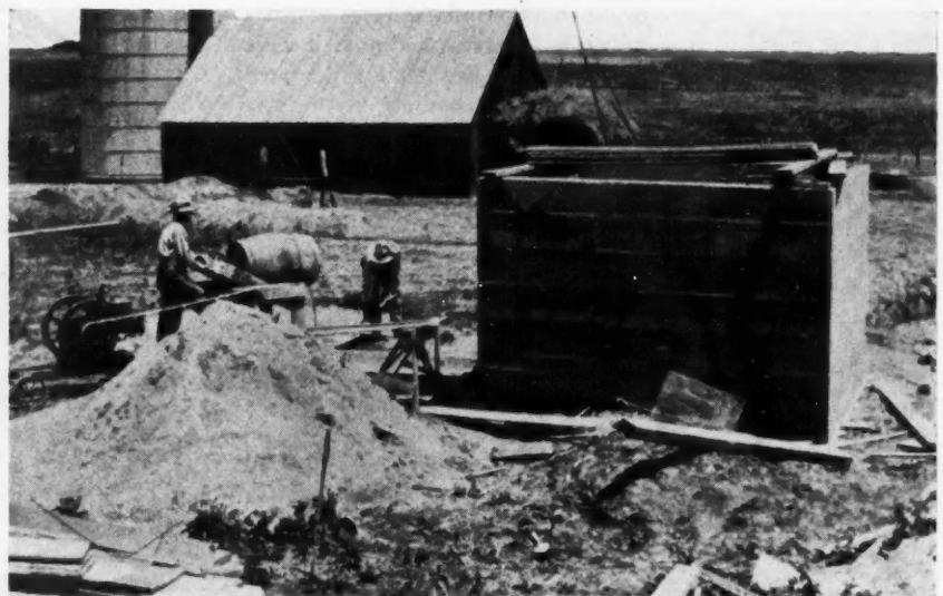
This View Shows the Mixer Made From a Barrel, Being Used by L. H. Brehm, Near Neligh, Nebr.
