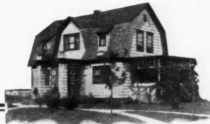
Home of Arch. Carl E. Morrison, Erie, Pa. 24-inch "CREO-DIPT" DIXIE WHITE Stained Shingles on side walls. 16-inch "CREO-DIPT" Stained Shingles (moss green) on roof.
