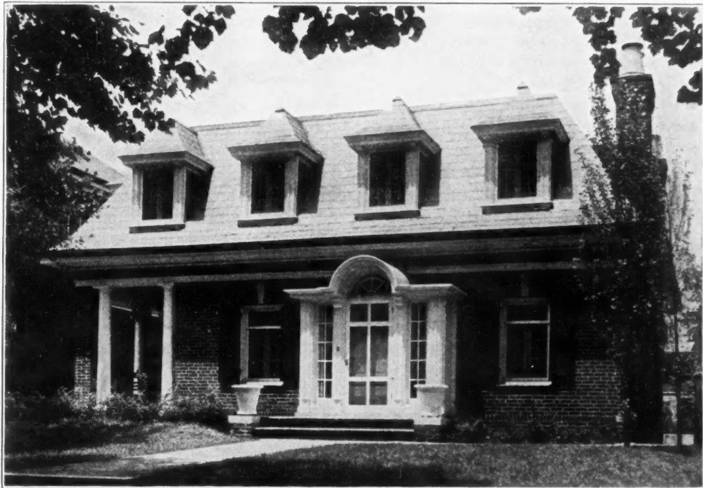
Maritz & Henderson, Architects
