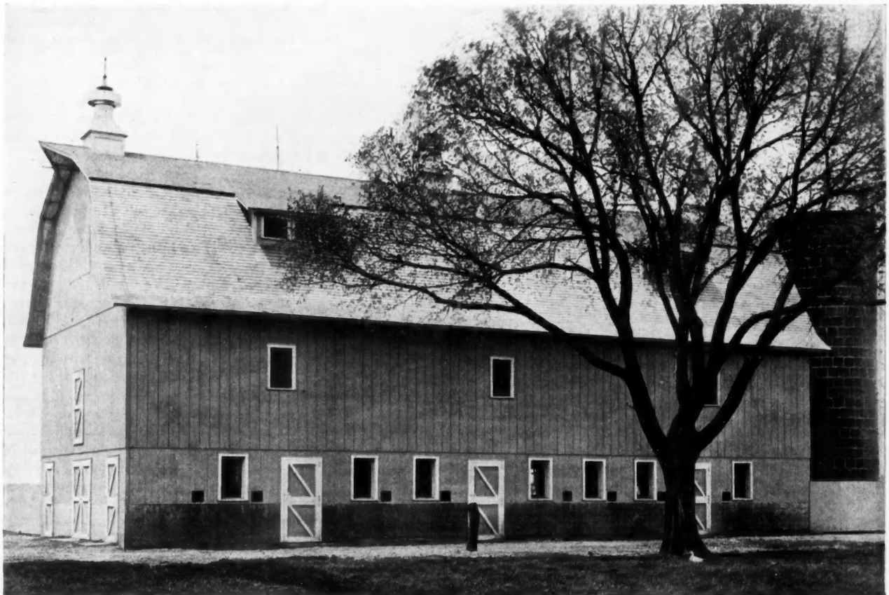
Photographic Perspective View of Dairy Barn 76 Feet 6 Inches by 36 Feet, Built Near Janesville, Wisconsin. This Barn Has Concrete Foundations and Floor and Concrete Block Basement Wall. Large Hay Mow Storage Space Is Provided Which, Together with the Tile Silo, Provide Adequate Feed Storage for the Forty or More Animals Which It Is Intended to House.
