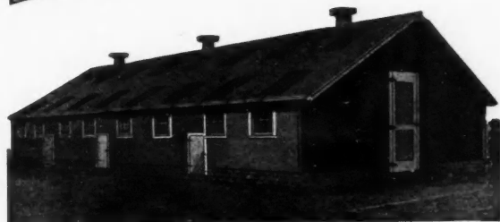
Detail drawing of this hog house will be mailed to you upon request
