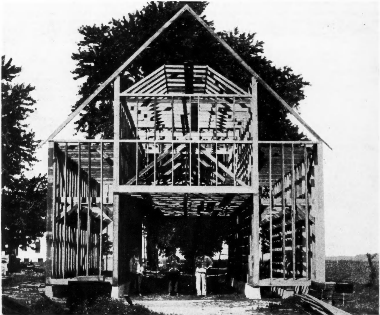
A Well Framed Two-Story Corn Crib by C. C. Robinson and Men Near Reddick, Ill.
