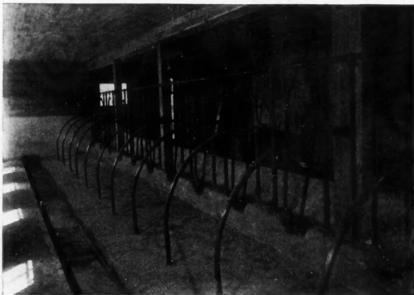
View of Cow Stalls Before Cork Brick Was Laid.
