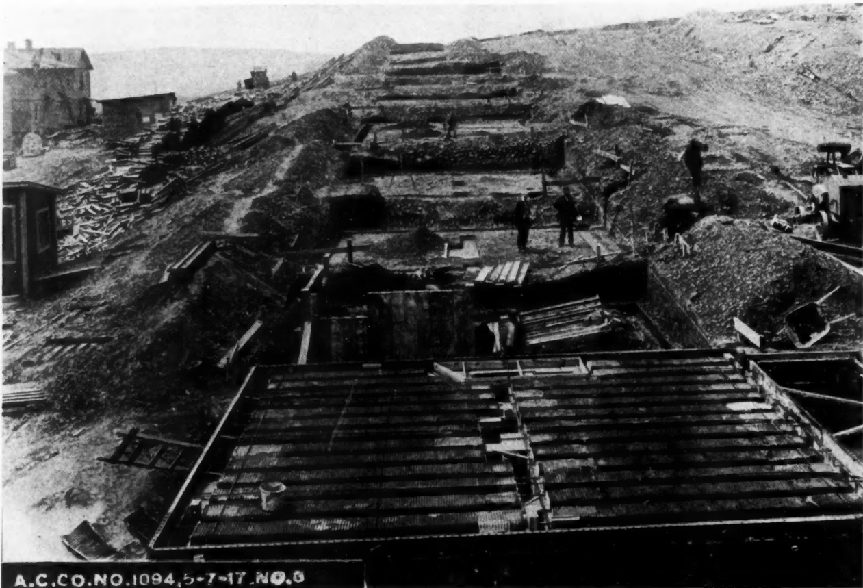
Progress Photo of Donora Concrete Housing Job, Showing Foundation Work. In the Foreground Tin Tile is in Place for Pouring a First Floor.
