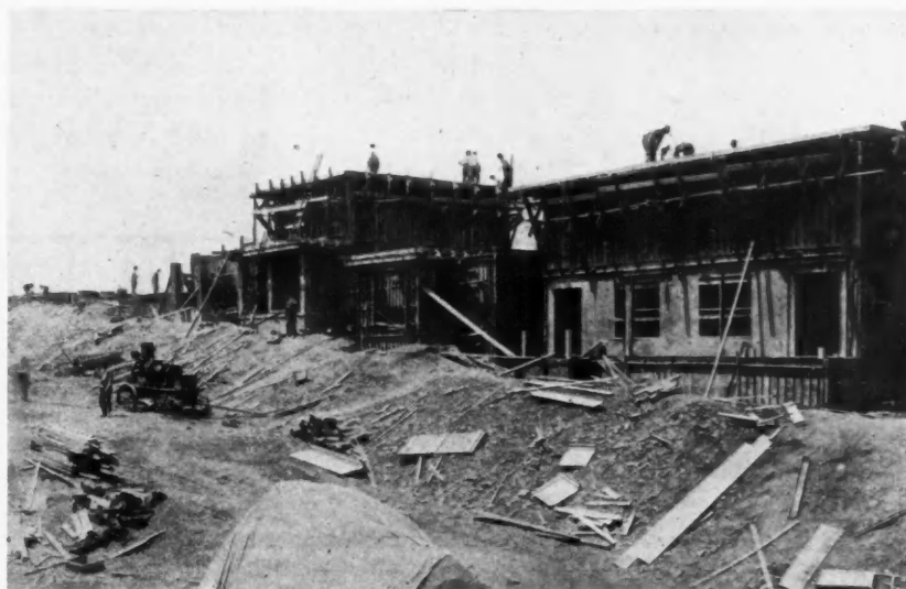
Steel Forms in Place for Pouring the Second Story Walls.
