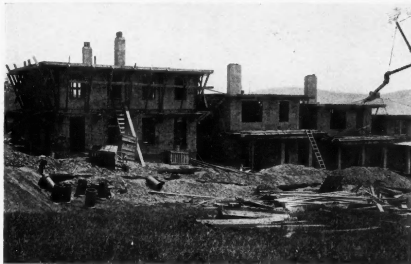
Pouring the Roof at Donora.
