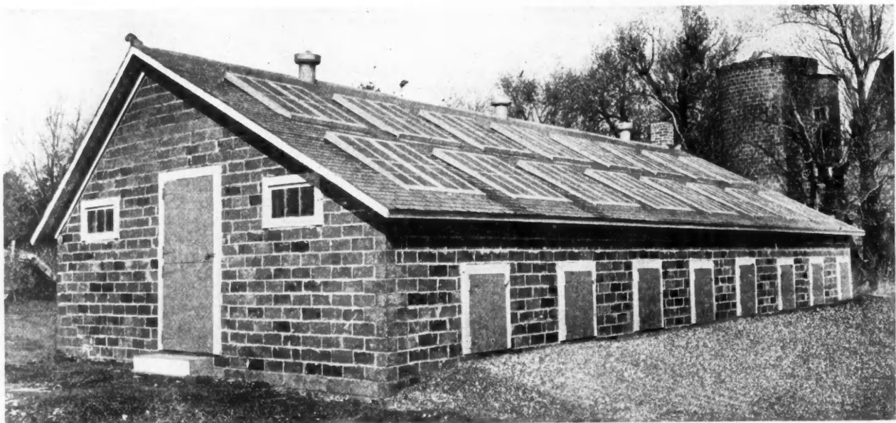
An Extra Substantial, Warm and Permanent Community Hog House, with hollow tile walls and sunlight windows. Size is 22 by 56 feet. Fifteen pens and a feed room with cooker are provided. The long slope of this roof faces the South. Outside pens are to be built later.
