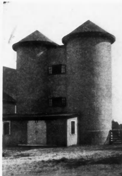
These Twin Silos are Absolutely Air-tight and Water-tight
