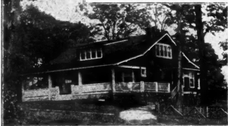
Mr. H. S. Kramer's Residence, E. St. Louis—Edward G. Garden, Architect, San Francisco
