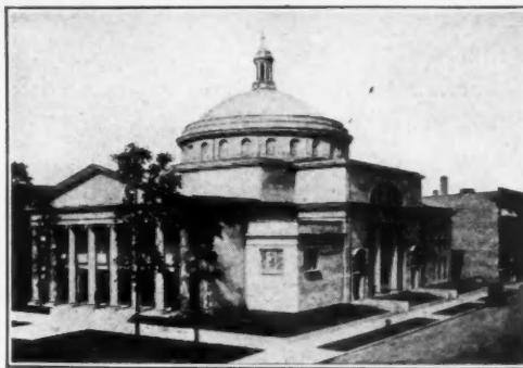
Eighth Church of Christ Scientist, Chicago, Ill. Leon E. Stanhope, Architect, Chicago
