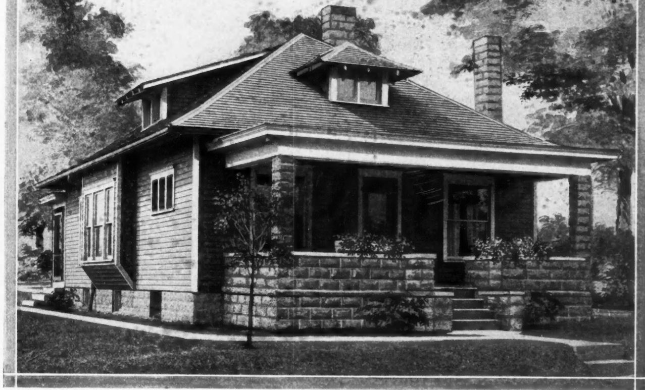
SIX-ROOM COTTAGE WITH FOUNDATION AND PORCH OF BLOCKS. Here is a sensible, straight-forward little place, size 26 by 46 feet, containing six rooms. Substantial porch gives extra weight to the design.
