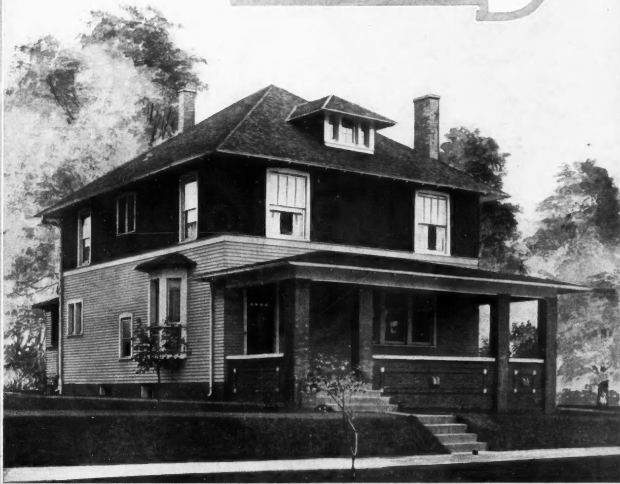
A SQUARE HIP ROOF RESIDENCE, COMFORTABLE AND ECONOMICAL. Here the home-builder gets most for his money. Angles are costly. This house has none of them. It is all for solid substantial comfort. Eight fine rooms are provided. A combination of brick porch, light colored clapboards for the first story, and dark stained shingles for the second, catches the eye.
