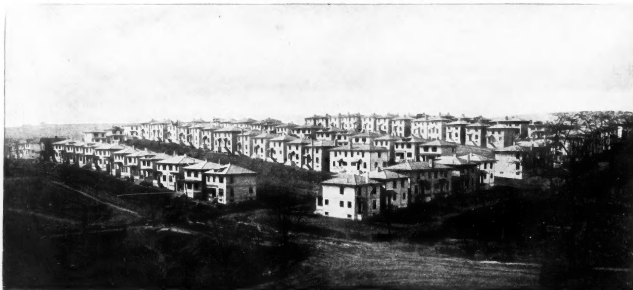
General View of American Steel & Wire Company Housing Group at Donora, Pa.
