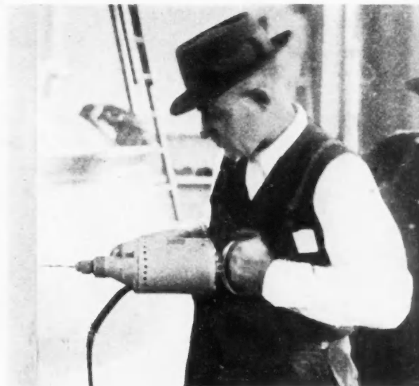
Electric Drill in a Sheet Metal Shop.
