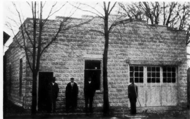
Concrete Block Garage Built by Earl Brewer at Harpster, Ohio.
