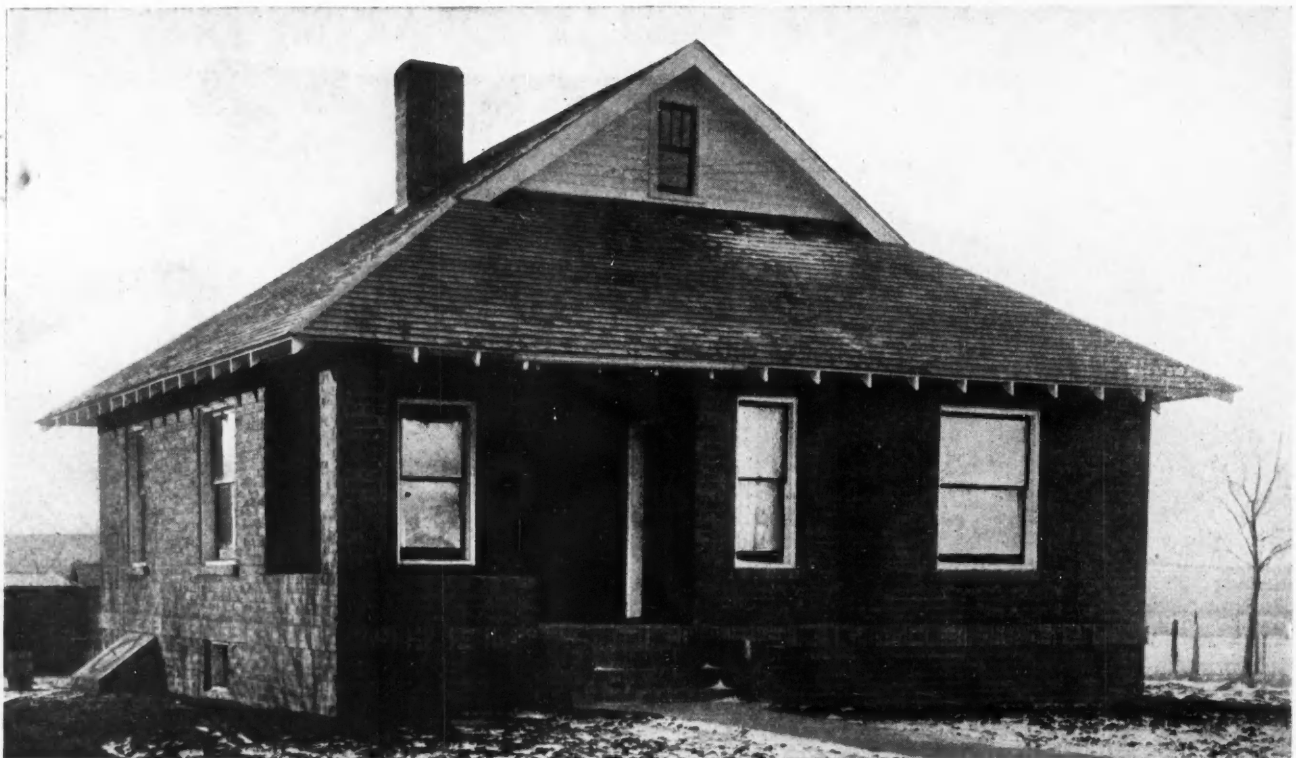
A Low Cost, Well Built Workingman's Cottage at Adel, Iowa, Constructed of a Special Brick-Face Hollow Tile. This House, Size 32 by 30 Feet, Cost Two Years Ago Only $1,750.00. Complete with Warm Air Furnace and Piping for City Water. It Was Part of a Group of Buildings Put Up by the Adel Clay Products Co. for Their Employees.
