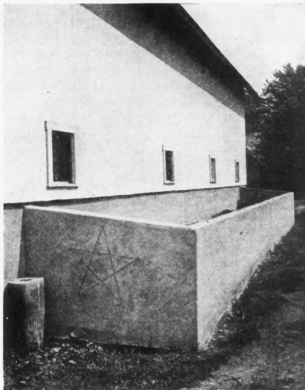
A Concrete Manure Pit Outside a Horse Barn Near Elwood, Ind. This encourages good housekeeping around the barn, and full use of the Fertilizer value of the manure.
