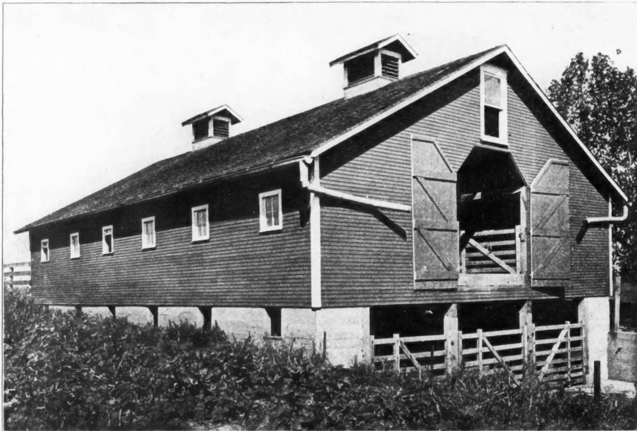
A Two-Story Sheep Shed for a Sloping Site. The Main Floor Is Entered From the Far End at Ground Level. It Is Fenced Off with Pens in the Simplest Sort of Way. Down Below There Is a Big Basement Stable with Concrete on Three Sides, But Practically Open at the Front.
