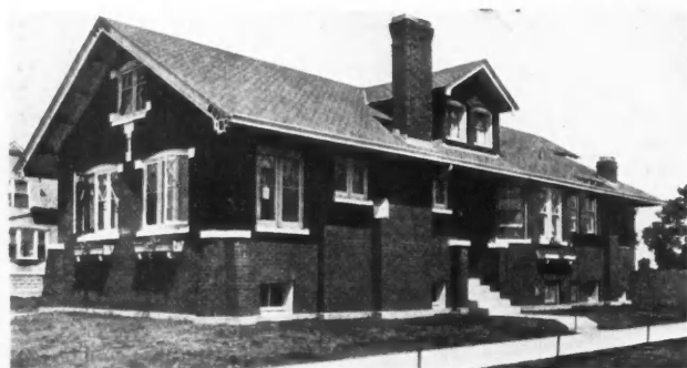
J. E. Hettinger Residence Chicago J. E. Scheller Architect
