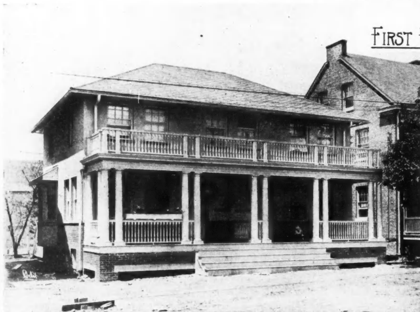
Type of Two-Family Houses Erected by the James Stewart Construction Co. for the Remington Union Metallic Cartridge Co. at Bridgeport, Conn. Alfred C. Bossom, Architect. These Houses Are of Permanent Construction, Hollow Tile, Stucco Finish. At Least Three Different Designs for the Exterior Were Used in Connection with the One Standard Floor Plan, the Changes Being Made Principally in Front Porch Treatment and Shape of Roof.
