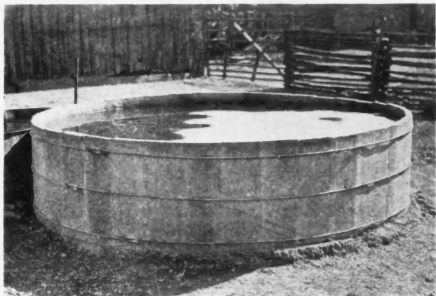
Farmyard Improvements Promote Better Farm Management and Sanitation. This round stock tank is made out of concrete staves, hooped and cemented together and resting on a concrete base.
