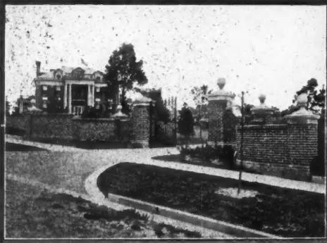
Residence of Mr. Harvey Seward, Petersburg Va. Architects - Corneal & Johnston - Richmond Va.
