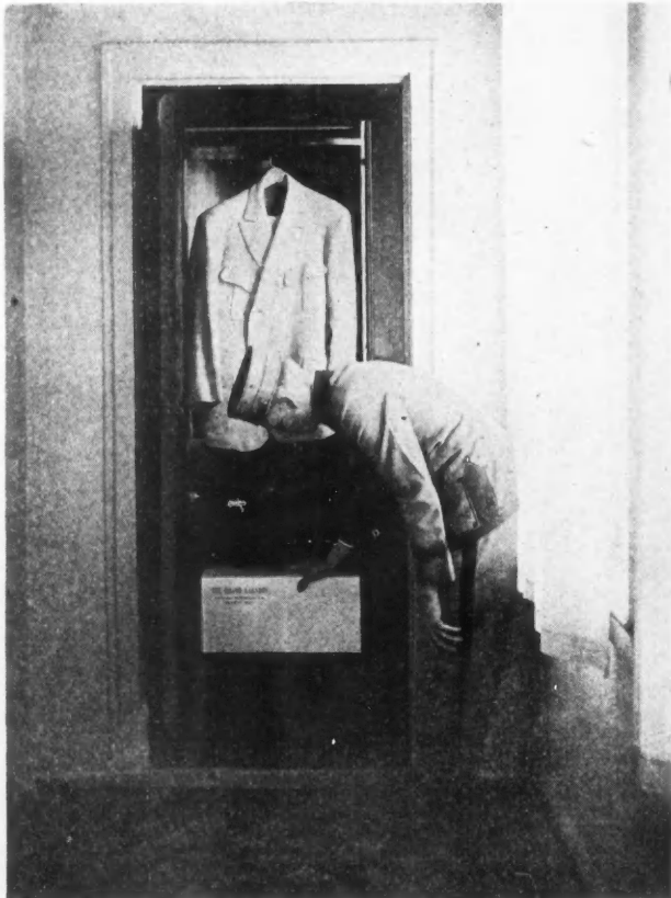
The Outside and Inside of New Style Guest-Room Door for Hotels. At the Left the Bell Boy Is Depositing Pressed Suit and Laundry in the Door Package Receiver. To the Right This Improved Door Is Viewed From Inside the Room, Guest Removing Parcels.
