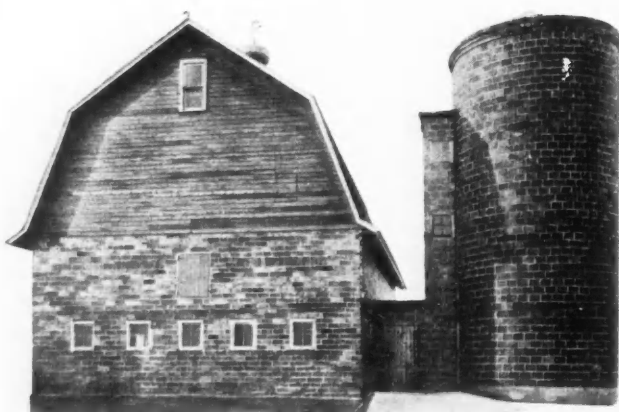
Very Well Constructed Hollow Tile Barn and Silo Near Mason City, Ia., showing the use of Structural Tile for Farm Buildings
