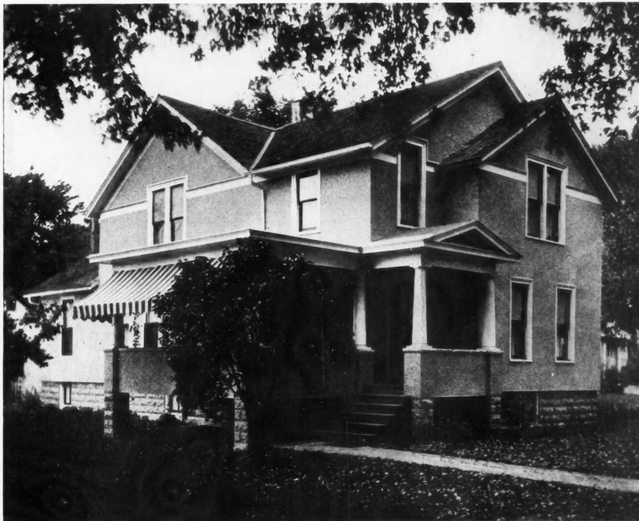
Removing the Old Style Front Porch and Building a Large Living Porch Out at the Side, and Overcoating the House with Stucco, Changed the Old Fashioned Dwelling Into a Modern Residence and Made It a Warmer, More Comfortable, and More Salable Home.
