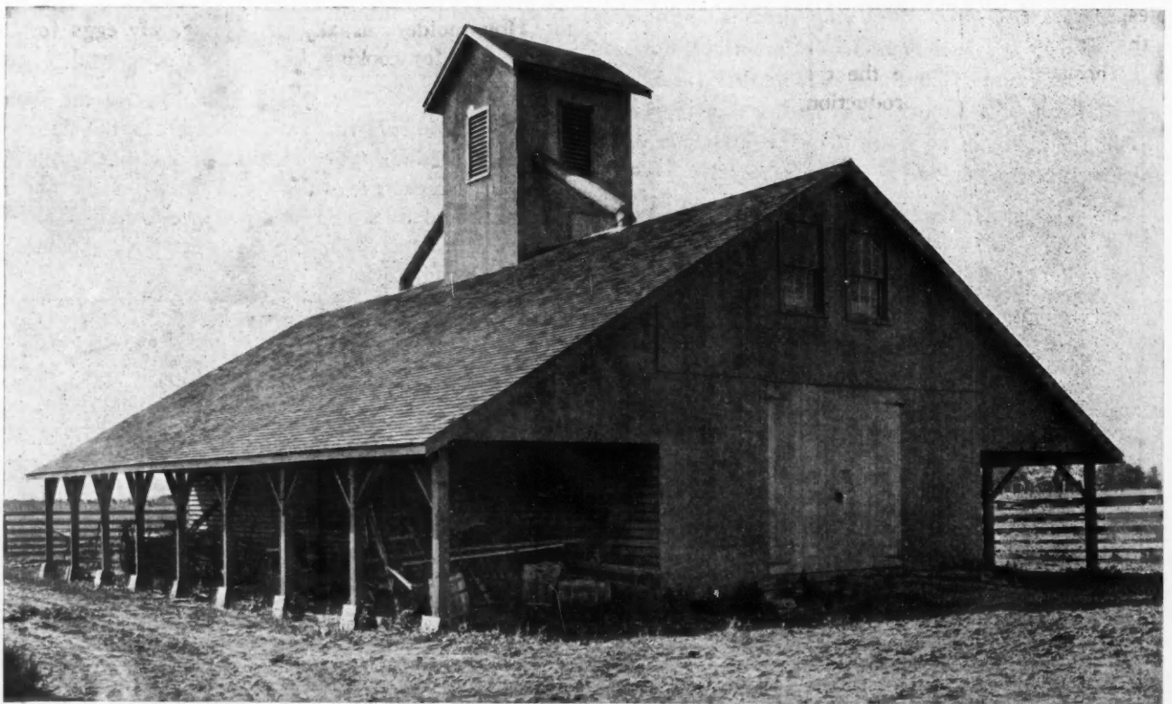
Photograph and cross section, showing construction of a very interesting farm structure near Greensburg, Ind. In center portion it is a two-story corn crib and granary, and on each side the roof has been extended out 14 feet to a line of posts to form an implement shed. This gives partial protection to farm implements at a very nominal cost. Additional protection can be easily had at any time by boarding up either or both ends and a part of the exposed side. The high cupola at the center contains the distributing head of built-in cup elevator. The two galvanized iron pipes carry the grain to the ends of the building, which is 64 feet long.
