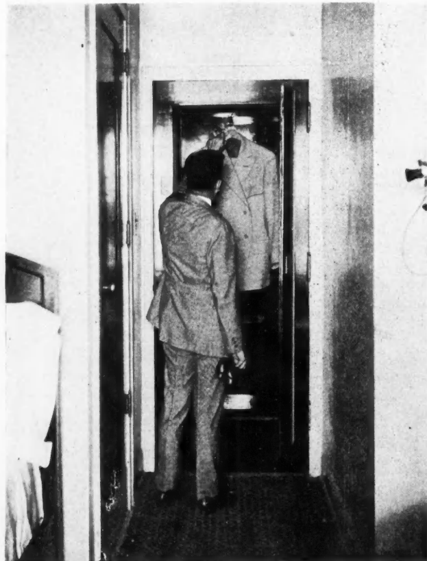
The Outside and Inside of New Style Guest-Room Door for Hotels. At the Left the Bell Boy Is Depositing Pressed Suit and Laundry in the Door Package Receiver. To the Right This Improved Door Is Viewed From Inside the Room, Guest Removing Parcels.
