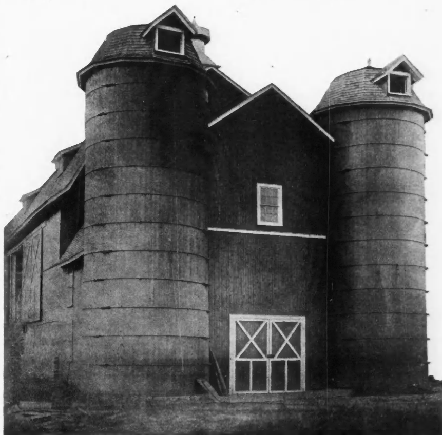
The Business End of a Modern Dairy Barn or Beef Cattle Feeding Barn; Two Exceptionally Well Built Wood Stave Silos.
