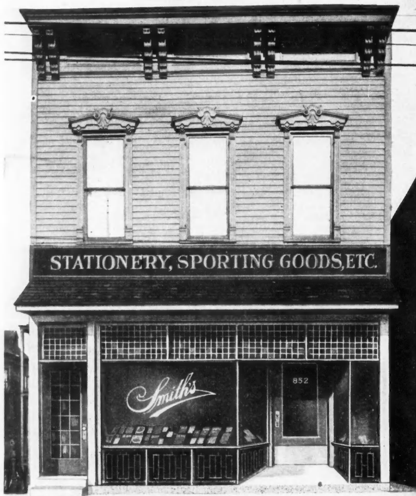
How the Old Style Double Decker Looked After Being Remodeled Into a Modern Store Building with Living Apartment Above.
