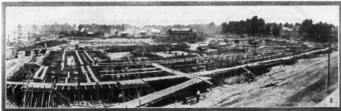
Bird's-eye view of industrial houses built for the U. S. Shipping Board Emergency Fleet Corporation, in the Sparrows Point District, Maryland. 300 houses at St. Helena, 531 at Dundalk. Exterior walls of St. Helena houses, stucco and Herringbone Rigid Metal Lath. Herringbone Lath and plaster were used for interior walls of Dundalk houses. Architect, E. L. Palmer, Baltimore. Contractors, Consolidated Engineering Co., Baltimore, G. P. Zouck, President, C. A. Cummins, Vice-President and General Manager.
