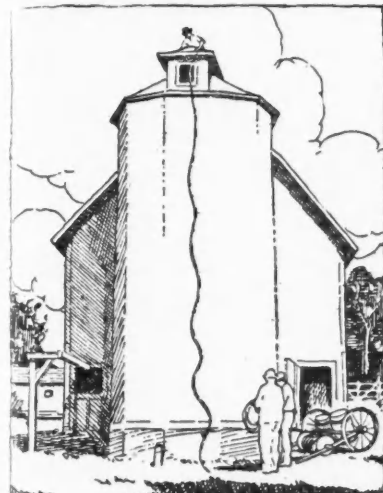
2. Rodding a Silo. Note the Cable Hanging Down Side.
