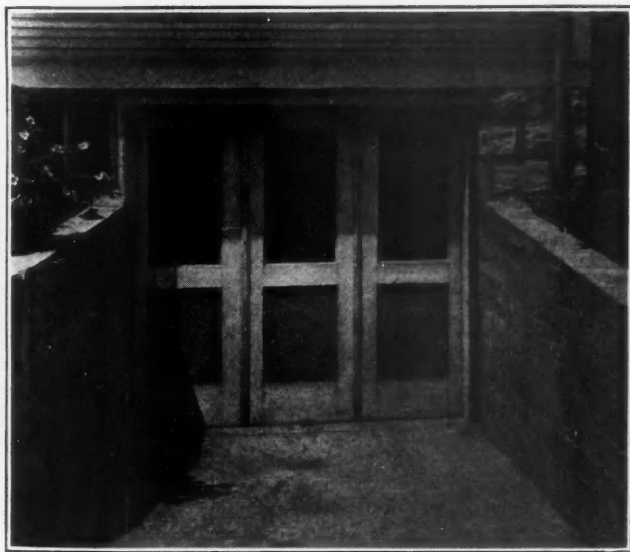
The Basement Converted Into a Garage. Only Enough Space for the Car Is Needed, the Swinging Sliding Doors Taking Up Little Room.
