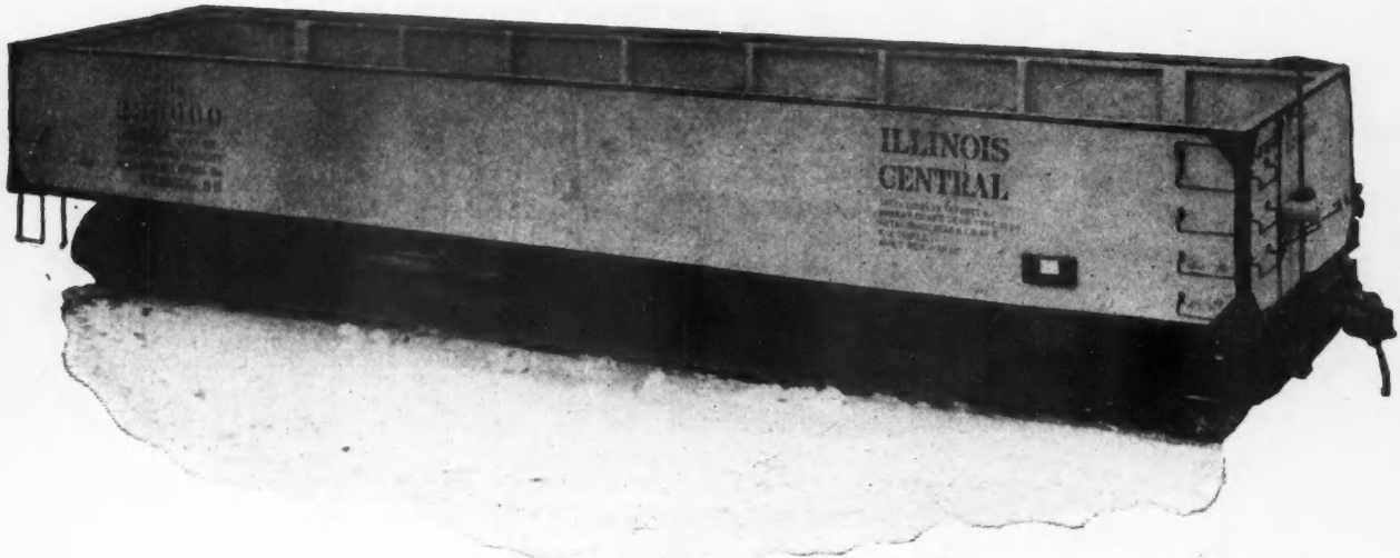
The Finished Concrete Freight Car Ready for Its Load.
