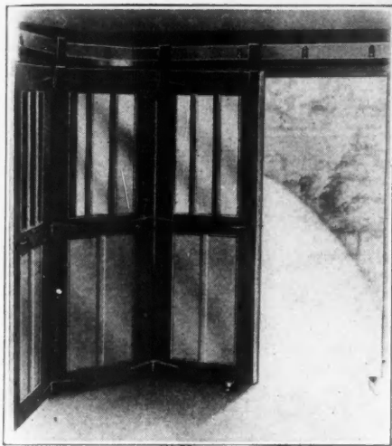
Triple Doors that Slide Around the Corner and Fit Snugly Against the Side Wall of the Garage. They Move Easily and Require Little More Than the Thickness of the Door When Open.
