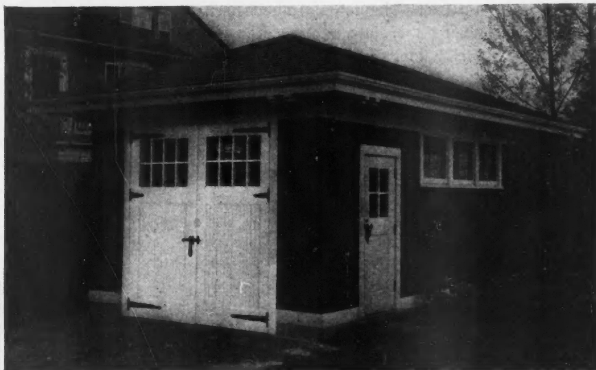
This Shingle Garage Makes an Attractive Building, and the Door Hardware Helps Greatly. These Doors Swing Out and Are Held Open by an Arm that Locks Automatically.
