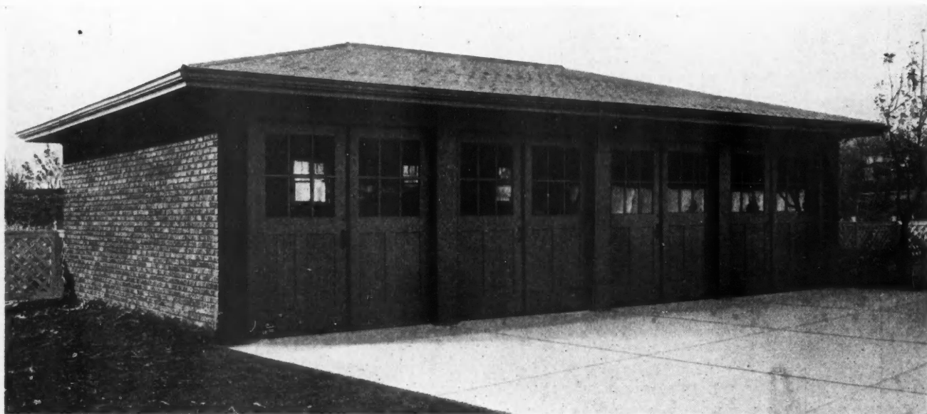
A Multiple Garage for Four Cars, Floor Plan and Cross-Section of Which Are Shown in Other Illustrations. The Plan May Be Used for Garages to House One or More Cars. The Hip Roof Makes this an Attractive Building. The Doors Are Illustrated Hung to Open in, but Any of Several Types May Be Used.
