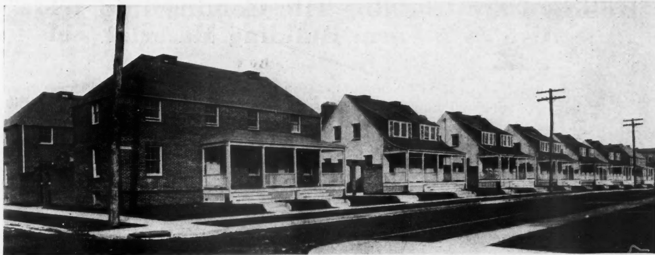
Hollow Tile Houses for the United States Shipping Board at "Sun Village," Chester, Pa.
