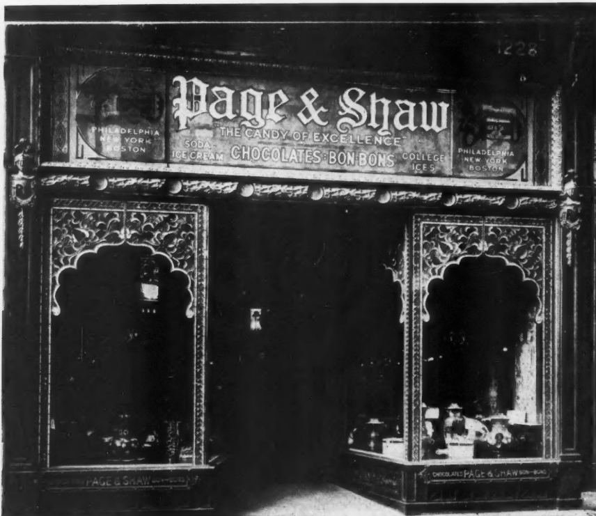
The Page & Shaw Co., Philadelphia, spent $25,000 on this elaborate bronze and ornamental glass store front. The ornamental band above the windows was in the original store, but the grill, bronze ceiling over the entrance, bronze door and ornamental glass panels inside all were recently put in. These elaborate fronts are favored by specialty shops in the larger cities.
