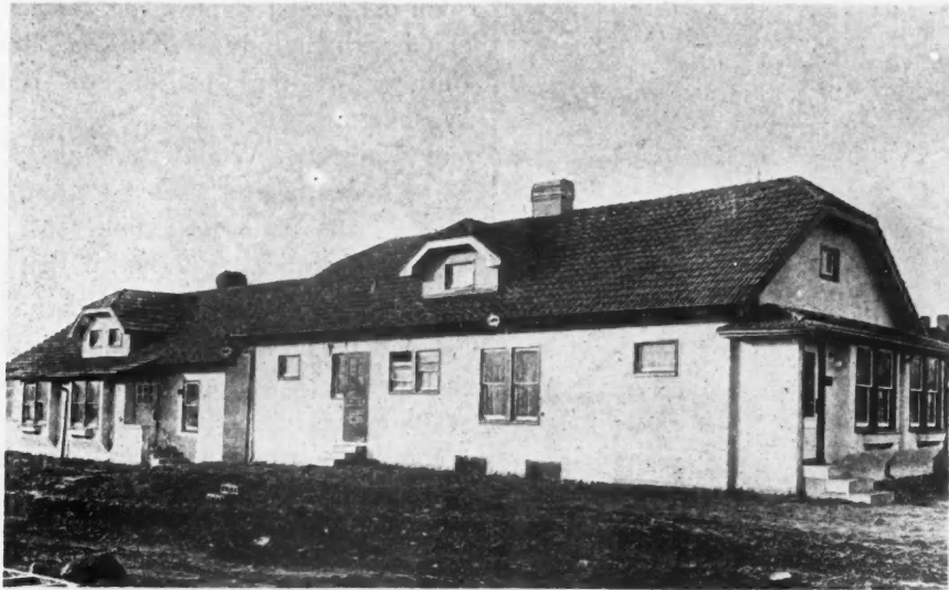
Cottage with a Brush Coat Finish of Medusa Waterproofed White Cement Circle City Construction Co., Indianapolis, Builders
