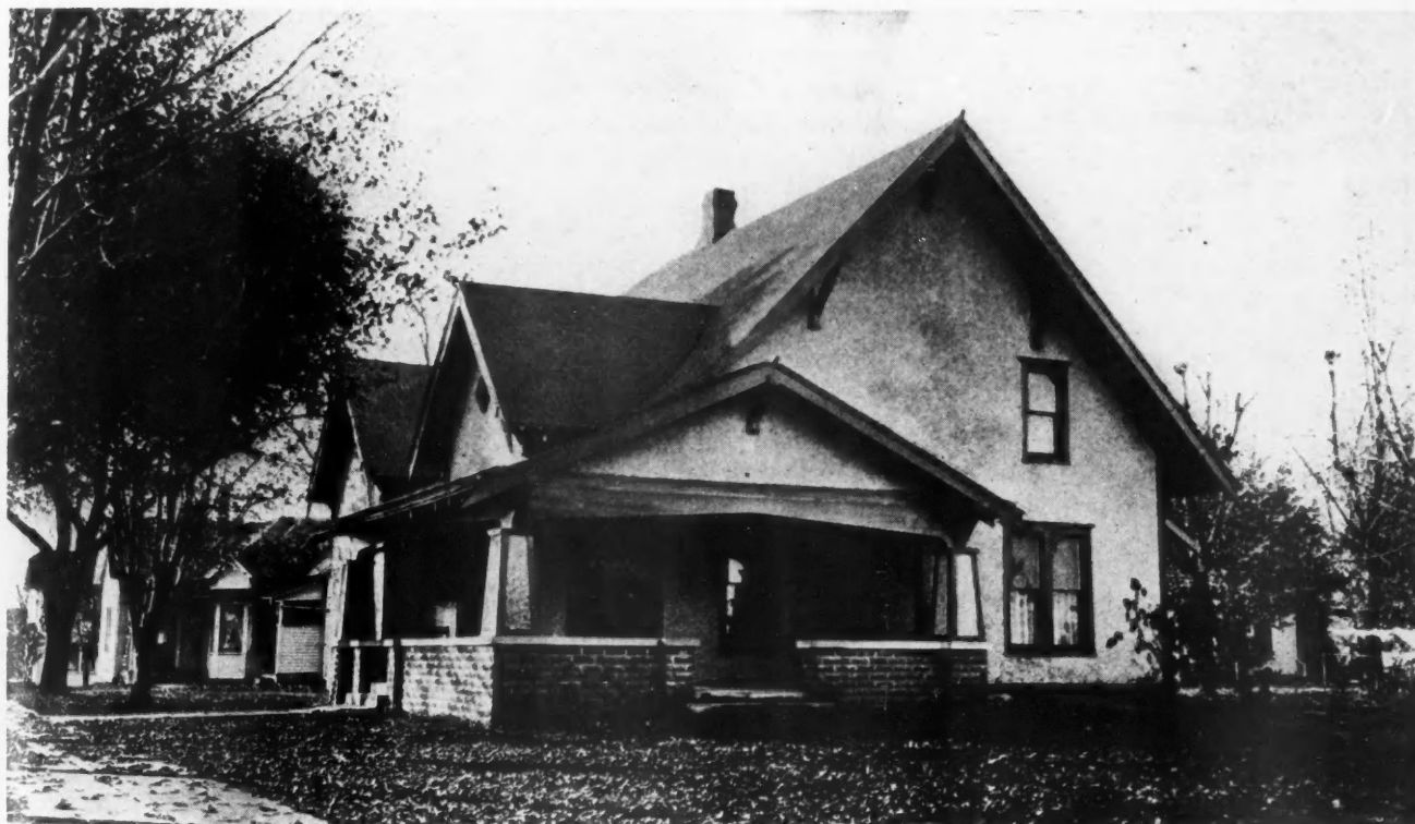
Here Is the Same House After It Had Been Converted Into a Modern Home of Attractive Appearance by Changing the Roof and Porch Lines and Applying Stucco to Wooden Lath Over the Old Siding. The Work Was Done by A. H. Stoecker, of Stanwood, Iowa.
