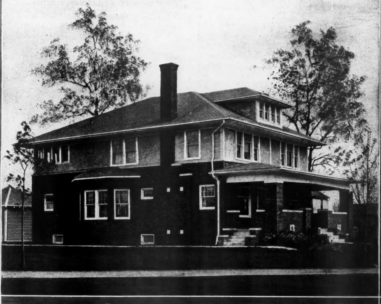
TWO-FAMILY HOUSE OF BRICK AND STUCCO. This is an exceptional design of a house for two families. Each side contains five rooms and bath besides the sleeping porch on the second floor. The hip roof and substantial attractive porch are exterior features. This is an up-to-date design for such a building and it affords the greatest possible value for the home-building funds invested in it.
