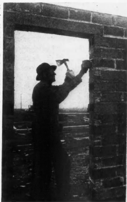
Fig. F. Proper Method of Driving in the Nailing Blocks. Vertical Wedges Cannot Split the Tile; Horizontally Placed Wedges Might Do So.
