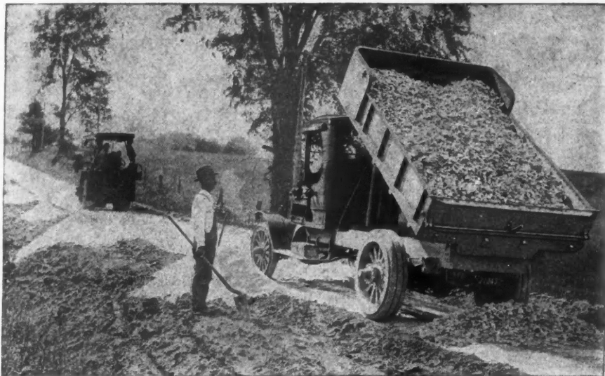
Louis Hoffman, Contractor, Hauled 33 Yards of Crushed Stone Daily Four and One-half Miles to This Road-Building Job, at Belgium, Wis., with This 3½-Ton Acme Truck.
