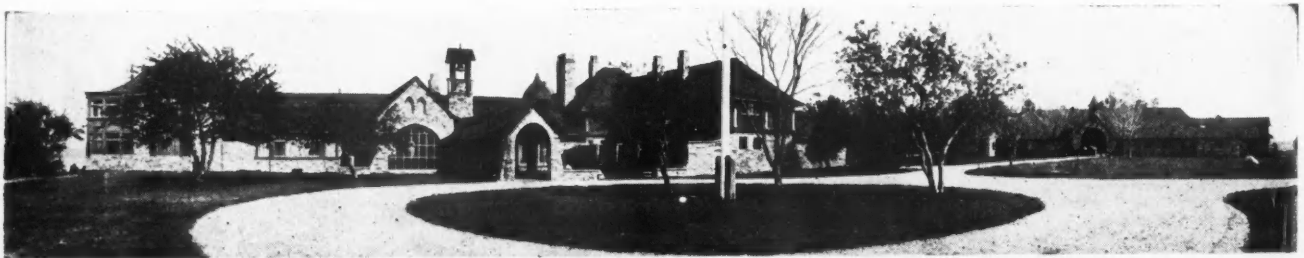
Country Home at Charlevoix, Mich.—All the Buildings Are Supplied with Electric Light from a Private Plant.
