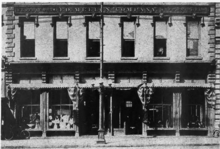
The Ed. Mellon Co. Store Before Remodeling.
