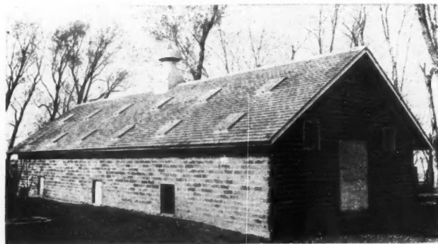
Fig. I. Hollow Tile Hog House. The Hog Entrance Door Frames Are of Concrete, Cast in Place with a Simple Wood Form. See Fig. K.
