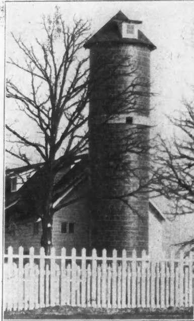
Hollow Tile Silo with Water Tank on Top; Also Detail of Tile Used.
