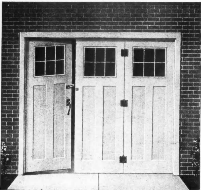
By Hanging One Door So That It Swings Free, Access to the Garage May Be Gained Without Trouble.
