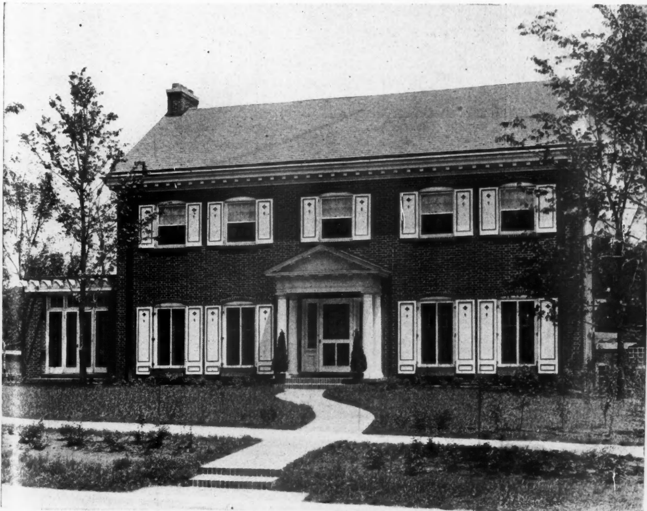
A Fine Example of a Brick Colonial House, Designed by Charles F. White, Jr., Architect, Oak Park, Ill. Face Brick Put on as Veneer to Any Other Material, Such as Hollow Tile, Wood or Common Brick Can Be Used to Produce a House Like This.
