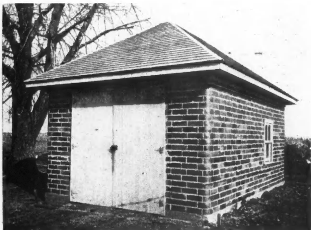
Fig. H. Garage Having Door Frames Made and Fastened as Shown in Detail in Fig. G.
