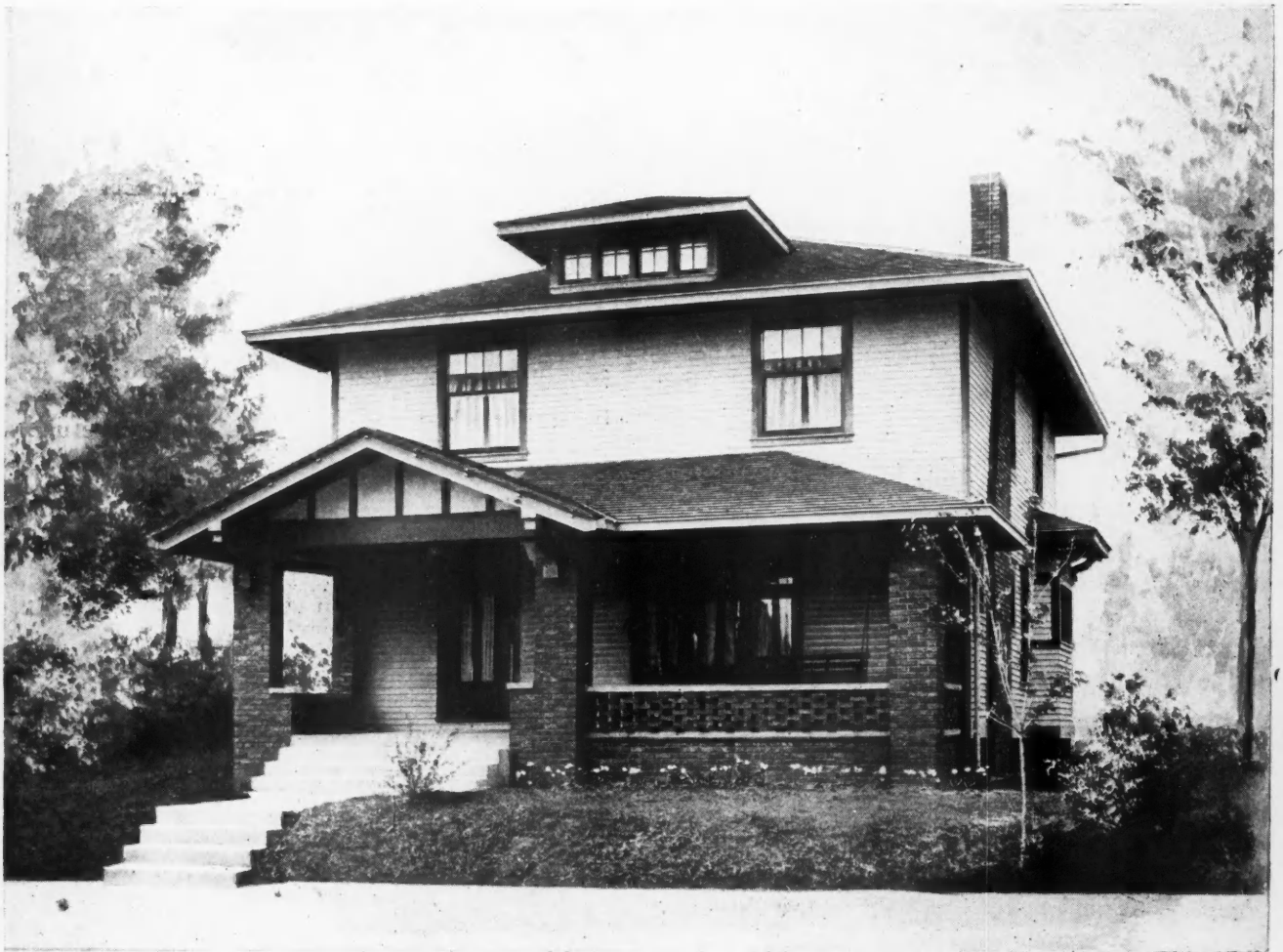
Seven-Room House of Moderate Cost. Here Is a Hip-Roof House, 28 by 32 Feet, That Is Popular. There Are no Frills About This Building, But It Is of the Type That Is Popular and Makes an Attractive and Comfortable Home. This Design Equally Suitable for Brick or Stucco. A Broad Porch with Brick Pillars Adds Greatly to the Beauty of This House.
