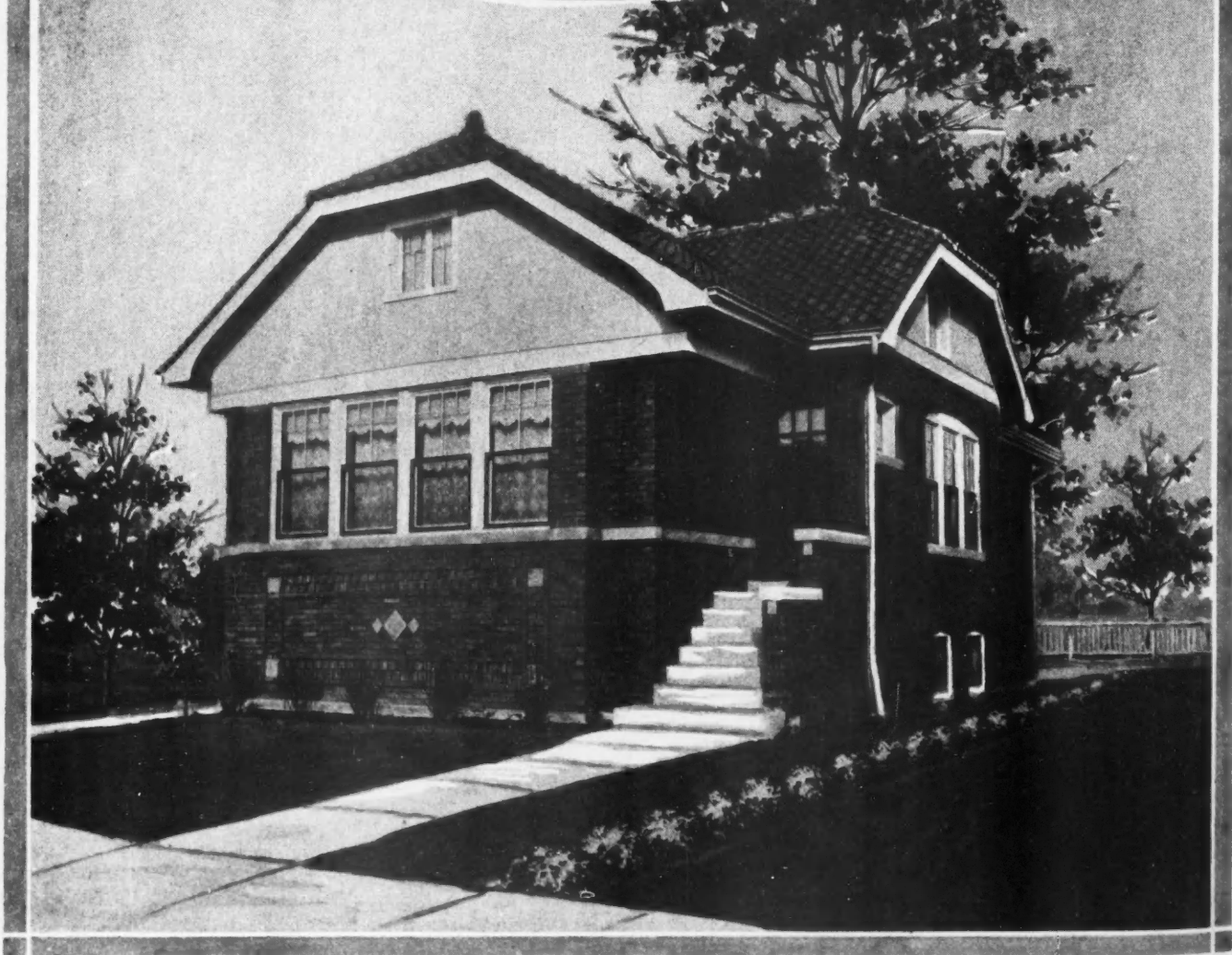
F IVE-ROOM BRICK AND STUCCO HOUSE. Here is a design for a brick and stucco house that is out of the ordinary. The house has the appearance of being much larger than it is, as it has an attic, the ceiling of which is high enough to permit the owner to finish off two or three rooms on the second floor. It is attractive in appearance, made so by the use of face brick and stucco in the gables. The dimensions are 22 by 50 feet. The foundation walls are run high above grade, saving in excavation, and also are veneered with face brick. Five rooms, all of good size and well-arranged, are shown on the floor plan. This design is suitable for both city and rural home builders.
