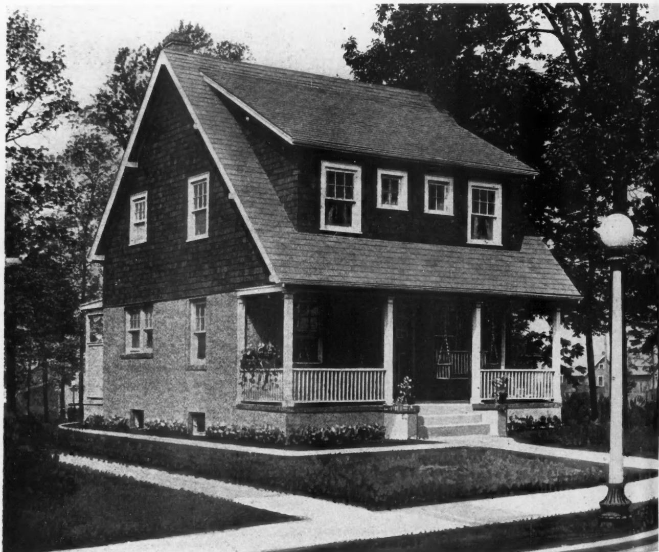
An Attractive, Economical Home. This House Is of Frame Construction, with Stucco and Shingle Exterior. It Contains Six Good Rooms and Bath. Size, 24 by 30 Feet.
