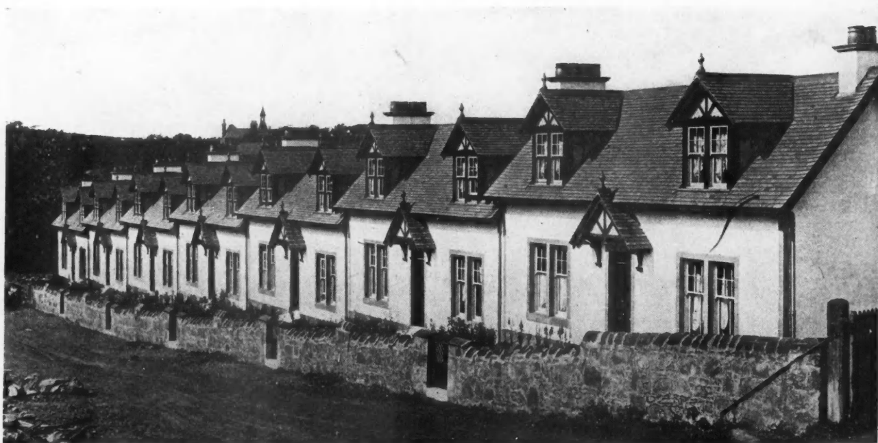
Workers' Houses at Hethercrays, Parstey, England. Stucco Over Brick with Dormers of Stucco Over Wood.
