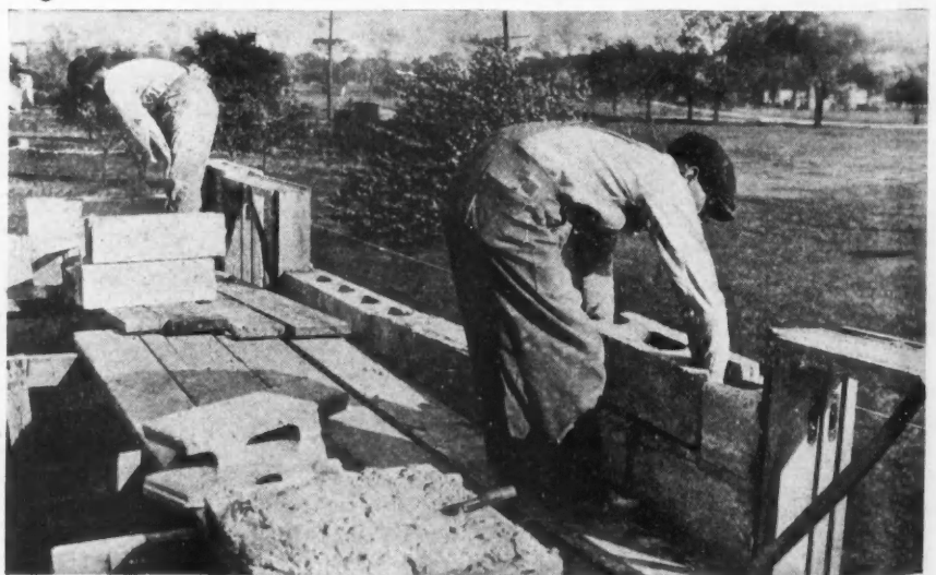
Figure 5. Laid with 3/8-Inch Mortar Joints, Each 8 by 8 by 24-Inch Block Occupies a space of 1 1/3 Square Feet in the Wall, or the Equivalent of About 12 Brick, Single Thickness or 24 Brick Double Thickness. Joints Do Not Have to Be Tucked or Pointed.
