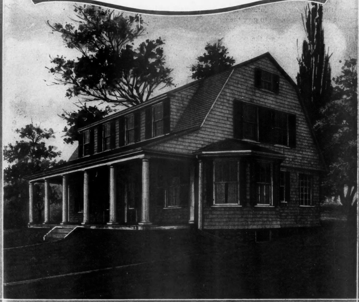
EIGHT-ROOM DUTCH COLONIAL SHINGLED HOUSE. Here is an unusual Dutch Colonial house. The full width porch, with its Colonial columns, the wide dormer and the dining room bay give it an individual exterior appearance. The size is 28 by 36 feet, with an 8-foot porch projection. The house contains eight rooms, five of which are bedrooms, one on the first floor and four on the second. The living and dining rooms are large and occupy the front of the house. As they are connected by two pairs of accordion doors, the two rooms can be thrown together. The convenient arrangement and the sizes of the rooms are shown on the floor plans.
