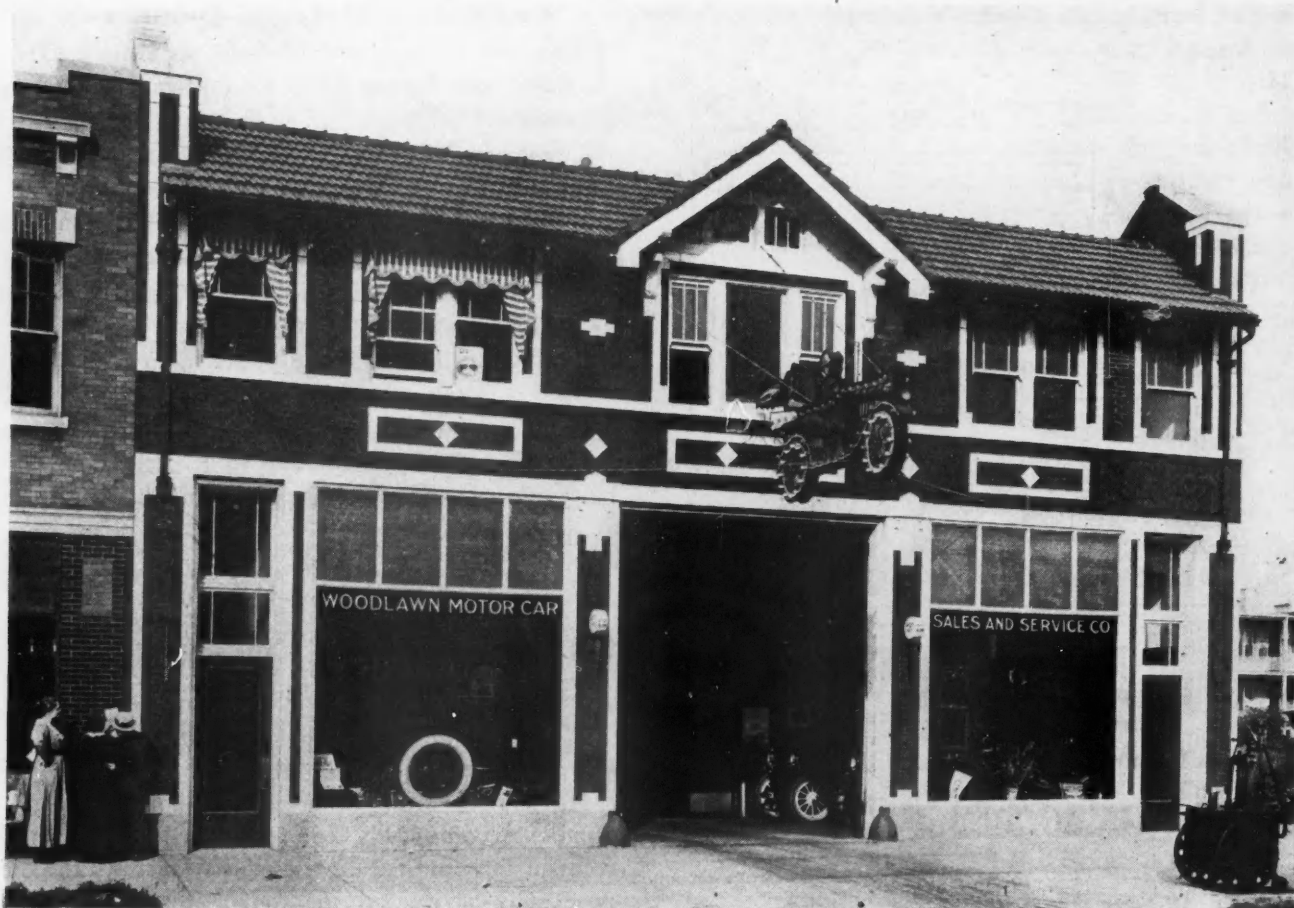
Exterior of Unusually Attractive Public Garage, with Offices at Front of Second Floor. Face Brick and Terra Cotta Beautify the Front.
