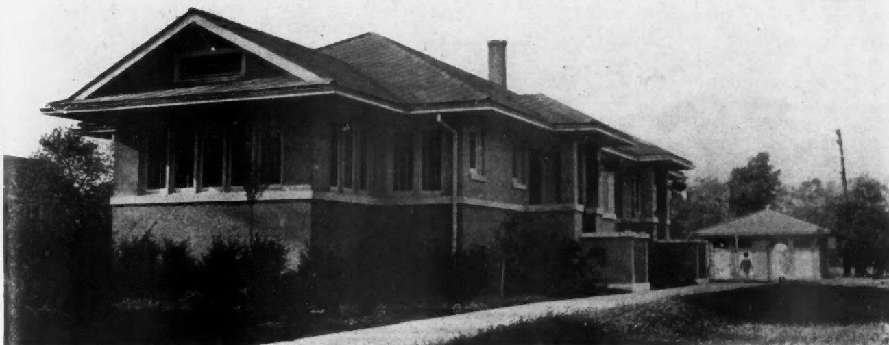
Figure 1. Concrete Block and Stucco Bungalow at Riverside, Ill. The Building Trim Is of Concrete and the Roof of Cement-Asbestos Shingles, the Only Exposed Wood Being in the Window and Door Frames.
