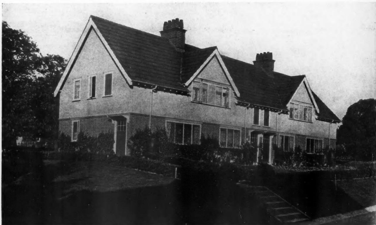
Four-Apartment House for Workers at Crawley, Hampshire, England. Brick and Stucco, with Slate Roof and Brick Chimney.
