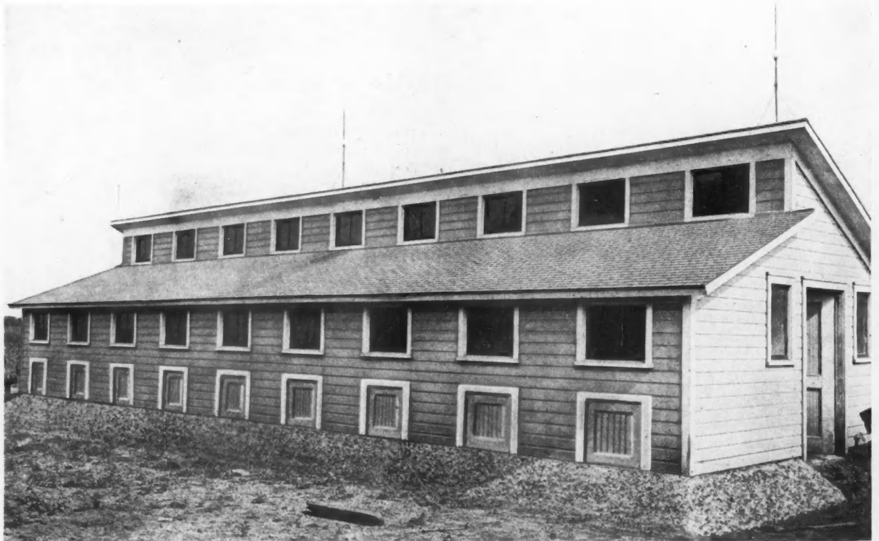
South Exposure of a Saw-Tooth, Community Hog House, That Will Provide Warm, Healthful Quarters for Eighteen Sows and Their Litters. The Building Is 24 by 54 Feet and Is of Frame Construction.
