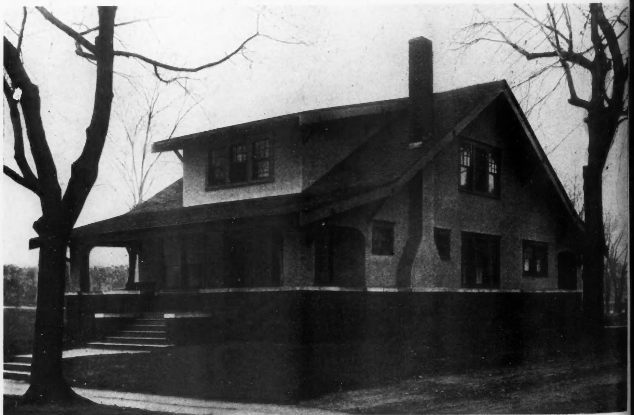
Seven-Room Story-and-Half Stucco House, Size 28 by 44 Feet, 6 Inches. This Is the House Mr. "H." of the American Builder Staff, Plans to Build. COMPLETE BUILDING PLANS IN THE BLUE PRINT SUPPLEMENT.
