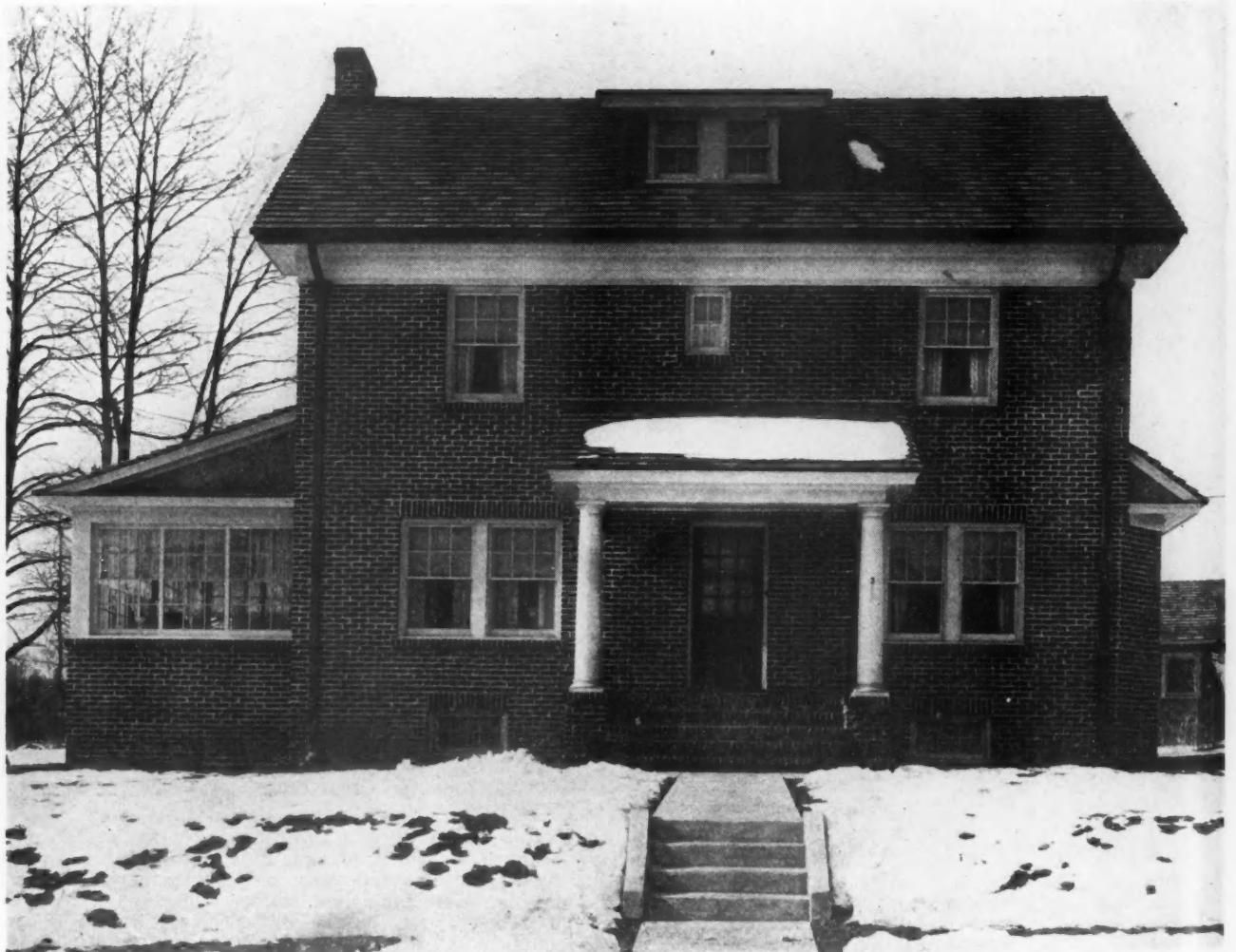
An Unusually Good Brick House Design, Size 26 by 36 Feet. The House Contains Seven Large Rooms Besides the Enclosed Sun Porch, and Has Many Attractive and Convenient Features.
