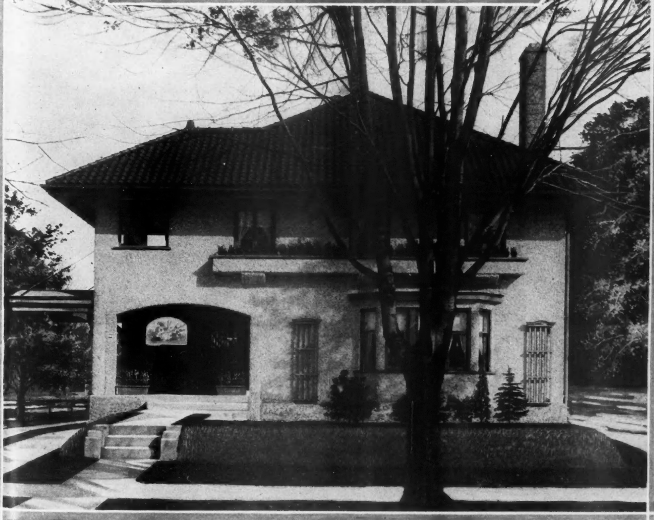
MODERN STUCCO HOUSE OF SEVEN ROOMS. This design for a stucco house contains the good features that are found in most modern homes. The broad entrance porch, with the enclosed sleeping porch above it, makes this a most distinctive home. The dimensions of the house are 34 by 34 feet. Large living and dining rooms and the kitchen are on the first floor, and four bedrooms, bath and sleeping porch on the second. At the rear of the first floor is a projection 7 by 23 feet, containing a breakfast porch, 6 feet 6 inches by 10 feet, the pantry and rear porch. All of the rooms are of good size and conveniently arranged. This is an excellent home building design for either the city or rural builder.
