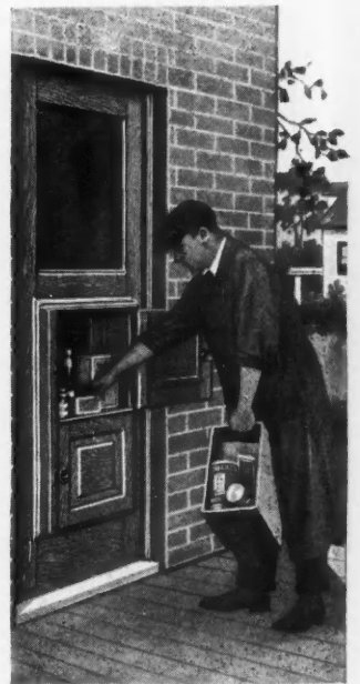
The Deliveryman Puts the Groceries in the Receiver and Shuts the Door, Which Automatically Locks and Unlocks the Inside Door.
