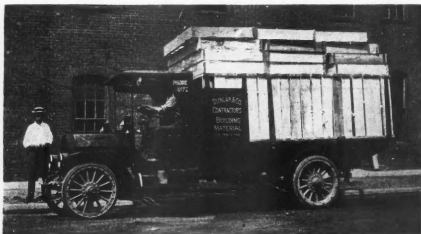
Light Indiana Truck Used by Dunlap & Co., Columbus, Ind., Starting Out with a Load of Sash. They Haul It to the Job When the Carpenters Are Ready.
