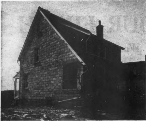
Another Type of Home Built in Destroyed Section. All These Houses Were Built with Vestibules, Which Were Found Necessary Because of the Climate of Nova Scotia. The Roof Is Slate.
