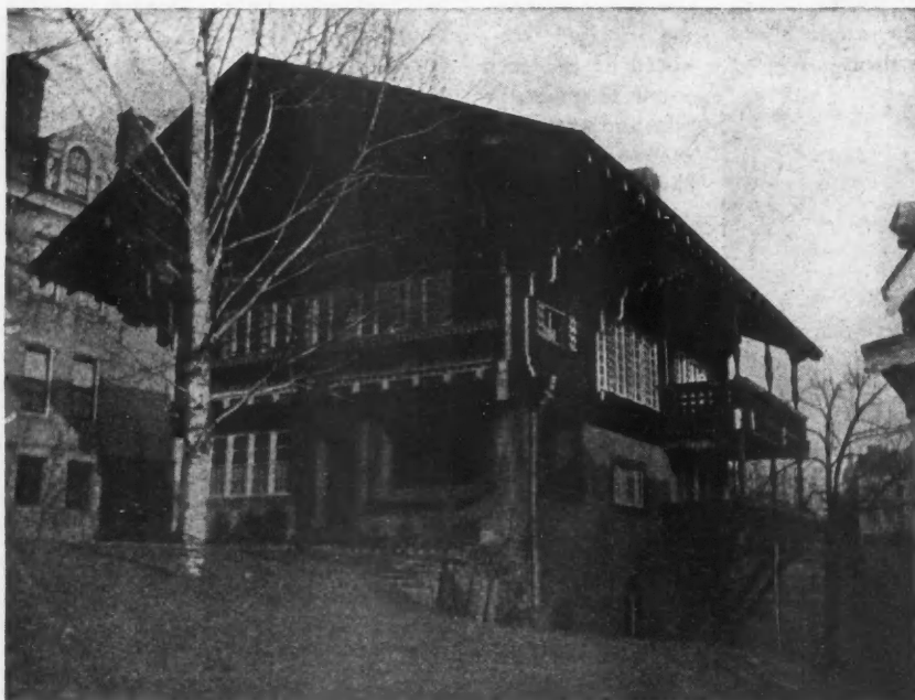
Swiss Chalet, Built by Albert Fisher, Cincinnati. Even Old-time Swiss Building Construction Was Employed, the Timbers Being Held Together with Oak Pegs, 3,000 of Them Being Required.
