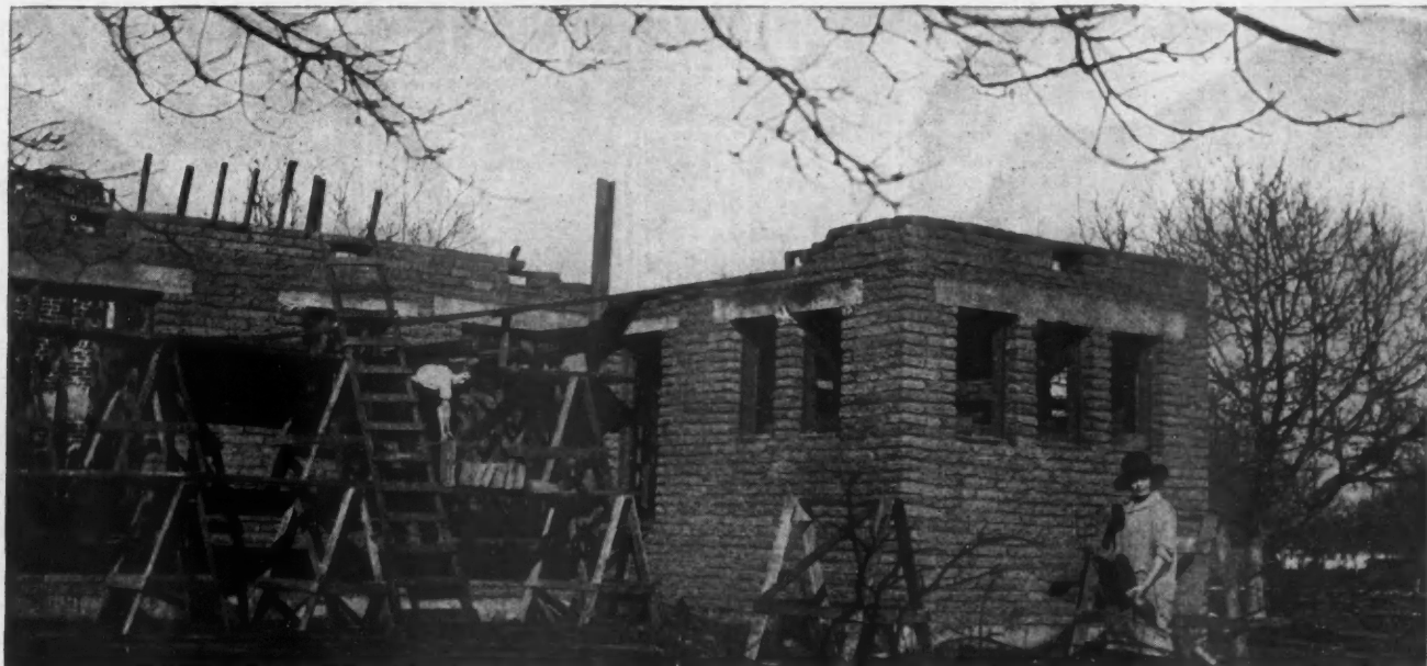
Building a Home of "Dobe" Brick. These Fair Artisans Are Solving Their Housing Problem by Using the Materials Which the Aztecs and Spanish Fathers Used Four Centuries Ago.
