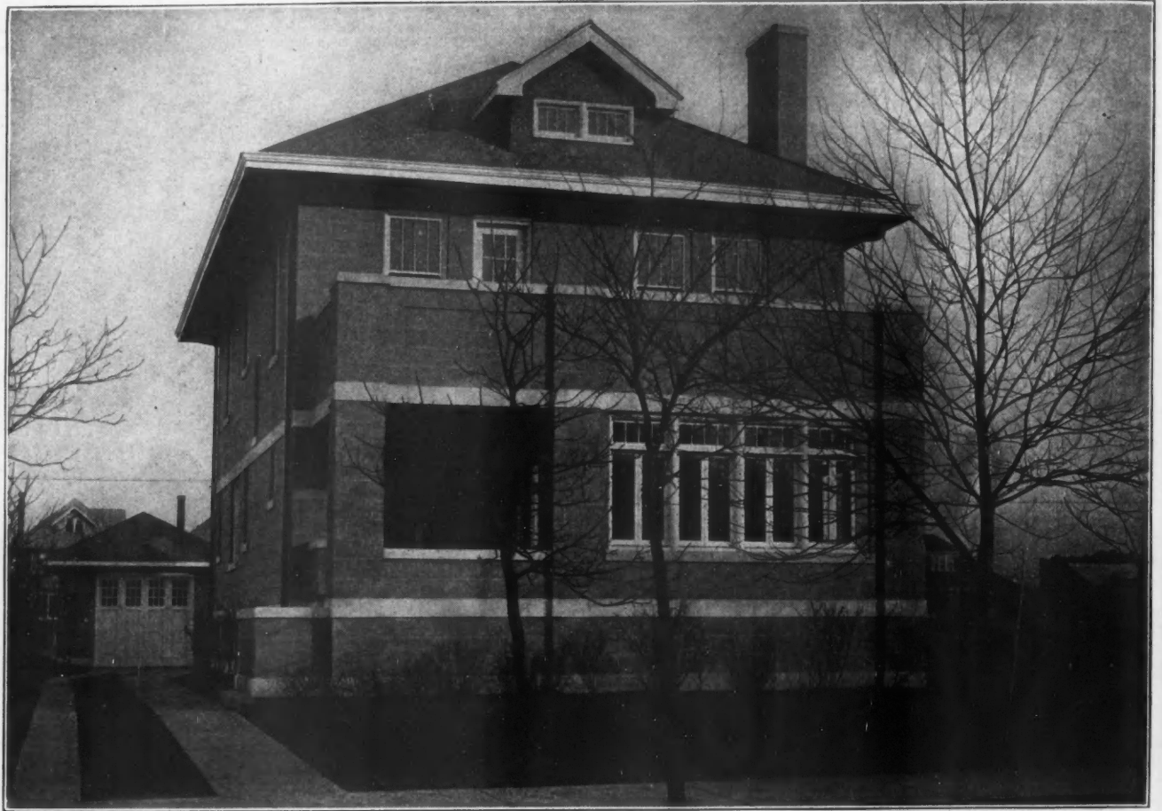
Concrete Block Residence and Garage Described in the Accompanying Article, in Which Smooth Surface Granite-Face Block Contrast Pleasingly with Dead White Trimstone.
