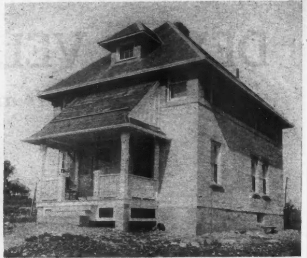
Attractive Six-Room Home with Slate Hip Roof. The Foundation Is Monolithic Concrete and the Exterior Has a Mottled Granite Effect. The Blocks Were Made Near the Scene of Construction.
