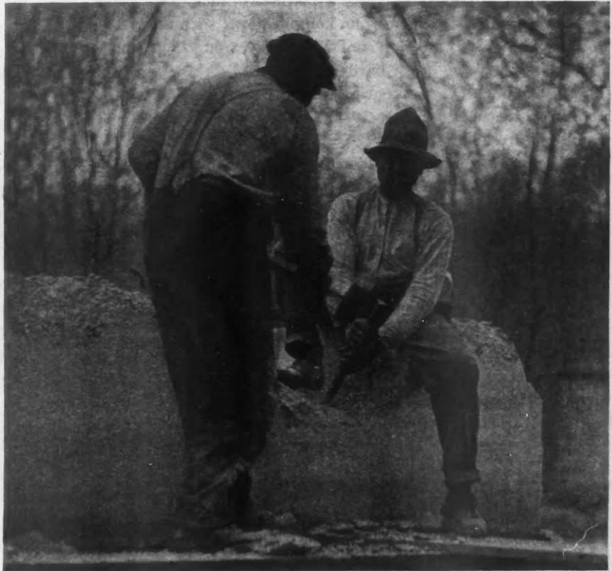
The Old Way. Razing a Concrete Foundation by Hand. It Is a Tedious Job, Costing Money and Causing Delay.
