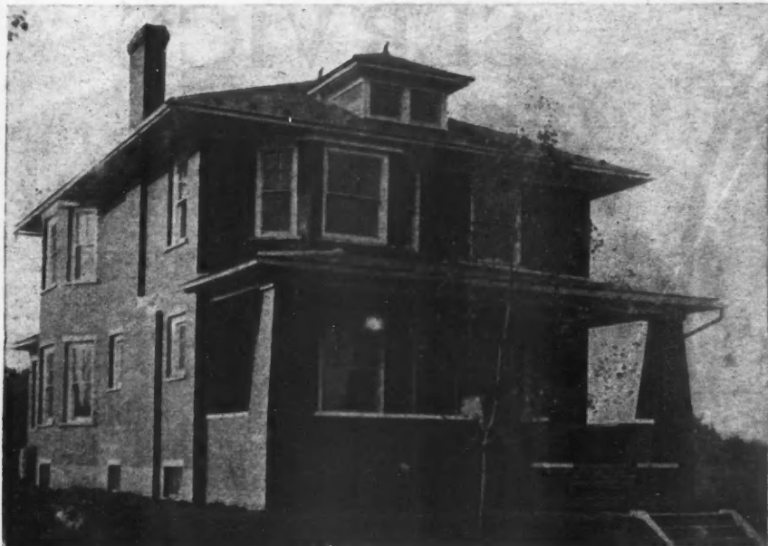
Front View of Hip Roof Brick House Built by Arnold Weissenloff, Contractor, in Easton, Pa. He Used Plans Which Were Published in the AMERICAN BUILDER.
