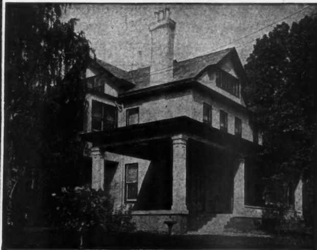
Residence of Arnold Kaishen, Cincinnati, Ohio An Old Wooden House Transformed into a Modern, Permanent Residence by Overcoating with Hy-Rib Lath and Stucco.
