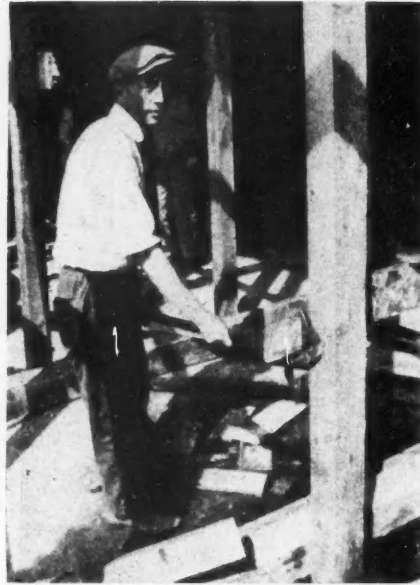
View Looking Toward Operator Showing How Device Fits Against Support and Board Which Is to Be Removed. It Can Be Used from Either Side of the Post.
