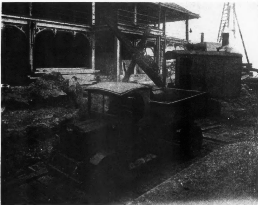
Excavating Work Requires Endurance and Power. This 5-Ton "Service" Truck Has Stood the Test by Making the Steep Grades up to Street Level for Many Months Without Rest.
