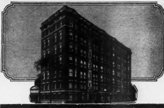
Equipped with Kernerator W. O. Goodman Apartment, Chicago William E. Walker, Architect
