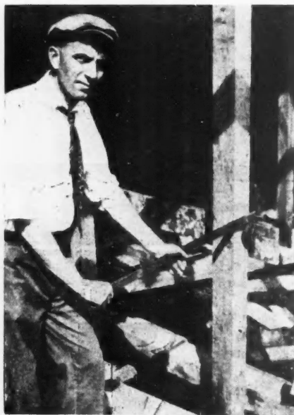
View of New Stripping Device for Removing Ledger Boards Without Damaging the Boards.
