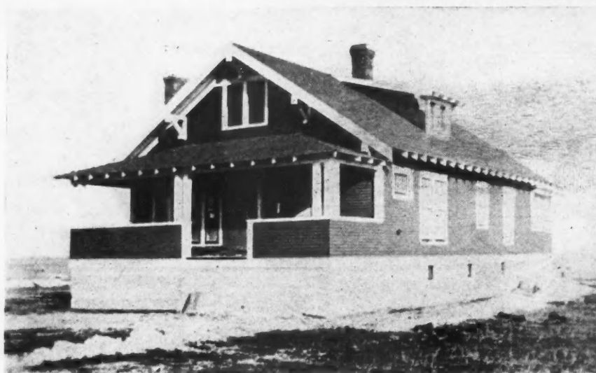
A Real Honeymoon Bungalow Built on an Idaho Ranch by Arthur H. Fay, Contractor, of Kimberley, Idaho. Among Its Many Features Are an Electric Lighting Plant, Water Supply System, and Hot Air Furnace. Mr. Fay Believes in Modern Equipment for Comfort.
