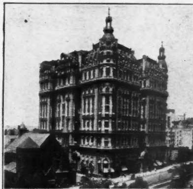
Hotel Ansonia, New York City: Warren & Wetmore, Architects; E. Smolka Plumbing Supply Co., Jobbers; James McCullagh, Plumber
