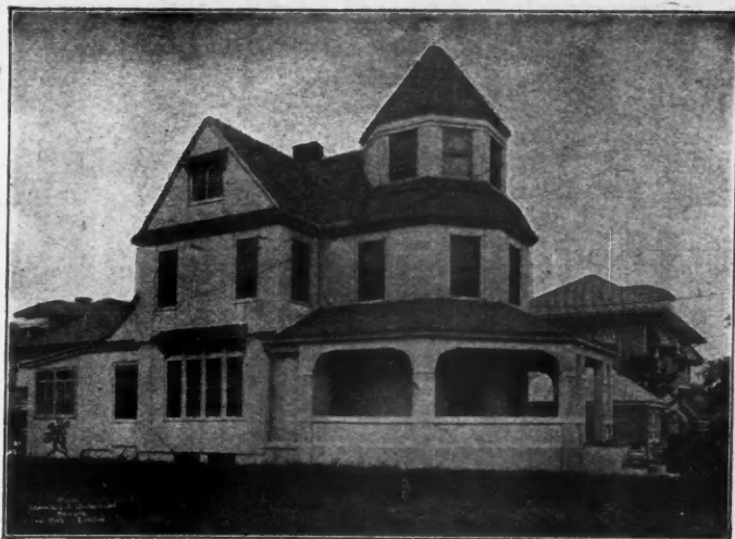
Radiant shingles over old wood shingles
