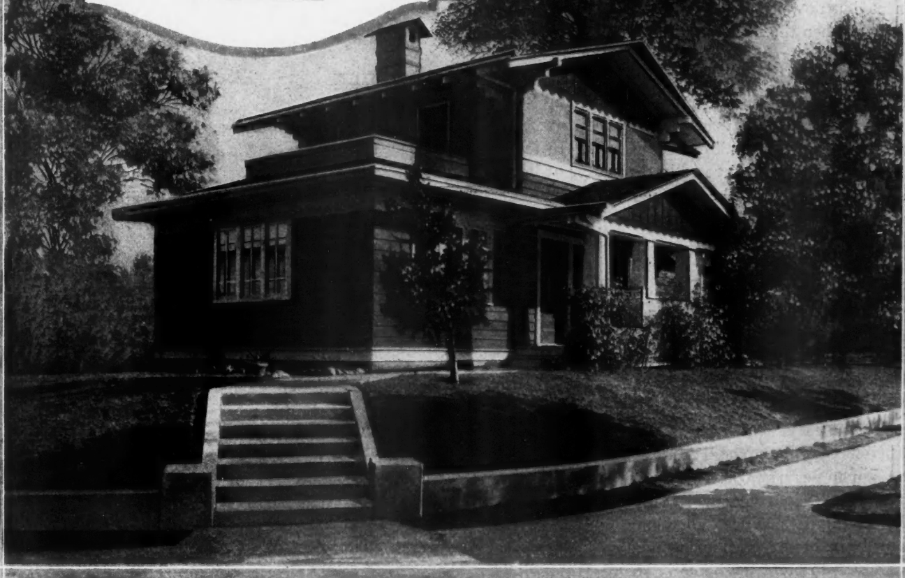
SIX-ROOM HOUSE OF UNUSUAL DESIGN. Here is home that will appeal very strongly to those who are seeking something different. Built along the so-called "airplane" lines which are so popular in the west, it has many features that tend to make it unique. The cupola effect of the second floor is one of these. At either end is a balcony covered with prepared canvas, a very popular flooring and roofing material. Two bedrooms are located on the second floor. On the lower floor are the living room, ample and comfortable dining room, bedroom and kitchen, also a sun parlor. The chimney has been well camouflaged to conform to the general design of the dwelling. The exterior is frame and stucco. 24 by 52 feet are the dimensions.
