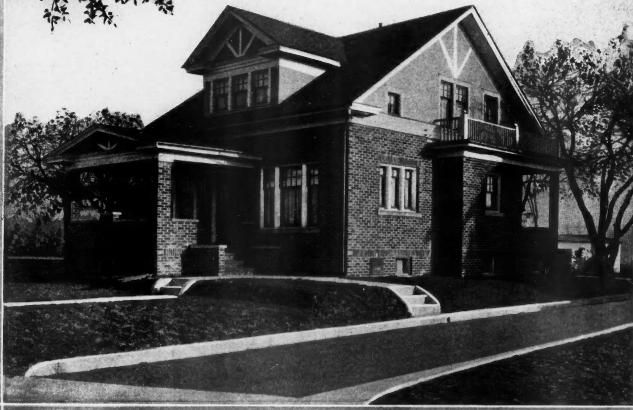
SUBSTANTIAL STORY-AND-A-HALF HOME. This type of dwelling continues to hold its popularity because of its convenience for a medium-sized family. Built of brick with stucco on the half story, it is unusually substantial and well designed. The roof has been covered with asbestos shingles similar to those shown in detail on the opposite page. This home contains seven rooms, four on the first floor and three upstairs. The front entrance opens directly into the living room which is well lighted by a triple window facing the porch and a bay on the side. The dining room, kitchen and wash room make up the remainder of the lower floor. The bedrooms, three in number, are above. Two of them are very comfortable being 16 feet 6 inches by 10 feet 6 inches and 10 feet. The house is 30 by 32 feet.
