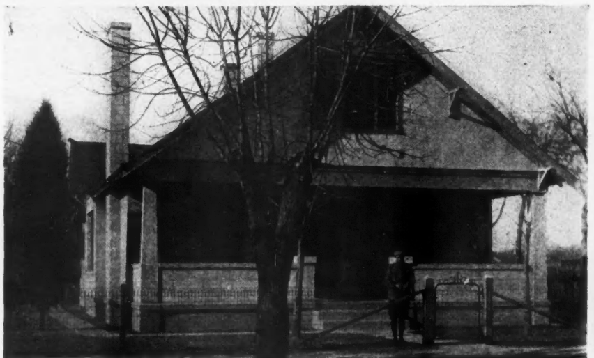
Figure 1.—Attractive Cottage at Pueblo, Colo. Walls and Chimney Construction Are of Smooth Granite-face Concrete Block. One of the "Home Product" Houses Erected by the Granitoid Construction Company.
