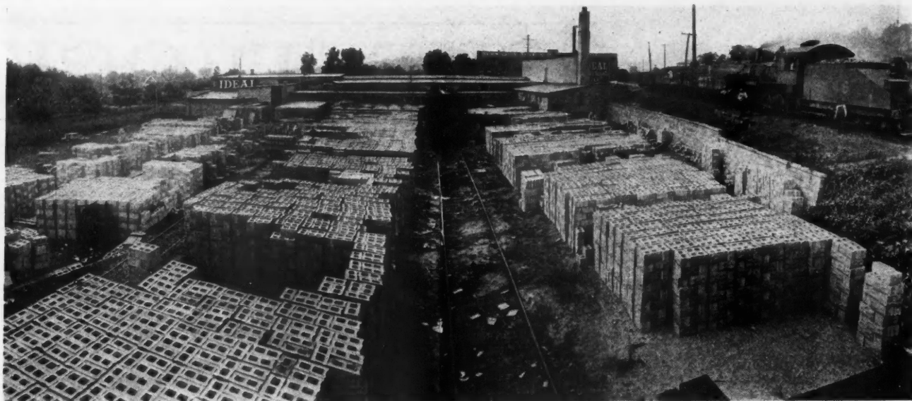
View of Shipping Yard of Concrete Block Concern. Last Year They Shipped 1,015,000 Blocks. The Daily Requirements Are 150 Tons of Sand and 600 Sacks of Cement. This Firm Has Established an Excellent Reputation in that Section of the Country.
