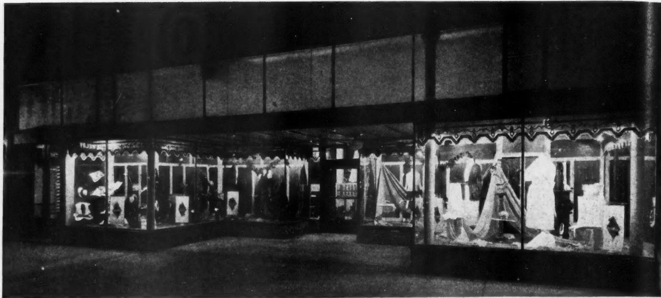
How the Stores Looked After Being Remodeled. The Value of This Window Space as Advertising Is Incalculable to the Owner of the Store. Many Builders Make a Specialty of Installing New Store Fronts in Old Buildings. This Store Is Owned by the McKinney Clothing Co., Durango, Colo.
