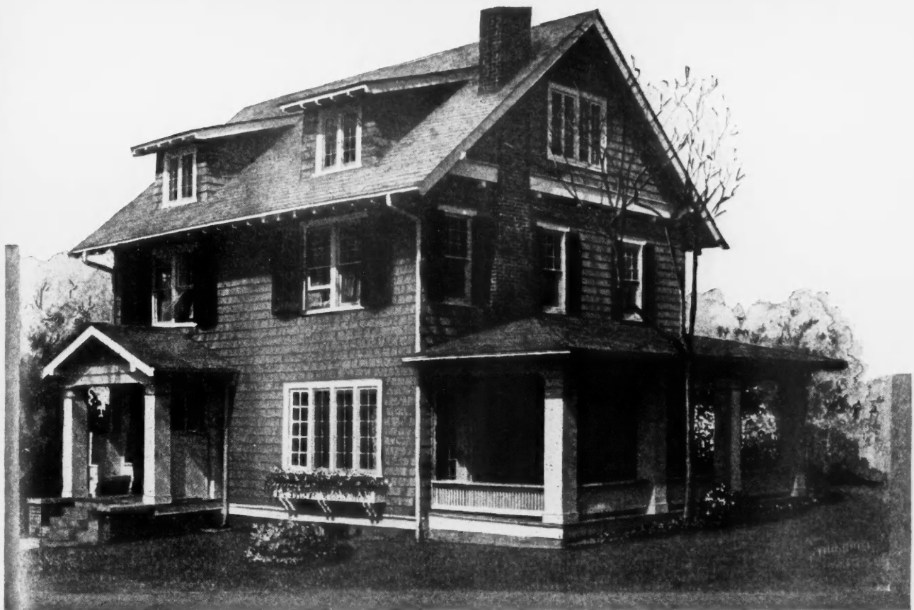
COMFORTABLE SEVEN-ROOM HOME OF PLEASING DESIGN. There is a quaintness and simplicity about this house that is bound to attract many homeseekers. It has an attractive exterior with shingle siding, broad front porch and hospitable side hooded entrance. In its small, well placed roof dormers, small paned windows, shutters and entrances it shows decided Colonial influence. Because of its rectangular shape it is an economical house to build. On the first floor are the large living room, 18 feet 6 inches by 13 feet 3 inches with open brick fireplace, dining room well lighted by two sets of four casement windows each, and kitchen. There is also a washroom adjoining the kitchen. On the upper floor are four bedrooms of comfortable size with ample closet space. The house is 30 feet wide and 28 feet long.
