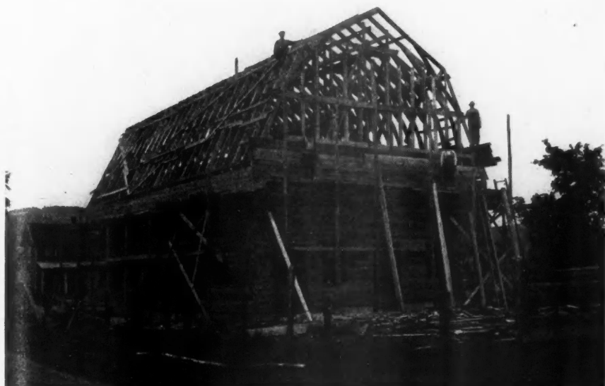
W. A. Van Luvancee, Athens, Pa., Built This Barn from Plans Shown in the American Builder. Only Four Men Were Needed to Raise the Roof.
