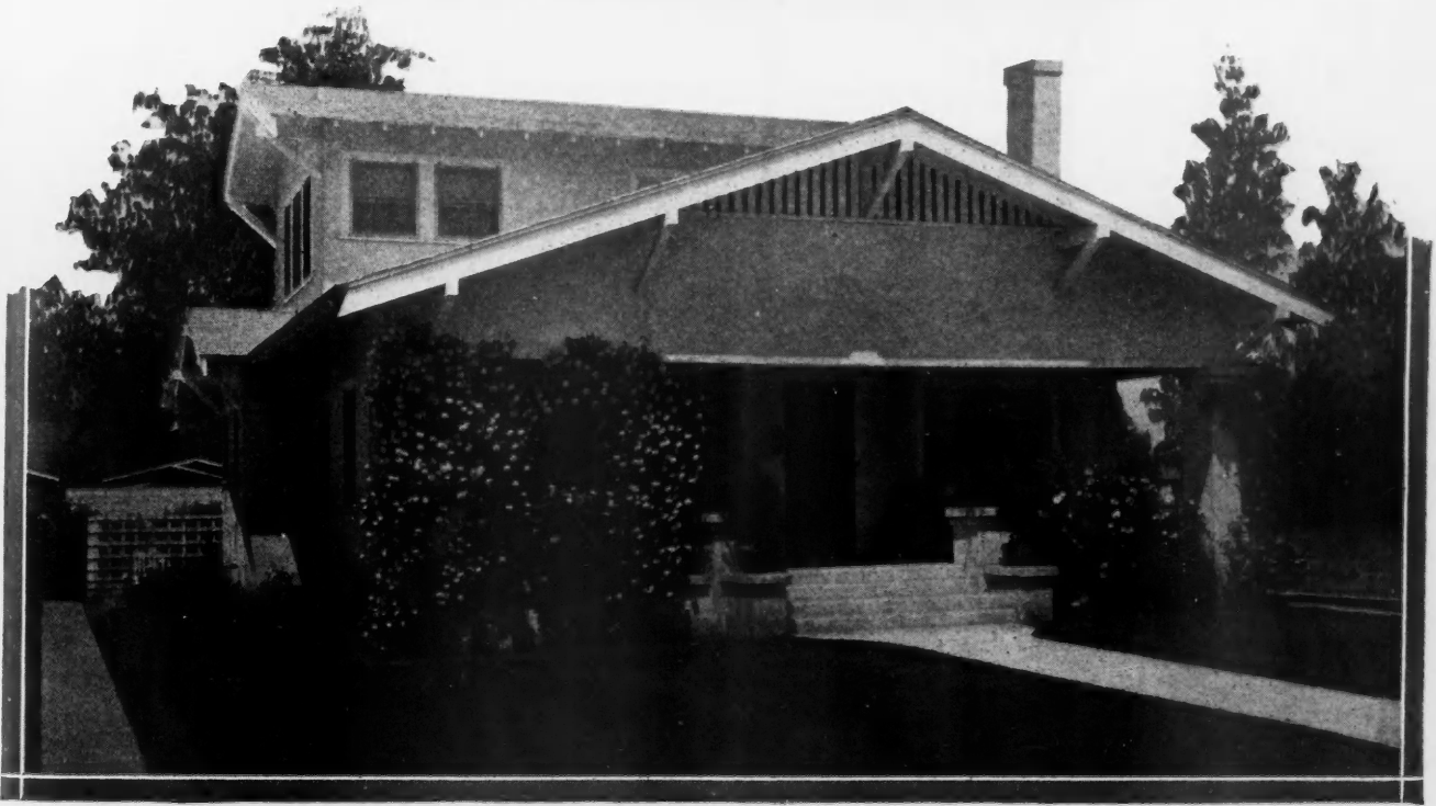
“AIRPLANE” BUNGALOW DESIGN OF QUALITY AND APPEAL. In this age of airplanes, the effect is readily seen in more than one branch of endeavor. That perhaps accounts for its influence on architecture and the introduction of the so-called “airplane” bungalow. Here is a design of this type, a stucco structure of eight rooms, two of which form the upper deck which gives cause for the name. These upper rooms are bedrooms and are usually converted into sleeping porches in the summer time, having exposure on three sides. On the first floor are six rooms, conveniently grouped with sleeping rooms separated from the living rooms by a hall. The living room and dining room are both bright and cheerful rooms of good size. A library is also provided. This home is 29 by 43 feet.
