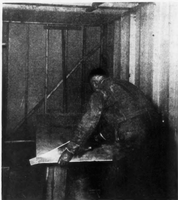
Wallboard Can Be Sawed and Nailed Like Lumber. This Man Is Using an Ordinary Cross-Cut Saw.
