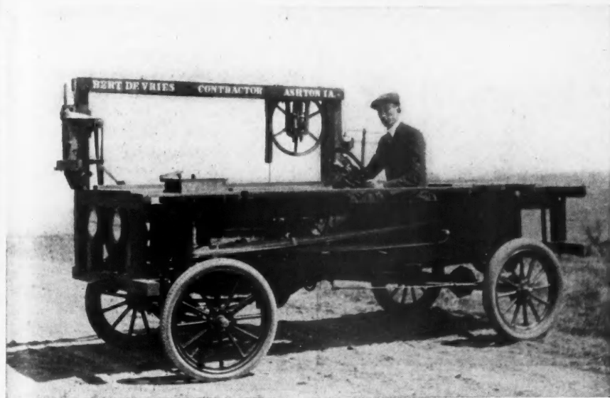
Bert De Vries, Builder and Contractor, Ashton, Iowa, Has Rigged Up a Very Unique Portable Saw Rig on a Ford Car. The Car Engine Furnishes Power to Run the Saw Rig which Contains Complete Equipment.
