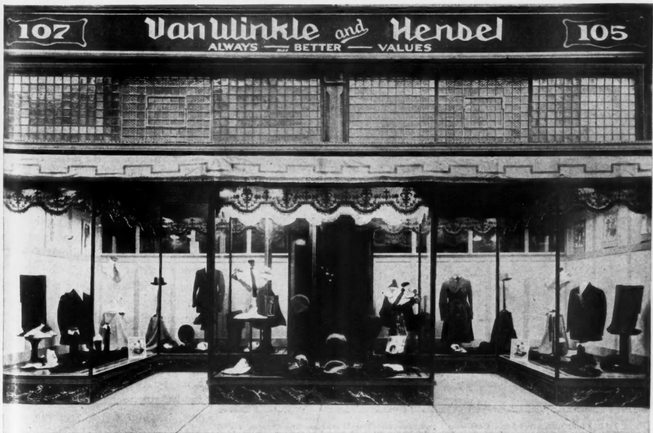
After—Contractor F. J. Nafziger Had Recognized the Value of Store Front Remodeling Work and When These Merchants Consulted Him on a Job He Was Ready to Handle it. Here Is the Result. A Real Window Display That Has Proved a Magnet in Getting Business.
