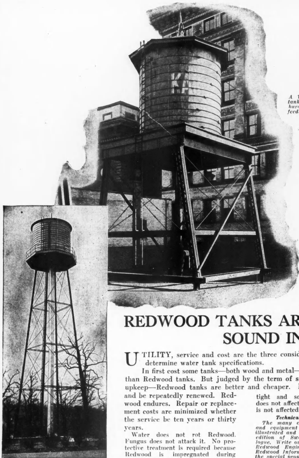
A 30,000 gallon water tank of 3" Redwood. Installed at the Pittsburgh Field Club for club house water system, watering the greens and supplying water for swimming pool.
