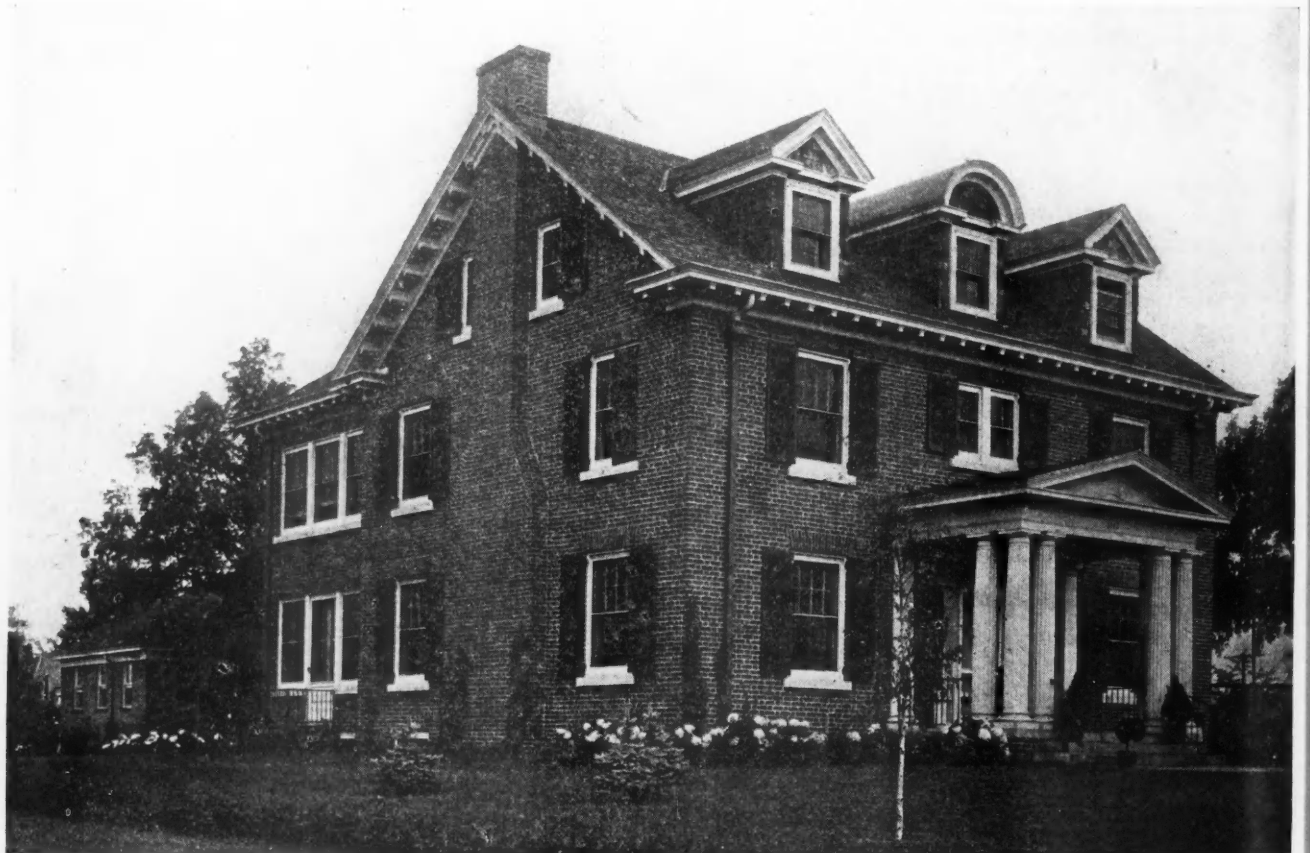
Pretentious Home of Very Charming Colonial Design. It Contains Seven Unusually Large and Comfortable Rooms and Sleeping Porch in Rear 19 by 14 Feet. It Is Built of Brick and Is 38 Feet Wide and 42 Feet 6 Inches Long, Including Rear Wing. A Brick Garage Is in the Rear.
