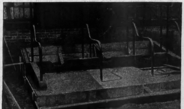
Fig. 6. Concrete Is Then Placed for the Manger. A 1:2:3 Mixture Is Recommended.
