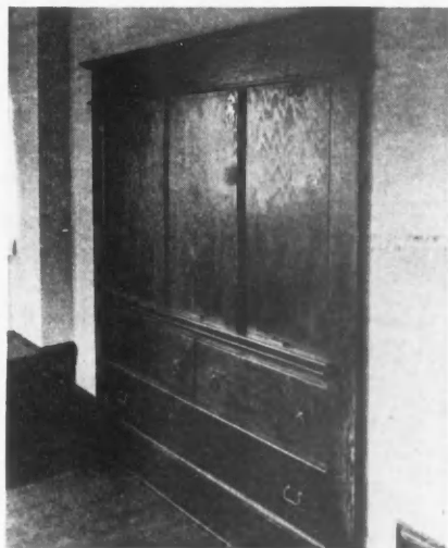
Built-in Sewing Cabinet for Small Home. This Handy Device Will Save Considerable Space.
