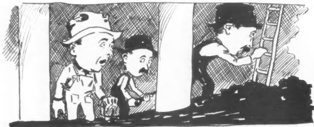
The Contractors Were Making Excavations Around the Piers when They Struck Quicksand.
