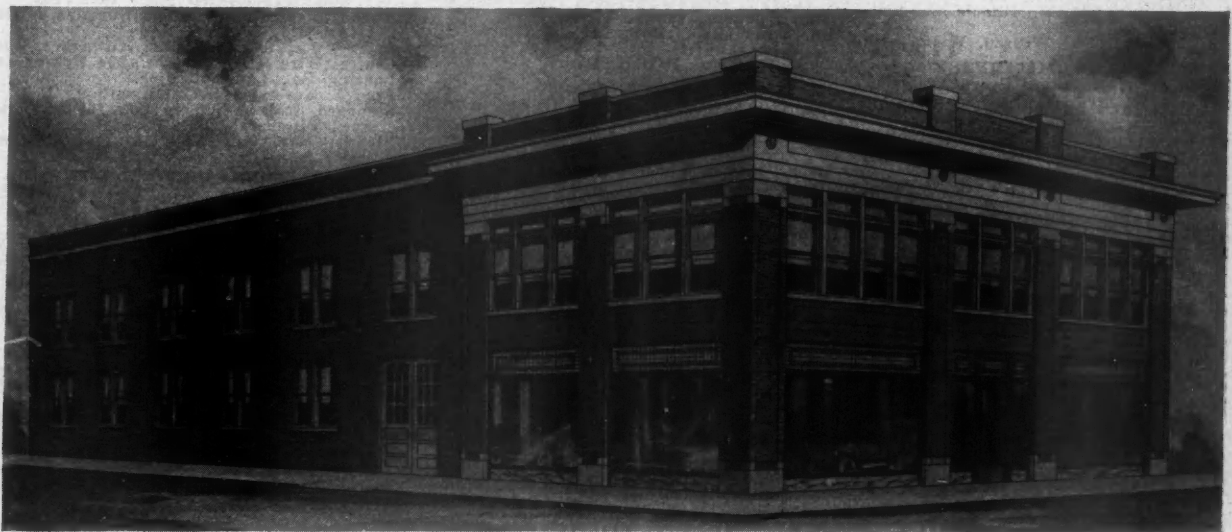
MODERN TWO-STORY GARAGE DESIGNED BY OUR ENGINEERING DEPARTMENT
