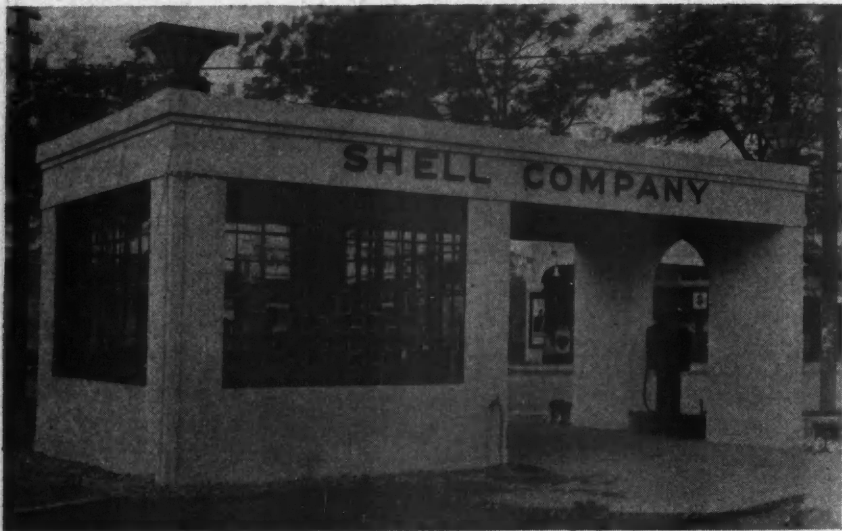
Gas Filling Station Which Has a Daylight Interior Afforded by Steel Sash Walls. Many School Houses Are Equipped with This Type of Window.
