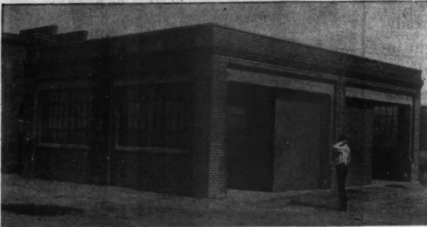
Small Brick Garage Equipped with Steel Sash and Ventilators. This Type of Sash Is Being Used in Many Buildings of This Type.
