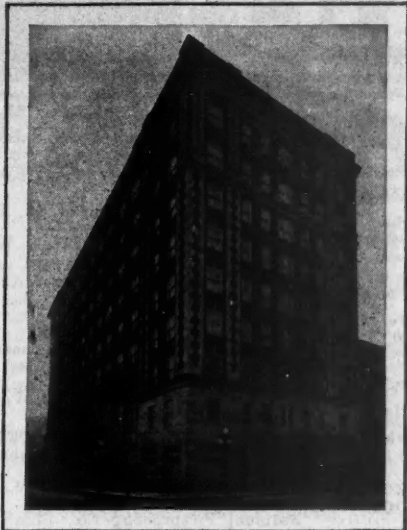
The Fort Steuben Hotel, Steubenville, Ohio: Frederic Webber, Philadelphia, Architect; J. D. Johnson Co., Inc., Philadelphia, Jobbers; Modern Plumbing & Heating Co., Philadelphia, Plumbers
