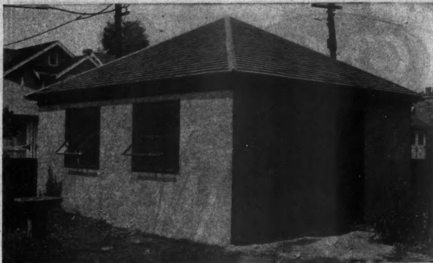
Small Private Garage Equipped with Pivoted Steel Sash Windows. Heretofore This Construction Has Been Confined to Factory Buildings.
