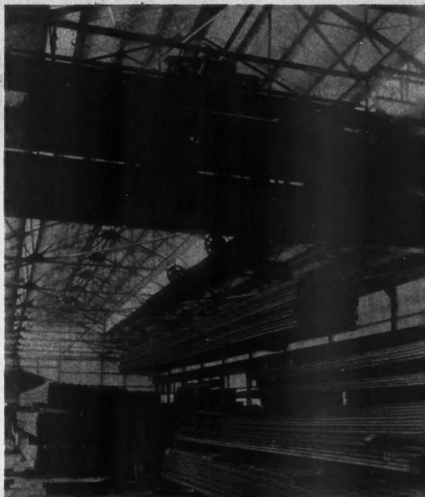
Electric Crane Handling Steel Joist Sections at Mill.
