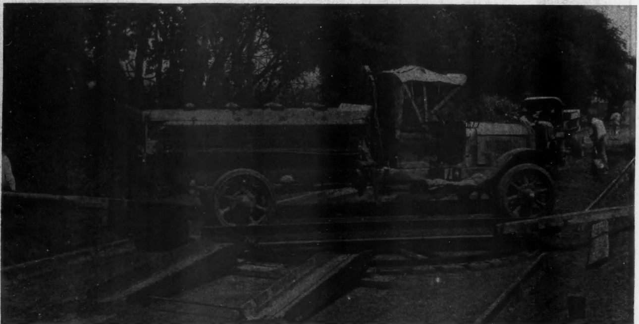
Six 3½-Ton Republic Trucks Like the One Shown Here Were Instrumental in Speeding Up the Work on a Six-Mile Concrete Paving Job Near Wichita, Kans.
