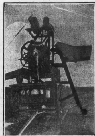
Mixer raised— track extended to charge mixer on same level with material piles.
