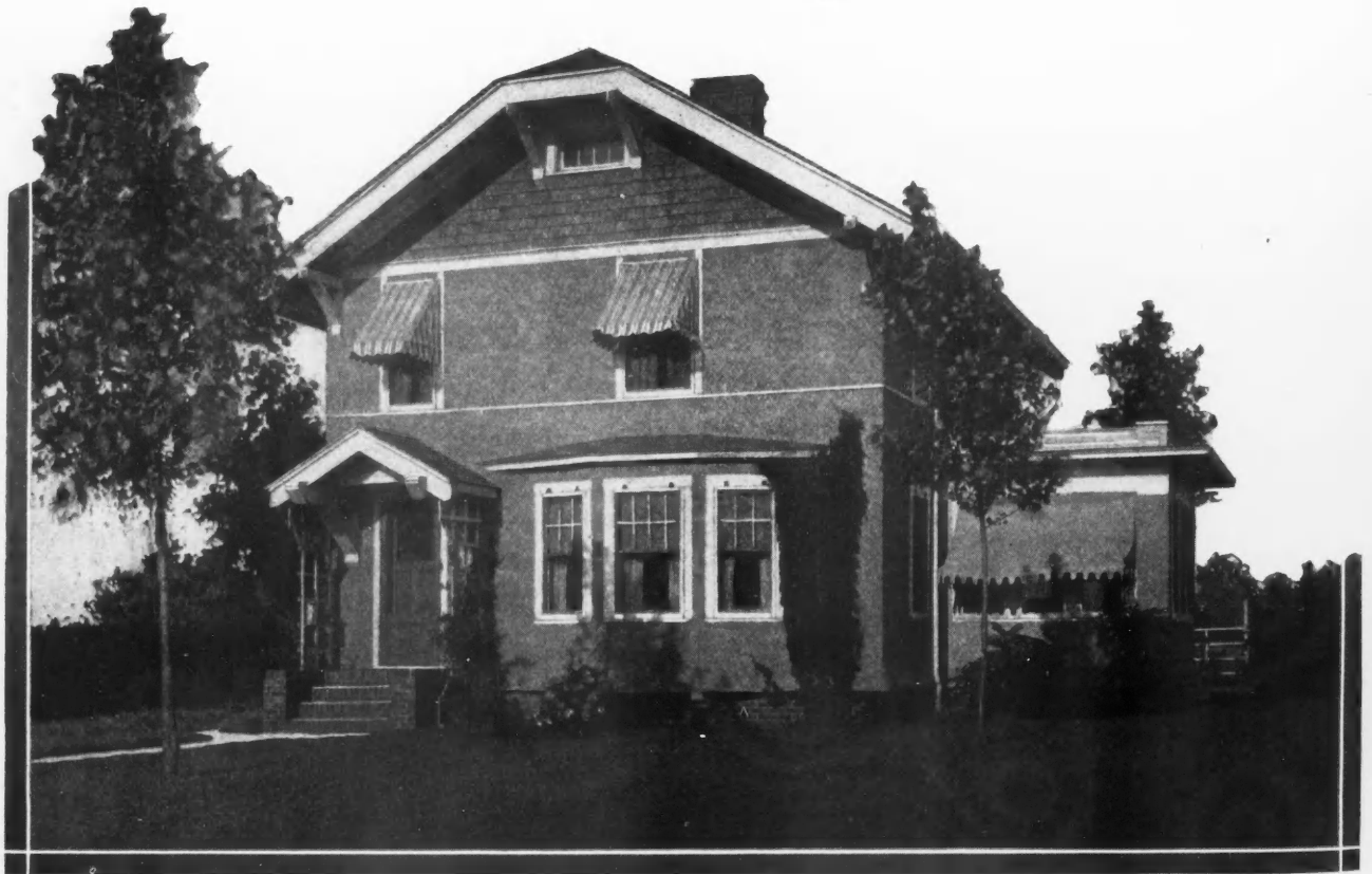
DISTINCTIVE, ECONOMICAL HOUSE DESIGN. Here is shown the familiar square-shaped house with slight variations in roof and entrance that give a little individuality that is helpful. There is also a side sun parlor which adds much to the convenience and comfort of the house. The front entrance, of simple yet dignified and inviting bearing, is set to one side to make way for a bay window in the large living room. The steps are brick, as is the foundation, while the main part of the house is stucco with just a touch of shingles under the eaves. Six large, comfortable rooms, sun parlor, 9 feet 6 inches by 15 feet, and sewing room upstairs are provided for in the floor plans. Living room, dining room, and kitchen are on the first floor, while the bedrooms are upstairs. The house is 24 feet wide and 30 feet long.
