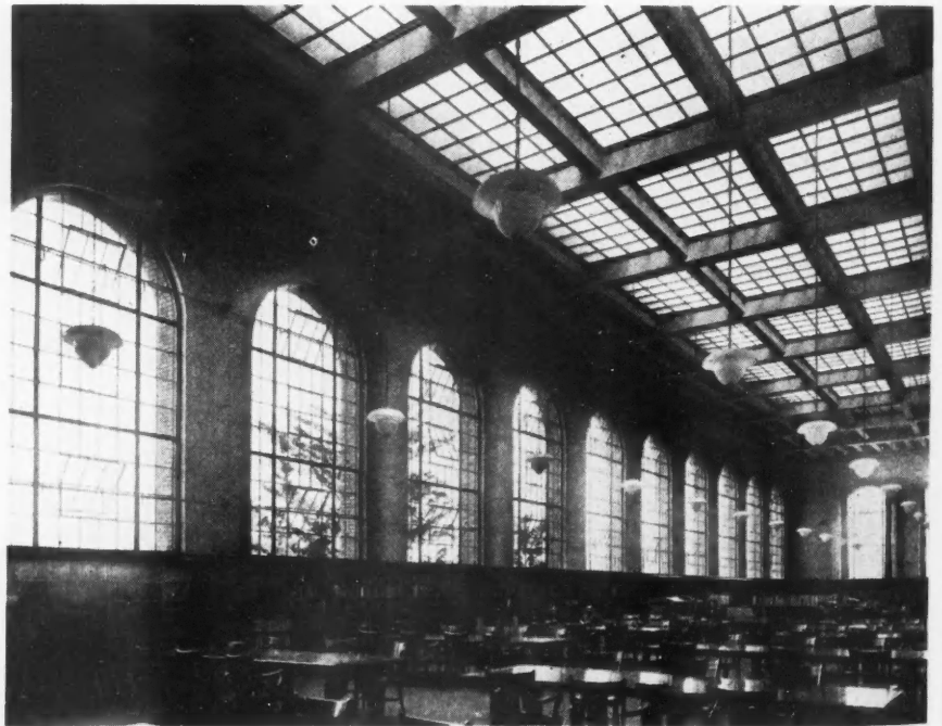
Library of Leland Stanford University, Palo Alto, Cal., Equipped Thruout with Steel Sash. Note the Wonderful Lighting Effect from Side and Ceiling.
