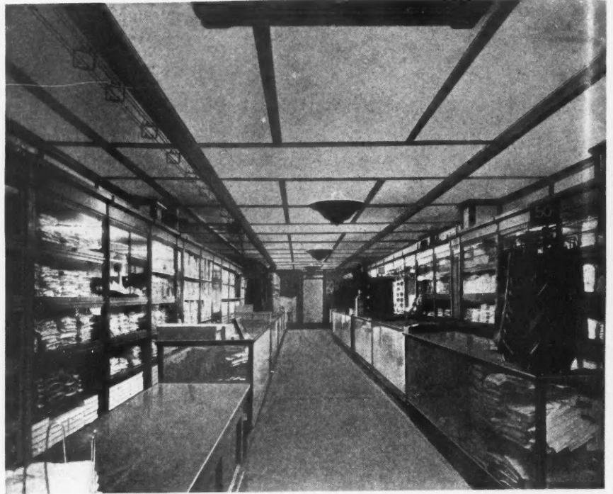
Store of H. B. Moore, Buffalo, N.Y., Finished with Wallboard. The Simplicity of the Design Is Very Effective and of Course Economical.
