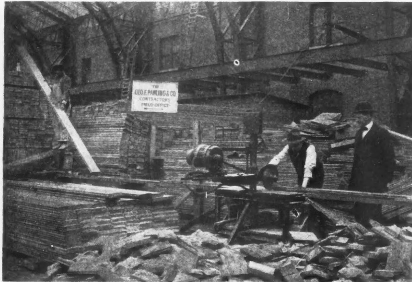
Woodworker on the Job. One of the Many Uses of This Labor-Saving Device. Here the Man Is Sawing Lumber for Rough Concrete Forms.
