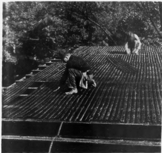
Placing Metal Lath Over Steel Joists in Ohio Store Building.
