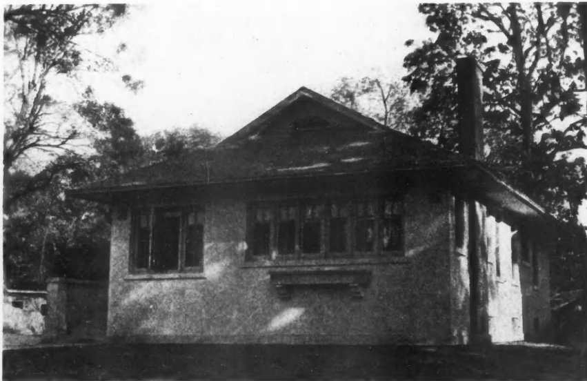
Fig. 2. Bungalow of Concrete Block and Stucco Construction, of Which Fig. 1 is a Wall Detail Before the Stucco Was Applied. Only Two Coats—a Scratch Coat and a Finish Coat—Are Required on the Average Concrete Block Surface.
