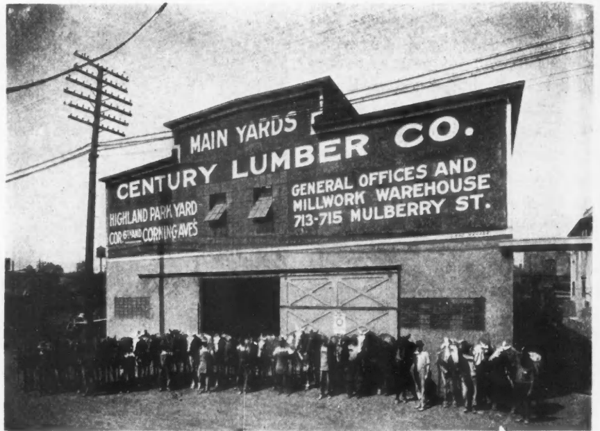
Main Yards of Century Lumber Co. This Building Is 505 Feet Long and Has a Capacity of 6,000,000 Feet. It Is Built of Concrete and Steel and Is Three Stories High.
