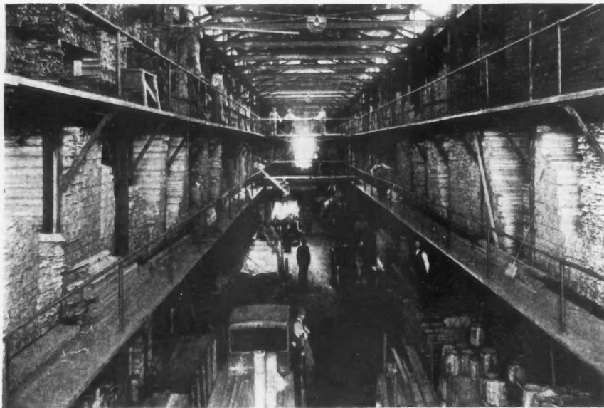
Interior View of Large Warehouse of Century Lumber Company. There are Three Tiers of Lumber. Trucks Can Drive Up to the Bin and Be Loaded Without Delay.
