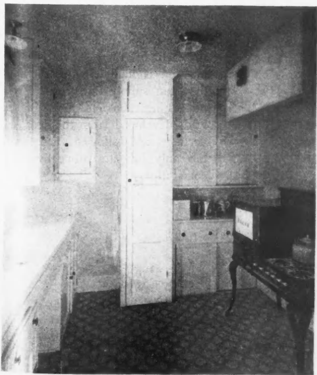
Broom Closet and Other Space Saving Features in Modern Kitchen. Note the Hood Over Stove to Keep Dirt and Gases from Spoiling Kitchen Walls.
