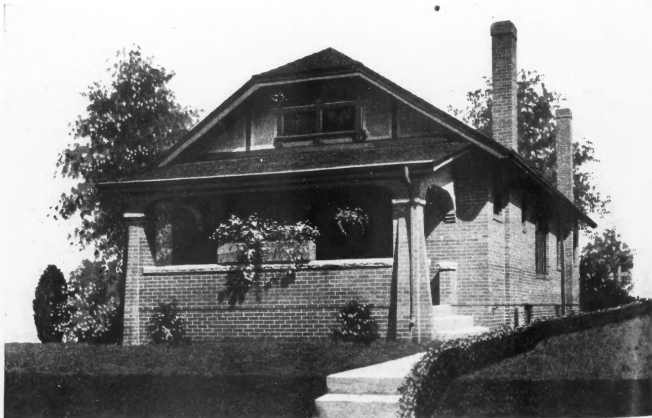
Well-Built Brick Bungalow of Five Rooms and Sleeping Porch. The Large Front Porch with Its Substantial Brick Pillars and Banisters Is a Practical Feature That Will Appeal to Most Families.
