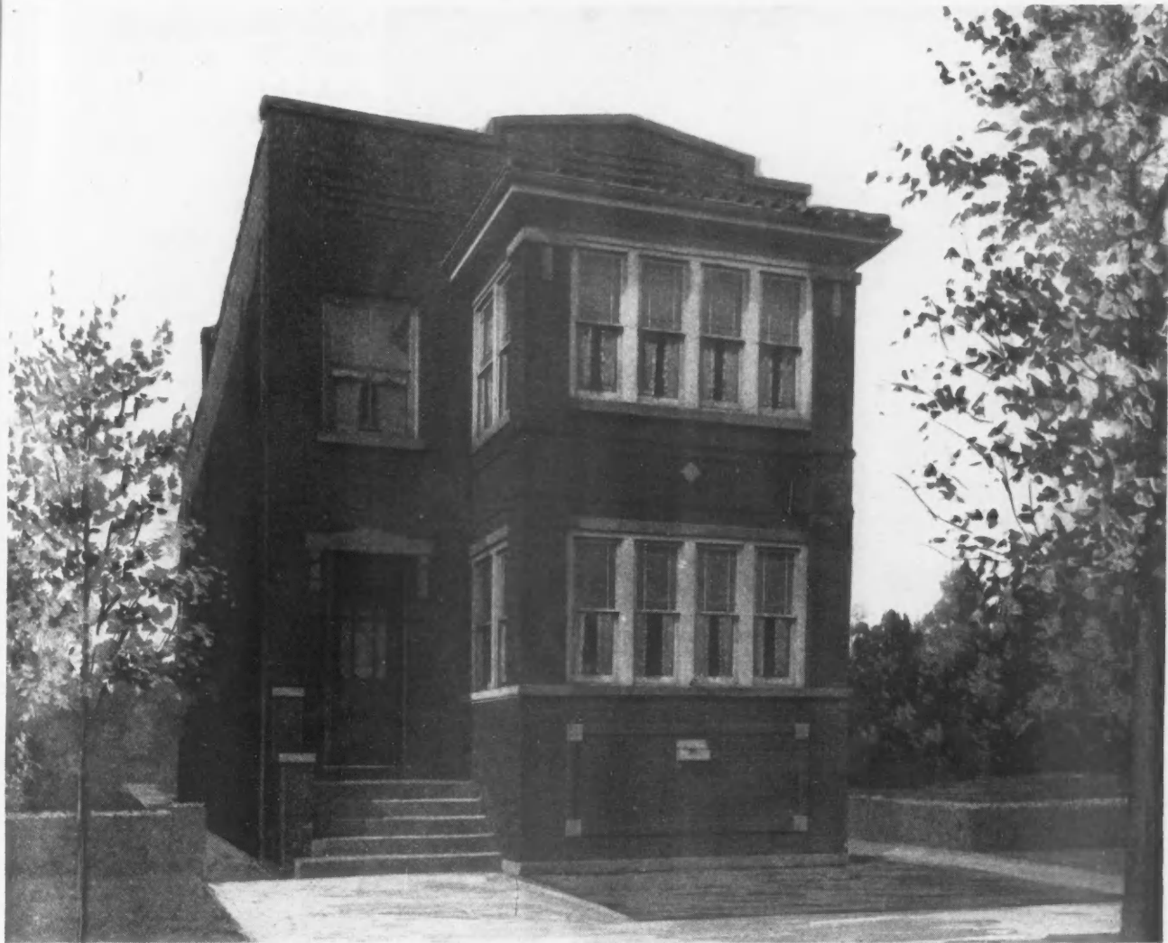
Typical Two-Apartment Building, Viewed with Favor by the Majority of Home-Seeking Public of Moderate Means. Note the Two Large Sun Parlors, Sturdy Brick Walls and High Basement. Each Apartment Has Five Rooms. Size, 24 by 49 Feet.
