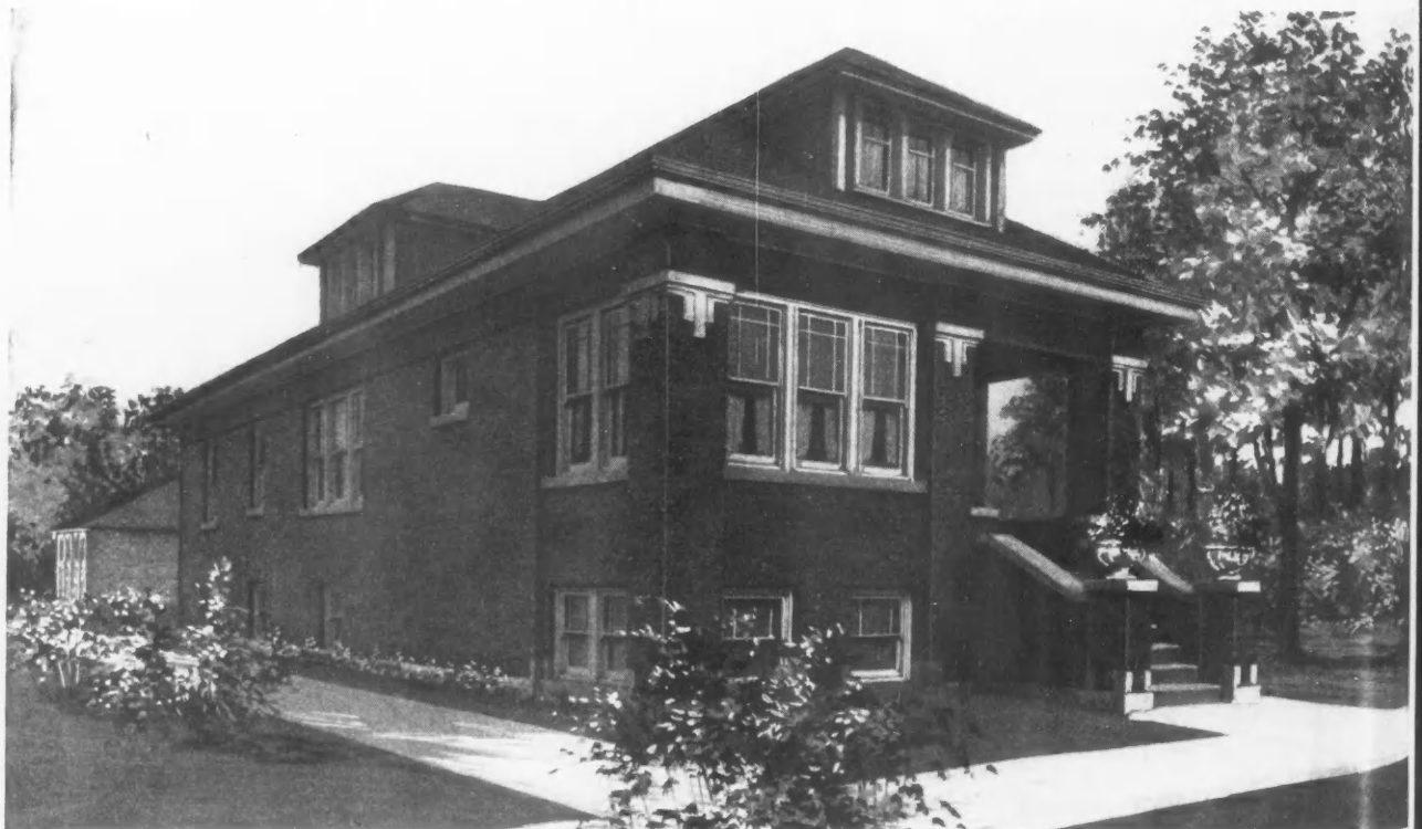
Attractive and Practical Brick Bungalow Design Which Is Being Built in Large Numbers in Most Cities. It Offers a Permanent Home of Five Rooms and All Modern Comforts. This House Is 24 Feet Wide and 43 Feet Long.
