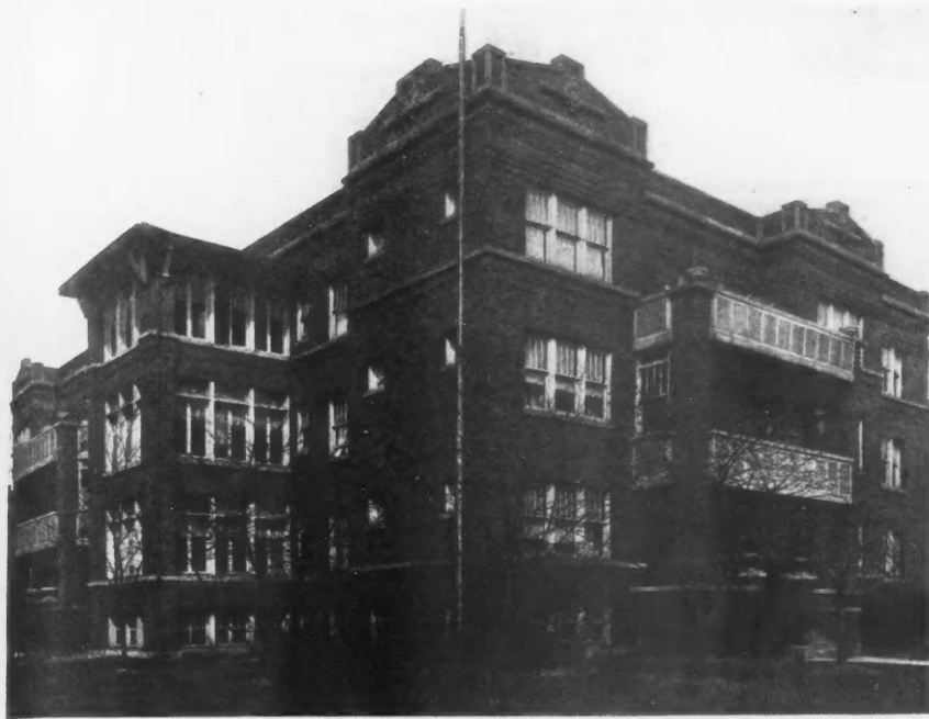
Five-Room Apartments Seem to Be the Popular Unit in the Co-Op Apartment Ownership Plan. A Yearly Budget Takes Care of the Operating Expenses and Each Owner Pays His Share.
