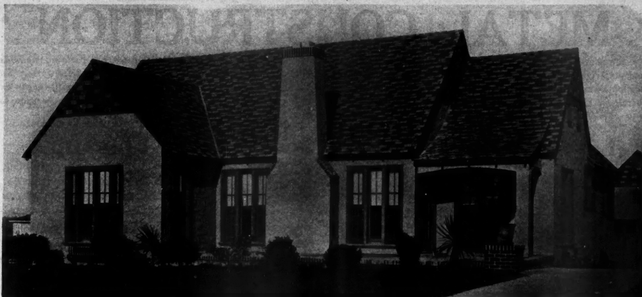
The Variegated Asphalt Shingle Roof, Showing Tapestry or Blended Effect Produced by Using Red, Green or Black Shingles in Combination. This Attractive Color Scheme Does Away with the Flat Monotony of the Ordinary Roof.
