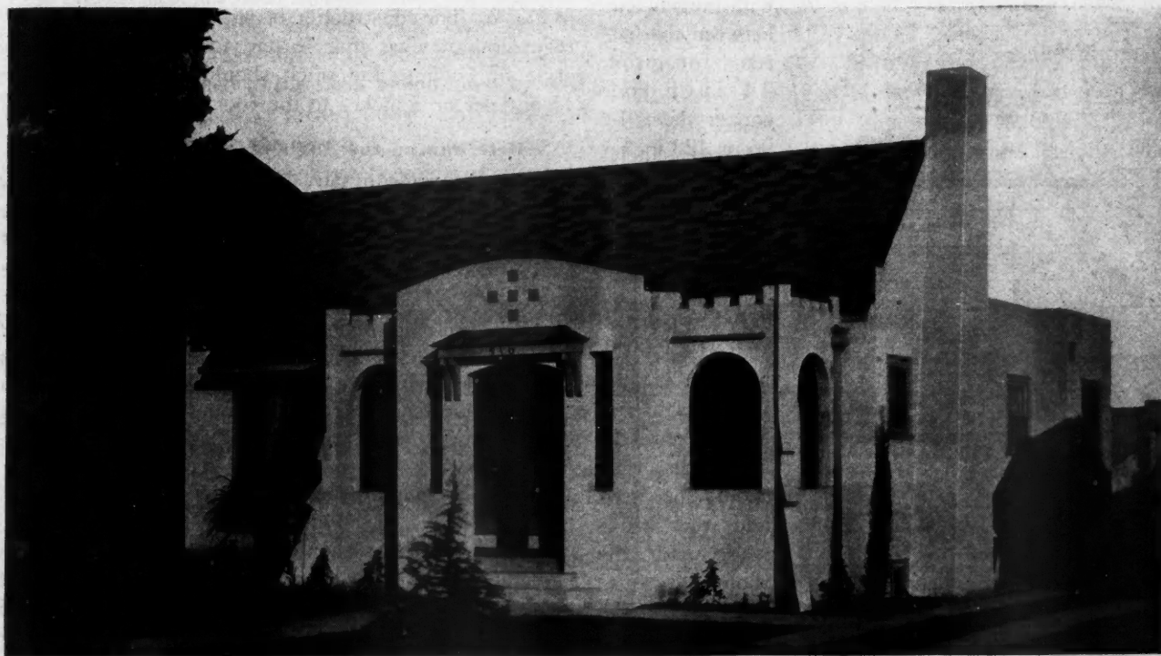
Another Striking Example of the Variegated Roof. In Laying This Roof Care Must Be Taken to Avoid a Definite Pattern. The Shingles Are Thoroughly Mixed and the Roofer Simply Lays Different Colors on the Same Course.
