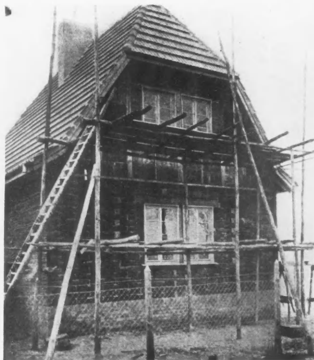
The Shortage of Homes in Berlin is Almost as Great as it is in this Country, Except That Here We Have Greater Resources for Construction. The High Cost of Building Materials Has Compelled Builders to Use Empty Cartridge Boxes, Filled with Mud and Put Together, Completing What is Known as an "Ersatz," One of Which is Pictured Here.
