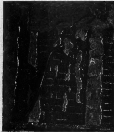
Fig. 1. Section of Brick Wall Over Which an Attempt Has Been Made to Apply a Surface Coat of Plaster Where There Was a Slow Seepage of Water.
