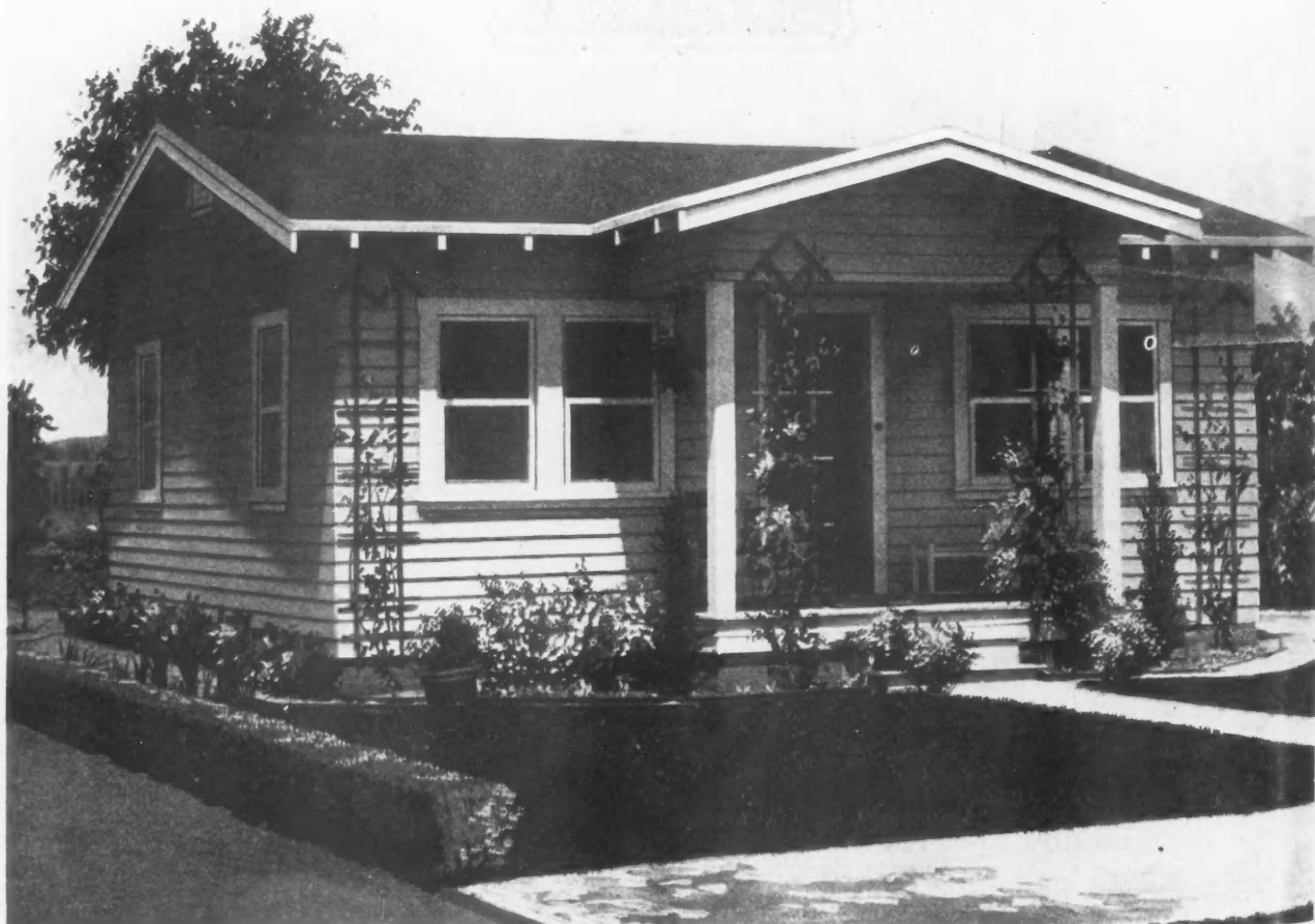
Three-room Bungalowette, 24 by 16 Feet, With Rear Wing for Kitchen and Bathroom. A Cozy Little Home That Can Be Built for Small Amount—A Home That Will Accommodate Family of Five in Modest Comfort.
