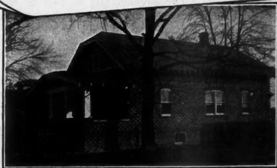
The Ideal All-Rolok Wall is laid in the attractive Flemish bond and is just as good looking as it is substantial.
