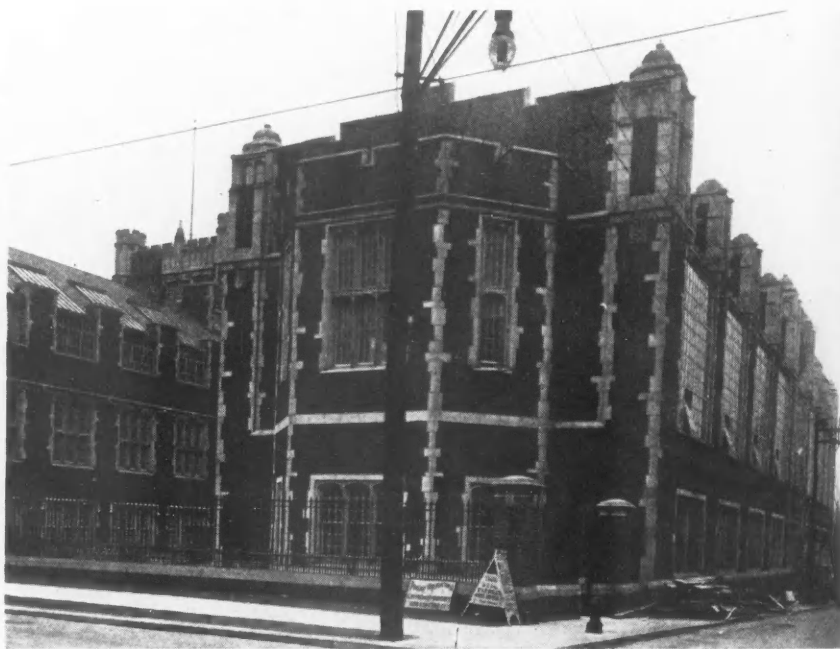
Newly Completed Evans Museum and Dental Institute, University of Pennsylvania, Philadelphia, Pa., Equipped with Special Steel Sash. Note the Adaptation of This Style of Sash to the Architectural Scheme.
