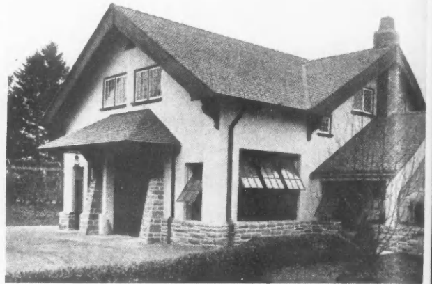
Garage of T. T. Watson, Wayne, Pa., with Steel Sash. There is the Balanced Ventilator Type Used Frequently in Smaller Buildings.
