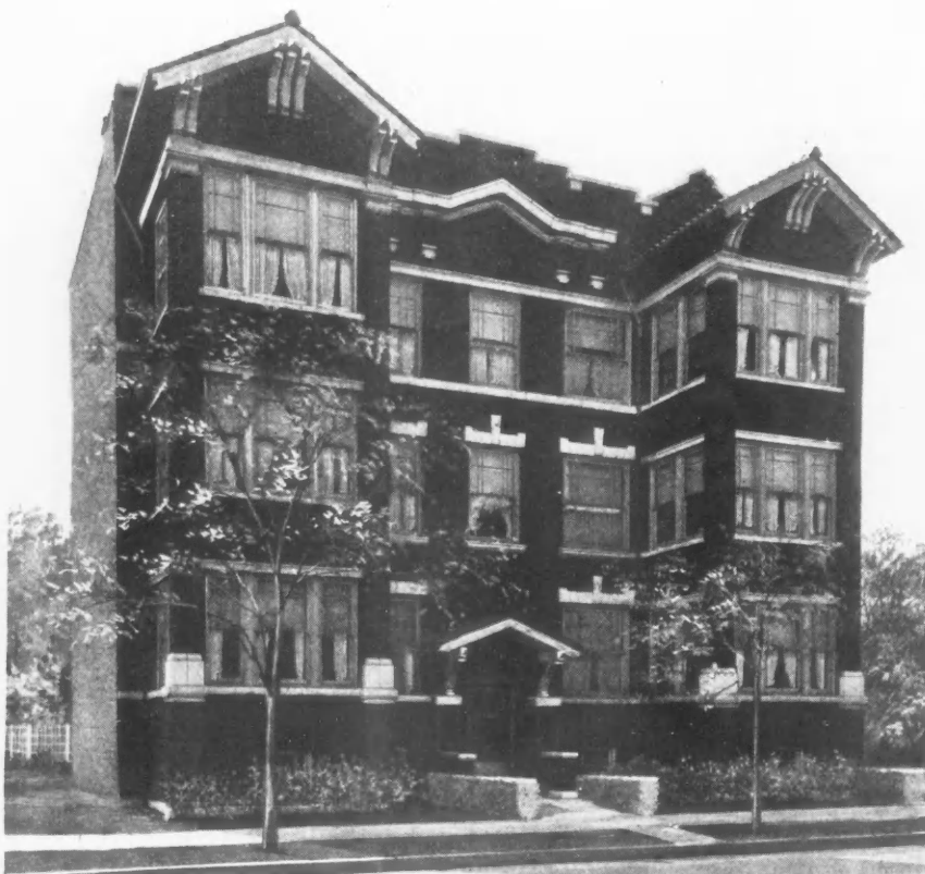
Six-Apartment Building of Brick Construction with Terra Cotta Trim. Each Apartment Has Five Rooms and Sun Parlor. The Building Is 50 Feet Wide and 64 Feet Long.
