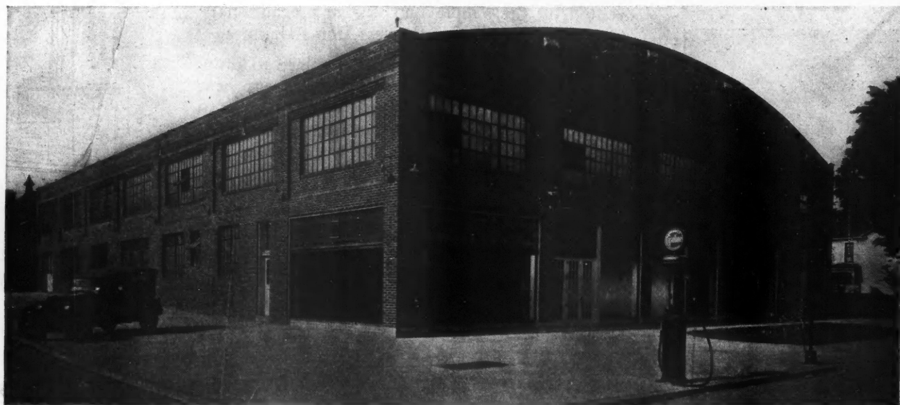
Type of Large Capacity Public Garage with Curving Trussed Roof. Very popular with builders, owners and the car-driving public.
