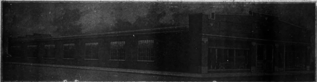
Exterior View of No. 2254 Garage
