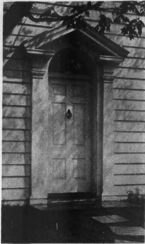
The Handsome Side Doorway Has Hand-wrought Latch, Hinge and Knocker Adapted from Similar Pieces Found in Old New England Houses.
