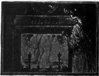
A slight contraction of the throat by turning the handle of the Peerless Dome Damper corrects this fault
