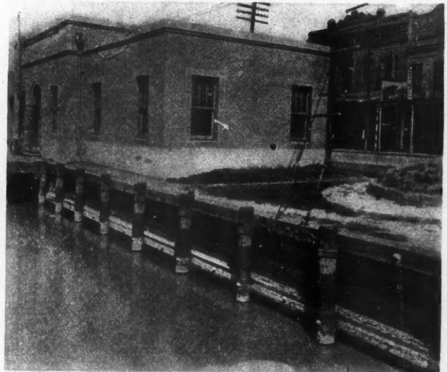
Treated Piling Necessary Here to Defeat the Ruthless Marine Borer.
